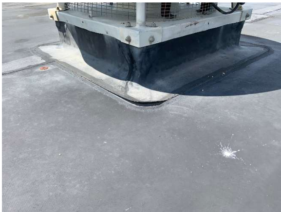
Failing Seam.
