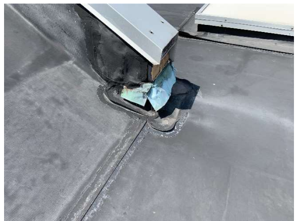
Damaged counter flashing.
