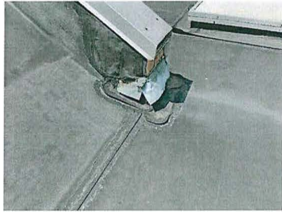
Damaged counter flashing.
