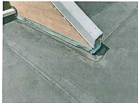
Damaged counter flashing.
