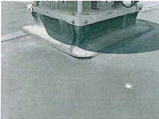
Failing Seam.
