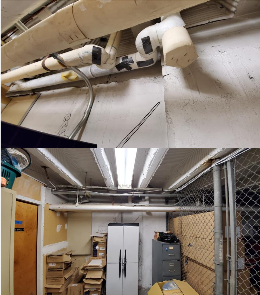
Picture 2.0-2.1: Shows positive ACM Pipe Insulation & ACM Mudded Joint Packing in the Storage Space of the Basement.
