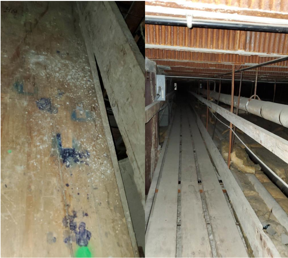
Picture 3.0-3.1: Shows positive ACM Pipe Insulation & ACM Mudded Joint Packing on the metal elbows and piping in the contaminated attic space. The attic space catwalk and fiberglass insulation are contaminated with ACM Pipe Insulation & ACM Mudded Joint Packing debris. Please refer to Table 1 to proper procedures regarding the abatement of the Attic Space.
