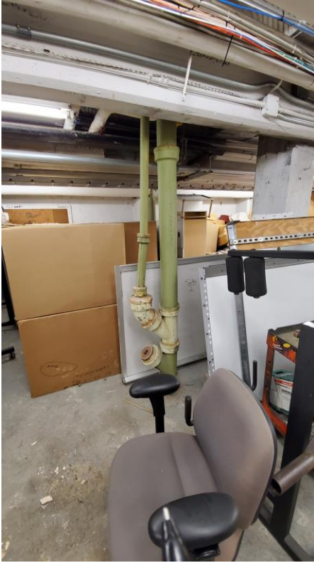
Picture 1.0: Positive Lead-Based Green Paint on the Sewer Pipes in the Storage Space of the Basement.
