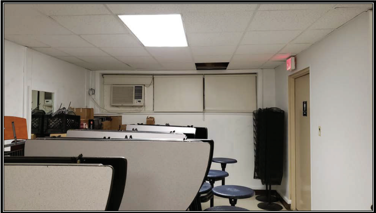
Photograph #1 – Existing installed Window Air Conditioning Unit in room 8 (identical to room 9)
