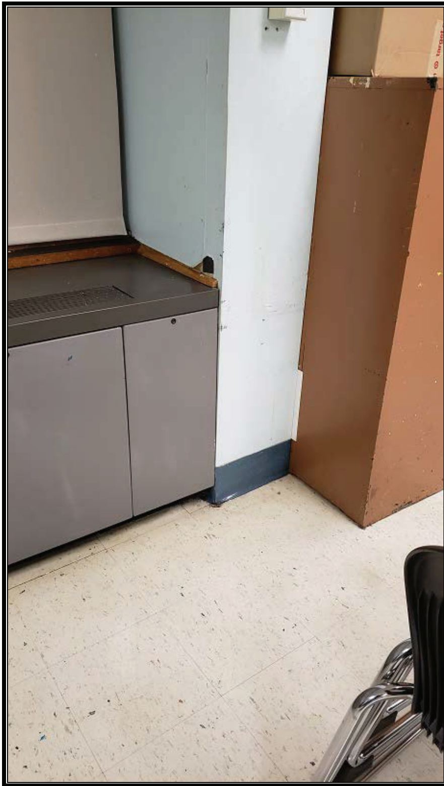
Photograph #1 – Typical Unit Ventilator installation associated with Non-ACM 12”x12” Beige with Blue Spots Floor Tile & Mastic, Non-ACM Blue 6” Cove Base & Mastic, Non-ACM Gypsum, Asbestos Containing Joint Compound and Non-ACM Wall Paper over Gypsum.
