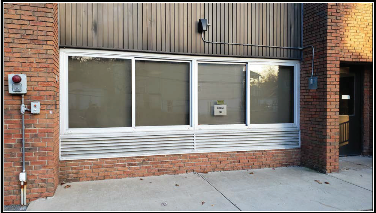
Photograph #2 – Typical Unit Ventilator Exterior Louver layout associated with Non-ACM Exterior Brick Mortar and Asbestos Containing Exterior Louver Caulking
