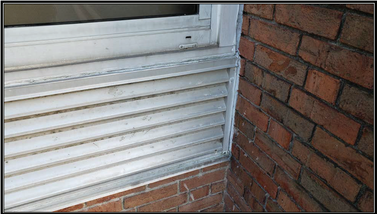
Photograph #3 – Asbestos Containing Exterior Louver Caulking (also associated with exterior window frames)
