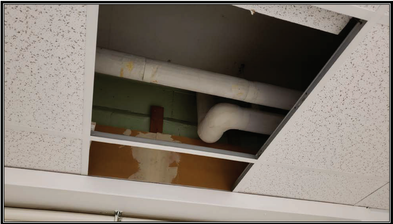
Photograph #2 – Non-ACM Gypsum, Asbestos Containing Joint Compound, Non-ACM 2x2 Ceiling Tile, Non-ACM CMU Mortar, Asbestos Containing Pipe Insulation, Asbestos Containing Pipe Fittings and Non-Suspect Concrete Ceiling Deck.
