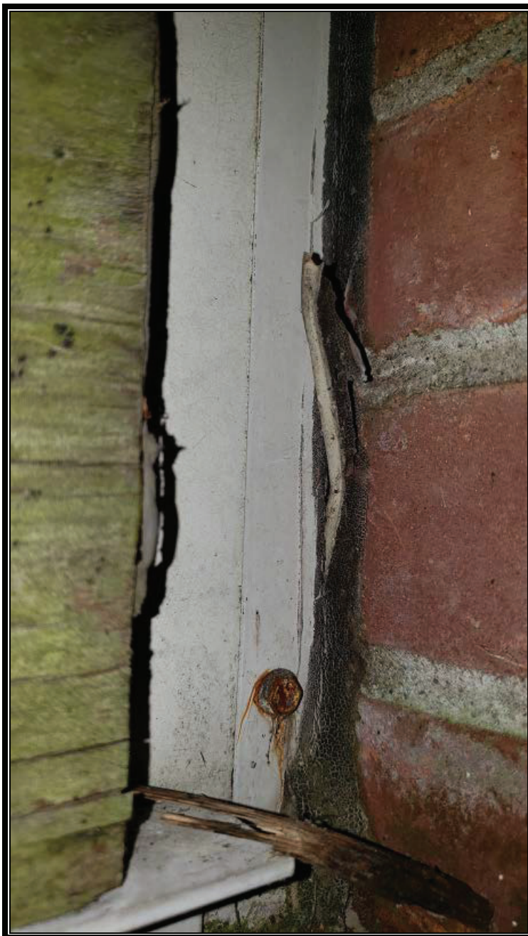
Photograph #4 – Non-ACM Exterior Brick Mortar and Non-ACM Exterior Window Frame Caulking
