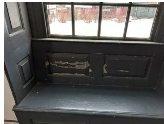
WOODWORK - COMPLETELY RESTORE TO SOUND CONDITION AND ORIGINAL PLANES AND PROFILES. REPLACEMENT COMPONENTS MUST REPLICATE THE SIZE, SHAPE AND PROFILE OF THE ORIGINAL. MATCH HISTORIC JOINERY DETAILS SUCH AS MORTISE AND TENON JOINTS.
