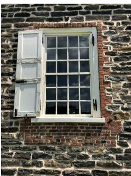
DAMAGED & MISSING SHUTTER
