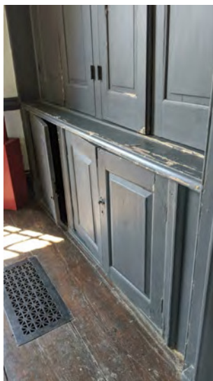
WOODWORK - COMPLETELY RESTORE TO SOUND CONDITION AND ORIGINAL PLANES AND PROFILES. REPLACEMENT COMPONENTS MUST REPLICATE THE SIZE, SHAPE AND PROFILE OF THE ORIGINAL. MATCH HISTORIC JOINERY DETAILS SUCH AS MORTISE AND TENON JOINTS.
