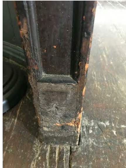
NEWEL POST DAMAGE TYPICAL FOR "STAINED & VARNISHED" WOODWORK. SHALL BE FILLED, STAINED AND VARNISHED.
