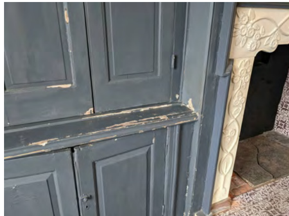
WOODWORK - COMPLETELY RESTORE TO SOUND CONDITION AND ORIGINAL PLANES AND PROFILES. REPLACEMENT COMPONENTS MUST REPLICATE THE SIZE, SHAPE AND PROFILE OF THE ORIGINAL. MATCH HISTORIC JOINERY DETAILS SUCH AS MORTISE AND TENON JOINTS.
