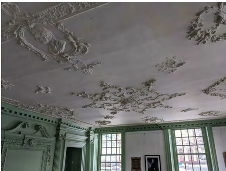
ROOM 103 - PAPER MACHE CEILING NOT TO BE DISTURBED. CONTRACTOR SHALL TAKE MEASURES TO PROTECT DURING CONSTRUCTION
