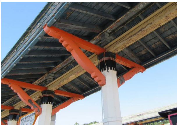
EXAMPLE OF BEAM AND BRACKET PLAYLAND BUS TERMINAL CANOPY FOR INFORMATION ONLY
