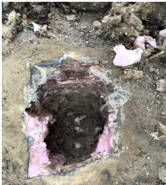
PHOTO 24: Built Up Roofing Composite (HA-24-L1/L2/L3/L4) – Roof at Northeast Corner (High Point)
