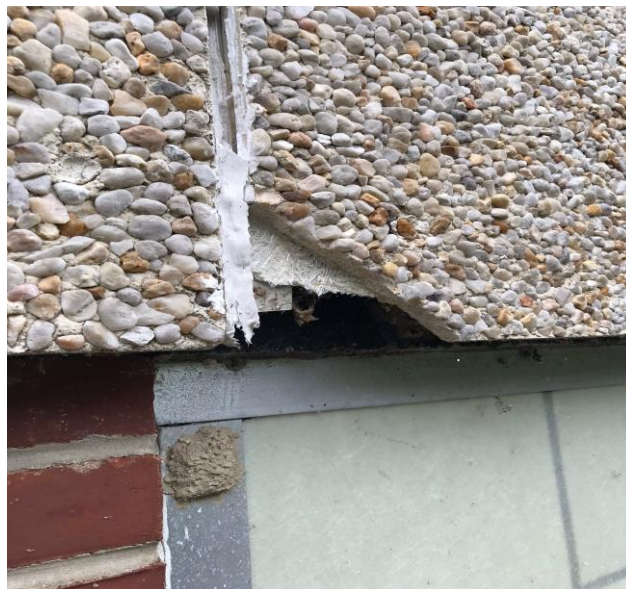
PHOTO 20: Caulk (white) to Decorative Cementitious Paneling (HA-20) – Exterior South Elevation
