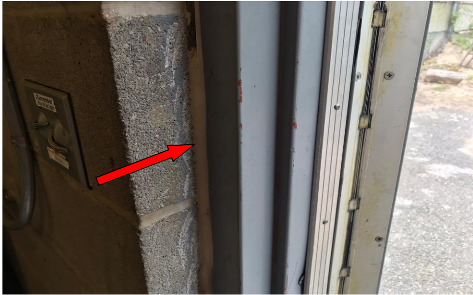
PHOTO 1: Interior (white) Door Frame Caulk (HA-01) – Main Level at Entry Door
