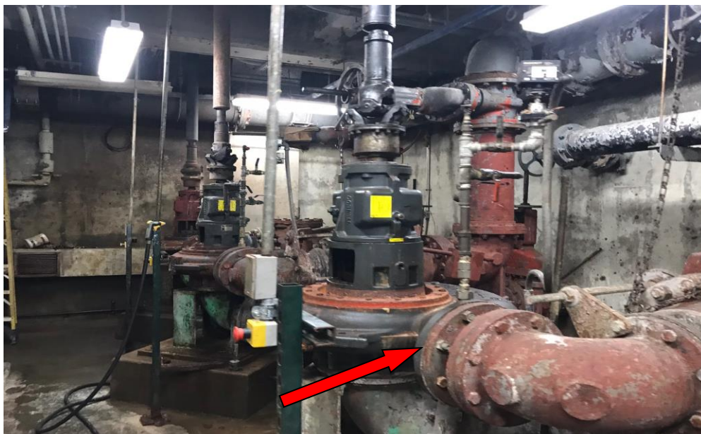
PHOTO 18: Flange Gasket (HA-18) – Lower Level Blower Unit Plumbing
