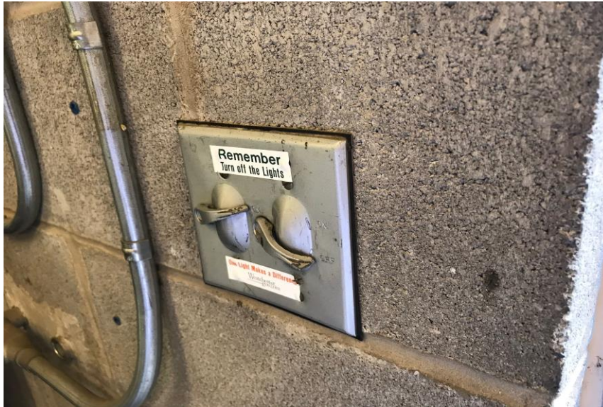
PHOTO 13: Fibrous Wall Receptacle Backing (HA-13) – Main Level Main Area Adjacent to Entry
