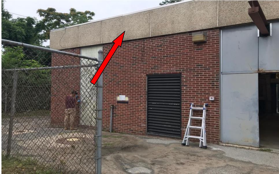
PHOTO 21: Cementitious Panels (with Decorative Aggregate) (HA-21) – Exterior South Elevation
