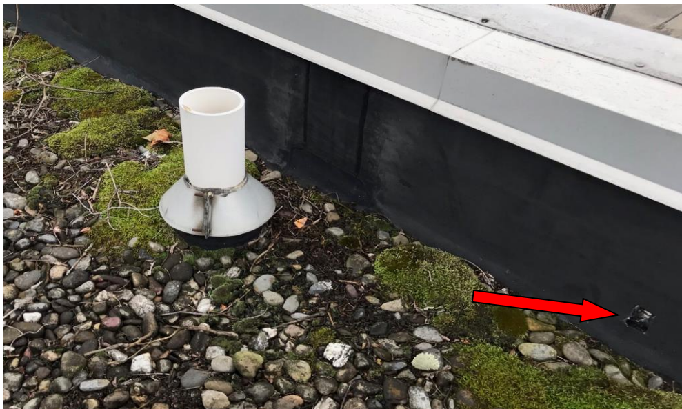
PHOTO 22: Tar to Parapet Wall and Base Flashing Roofing Membrane (HA-22-L1/L2) – Roof Perimeter
