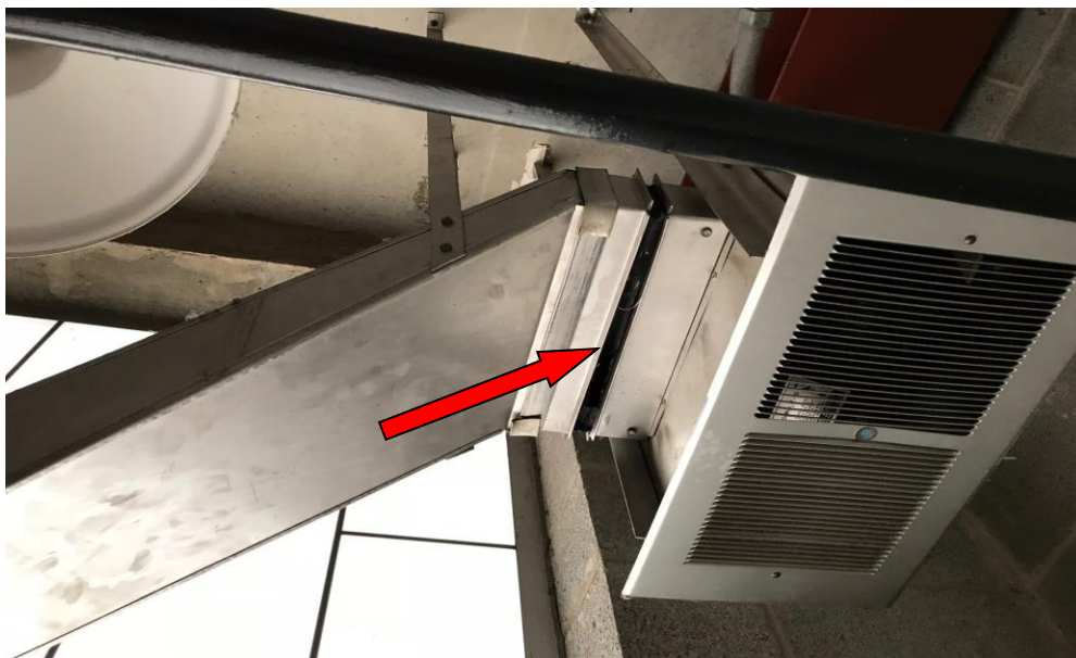
PHOTO 14: (black) Duct Vibration Cloth (HA-14) – Main Level Bathroom Diffuser Dampner
