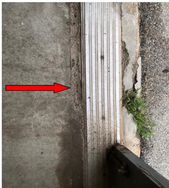
PHOTO 2: Leveling Compound (HA-02) – Main Level Entry Door Threshold
