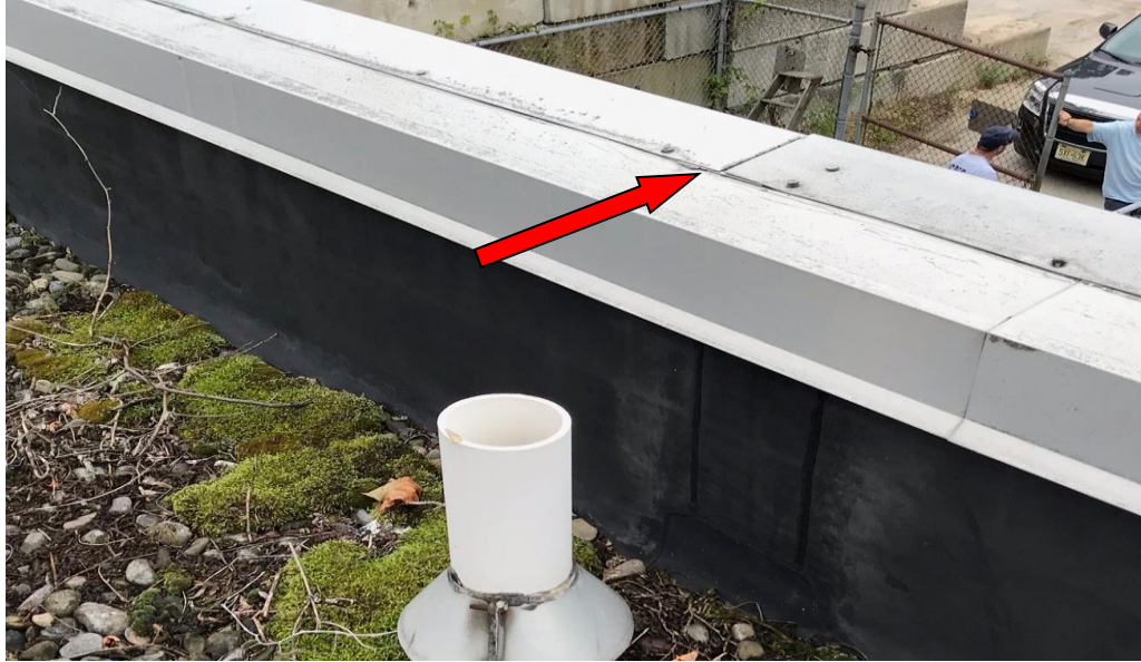
PHOTO 25: Caulking (grey) to Metal Cap Flashing (HA-25) – Roof at East Corner
