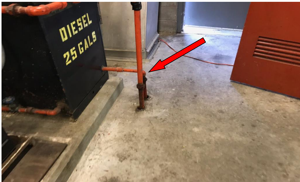
PHOTO 6: Pipe Dope to Diesel Fuel Line (HA-06) – Main Level Main Area to Generator Fuel Cell
