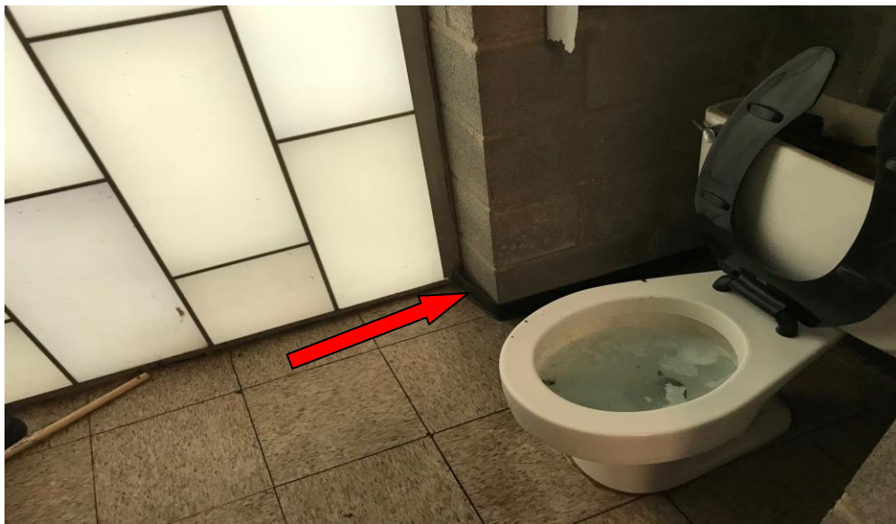
PHOTO 12: (black) 2.5" Vinyl Cove Base and Associated Glue (HA-12/12G) – Main Level Restroom
