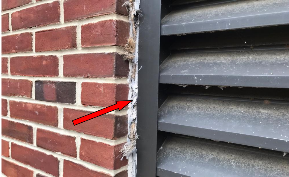
PHOTO 19: Backer Rod (fibrous) (HA-19) – Exterior East Elevation Louver
