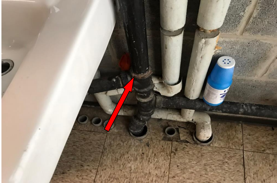
PHOTO 5: Pipe Dope to Drain Pipe (HA-05) – Main Level Restroom
