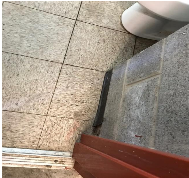
PHOTO 10: 12" x 12" (beige) Vinyl Floor Tile and Associated Mastic (HA-10/10M) – Main Level Restroom
