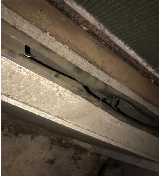
PHOTO 7: (black) Duct Vibration Cloth (HA-07) – Main Level Generator Intake Ductwork Dampener
