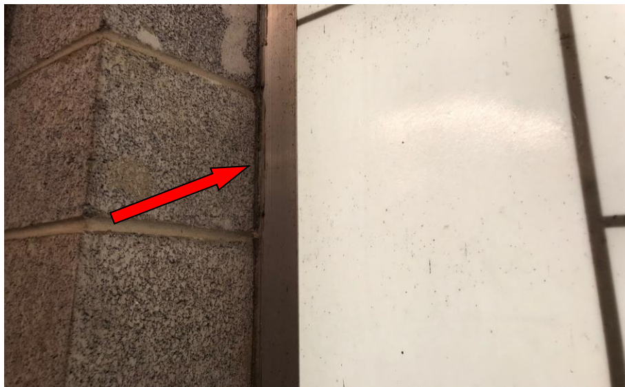
PHOTO 4: Interior (grey) Window Frame Caulk (HA-04) – Main Level at Northeast Window Unit
