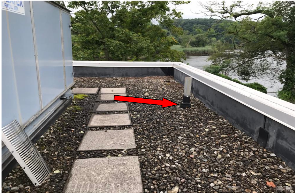
PHOTO 23: Vent Stack Pitch Pocket (HA-23) – Roof Area at North End
