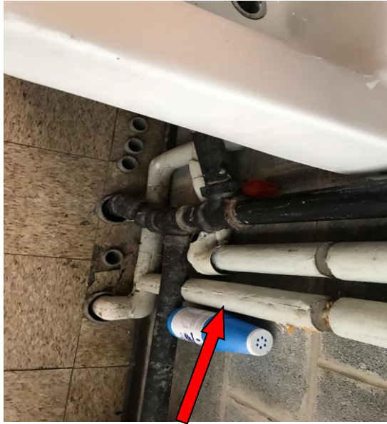
PHOTO 11: All Service Jacket to Fiberglass Insulated Ring (HA-11) – Main Level Restroom Domestic Cold Water Line Beneath Sink
