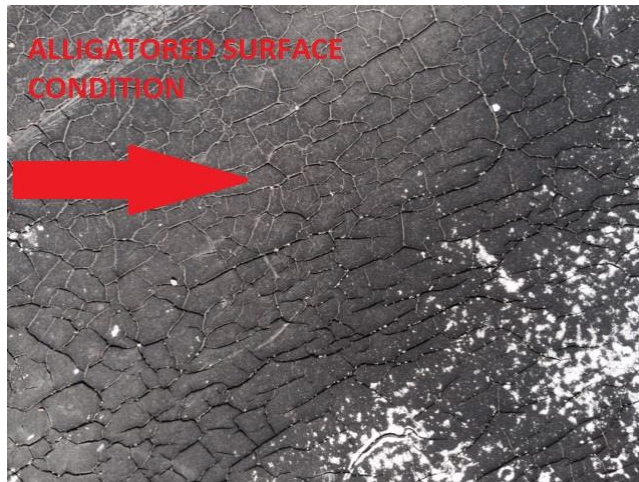
Photo exhibits alligatoring surface condition.
