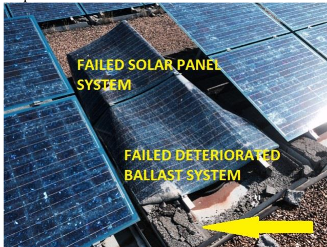
Photo exhibits failed solar panel system and ballast that is no longer secured and at risk of a blow off resulting in injury below.
