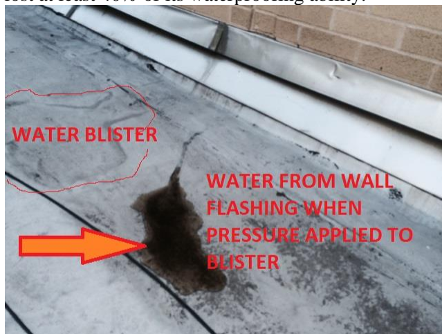
Photo exhibits surface blister condition.
