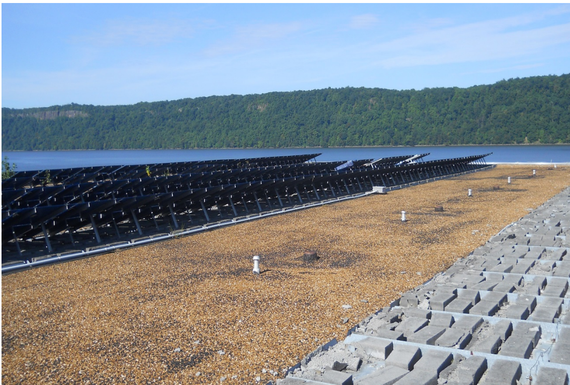
Photo #6: Thickening Building – Typical view of the built-up roofing. The field roofing materials were found to be non-ACM, however, the flashing material around the perimeter of the roof is ACM.
