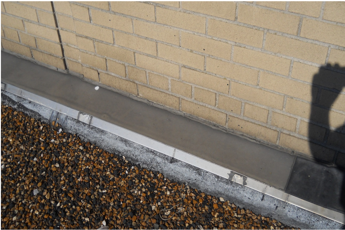
Photo #5: Administration Building - View of the dark grey caulk along the top of the metal counterflashing. This caulk does not contain asbestos or PCBs.
