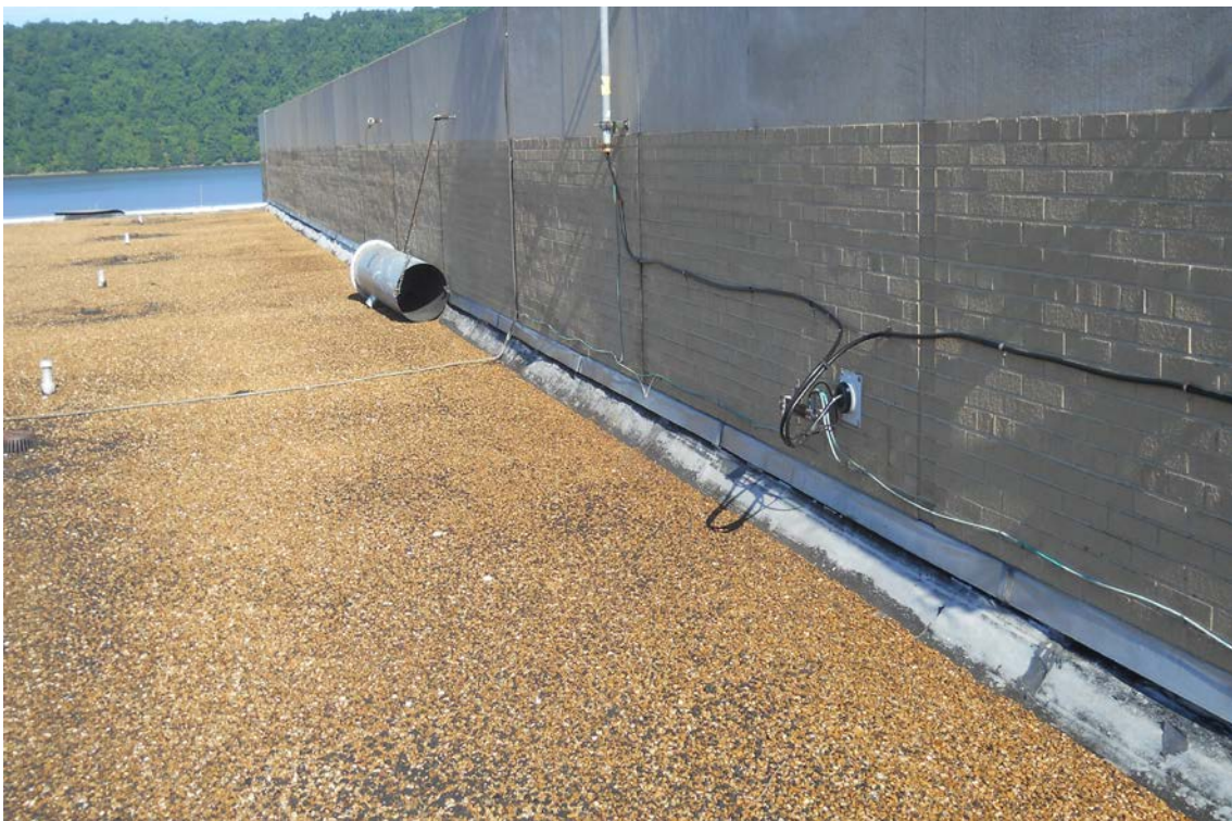
Photo #2: Blower Building - View of the asbestos-containing flashing top mastic (1200 SF) on top of the perimeter flashing. The flashing top mastic is non-friable and fair condition. The perimeter flashing is also asbestos-containing and is non-friable and in fair condition.
