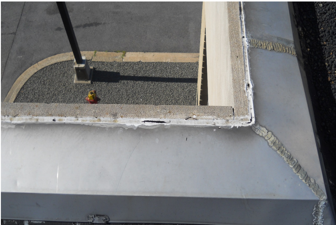
Photo #4: Blower Building - View of the white caulk along the coping on the parapet around the perimeter of the roof. This caulk does not contain asbestos or PCBs.
