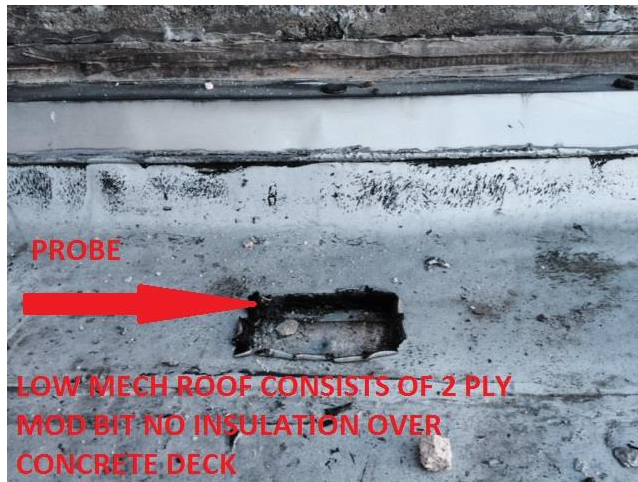
Probe of lower mechanical roof reveal a smooth 2 ply modified bitumen roof system containing no insulation and tapered concrete.
