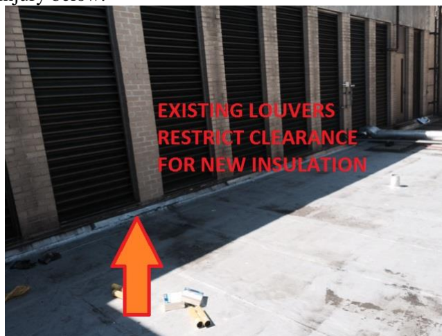
Photo exhibits wall louvers of lower mechanical roof are restricting flashing height for building code insulation requirement.
