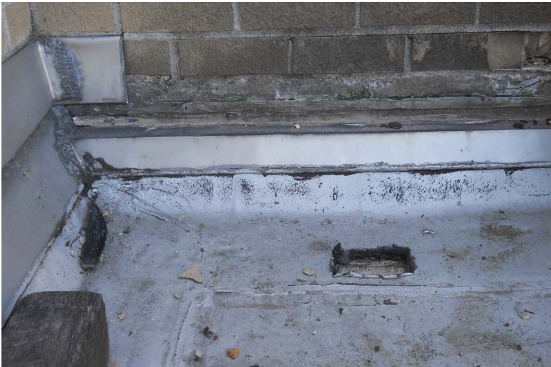
Photo #1: Administration Building - View of the asbestos-containing bottom layer membrane (3025 SF) located on the lower roof. The membrane is non-friable and in good condition.
