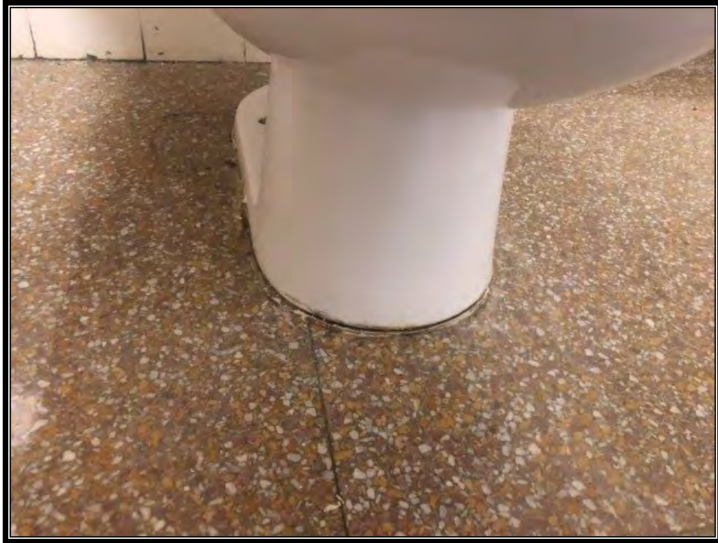
Photo 5: Non-ACM Fixture Caulking (White)
