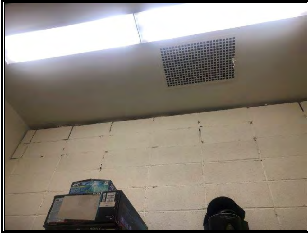
Photo 1: Non-ACM Interior CMU Mortar (Grey)
