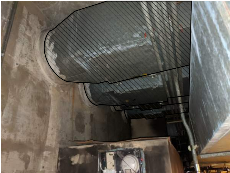
FIGURE 3: MER ROOM DUCT CONNECTION TO UNDERGROUND TRANSITE DUCTS
