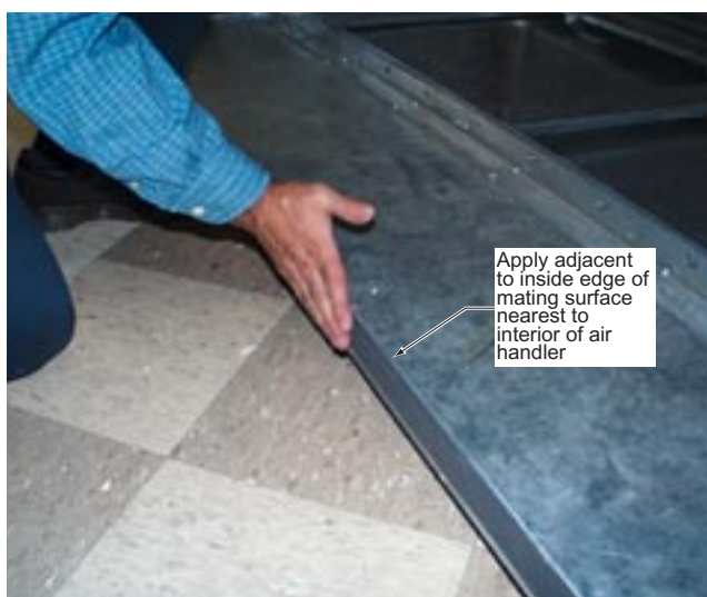
FIG. 2-17 – APPLYING GASKET
