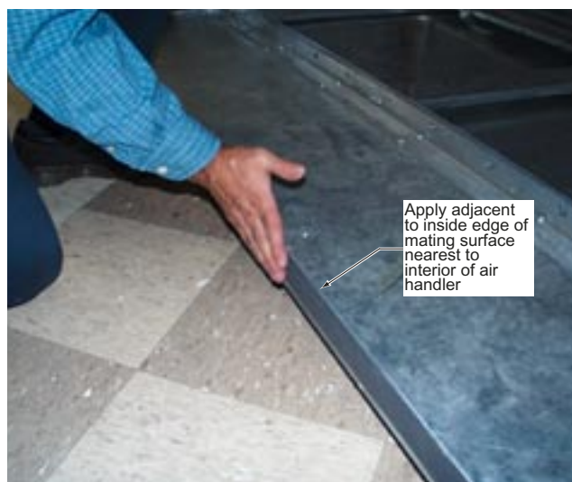
FIG. 2-9 – APPLYING GASKET
