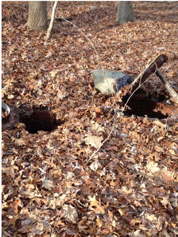
Septic tank and well pit
