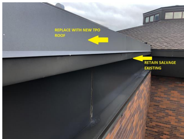
Above existing fascia should be able to be retained, existing roof metal edge to be replaced with new TPO roof system.
