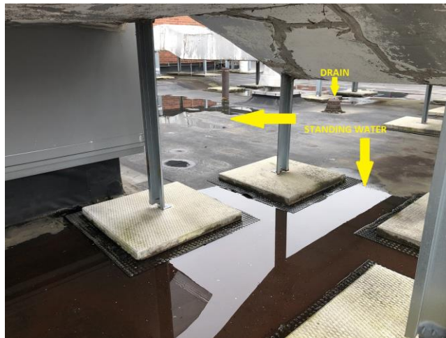
Above and below photos exhibit the standing ponding water condition throughout fields.
