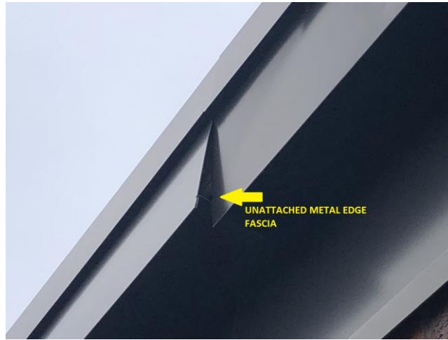
Photo exhibits unattached metal edge fascia.
