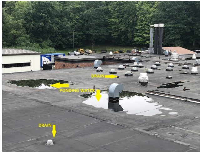
Above and below photos exhibit the standing ponding water condition throughout fields.
