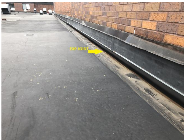
Above and below photos exhibit a high volume of perimeter bulkhead consists of an expansion joint detail.
