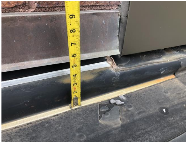
Above and below photos exhibit a high volume of perimeter bulkhead consists of an expansion joint detail.
