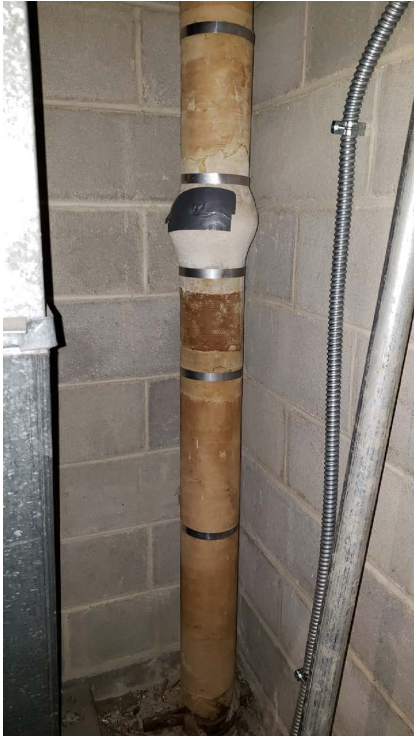
Asbestos containing Elbows to Fiberglass Pipe Insulation with Tar Containing Wrap, Gray
