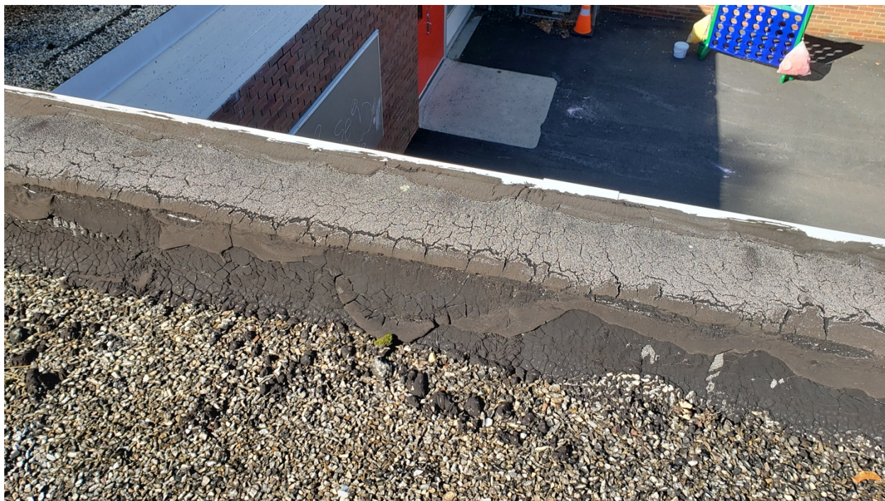
Non-Asbestos Containing Tar on Curbs/Eaves Flashing
