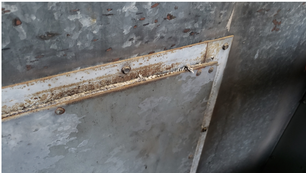
Asbestos containing Rope Insulation to Duct Hatch, White
