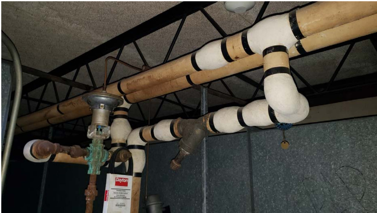
Asbestos containing Elbows to Fiberglass Pipe Insulation with Canvas Wrap, Gray
