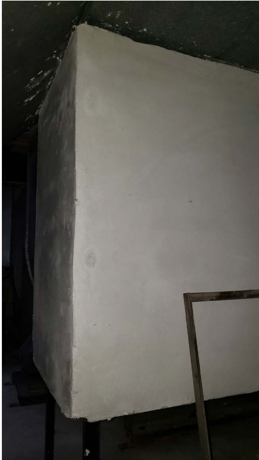
Asbestos containing Duct Insulation, Gray
