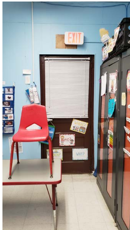
Asbestos containing 9"x9" Floor Tiles, Red & Mastic underneath non-asbestos containing 12"x12" Floor Tile, White & Mastic.
