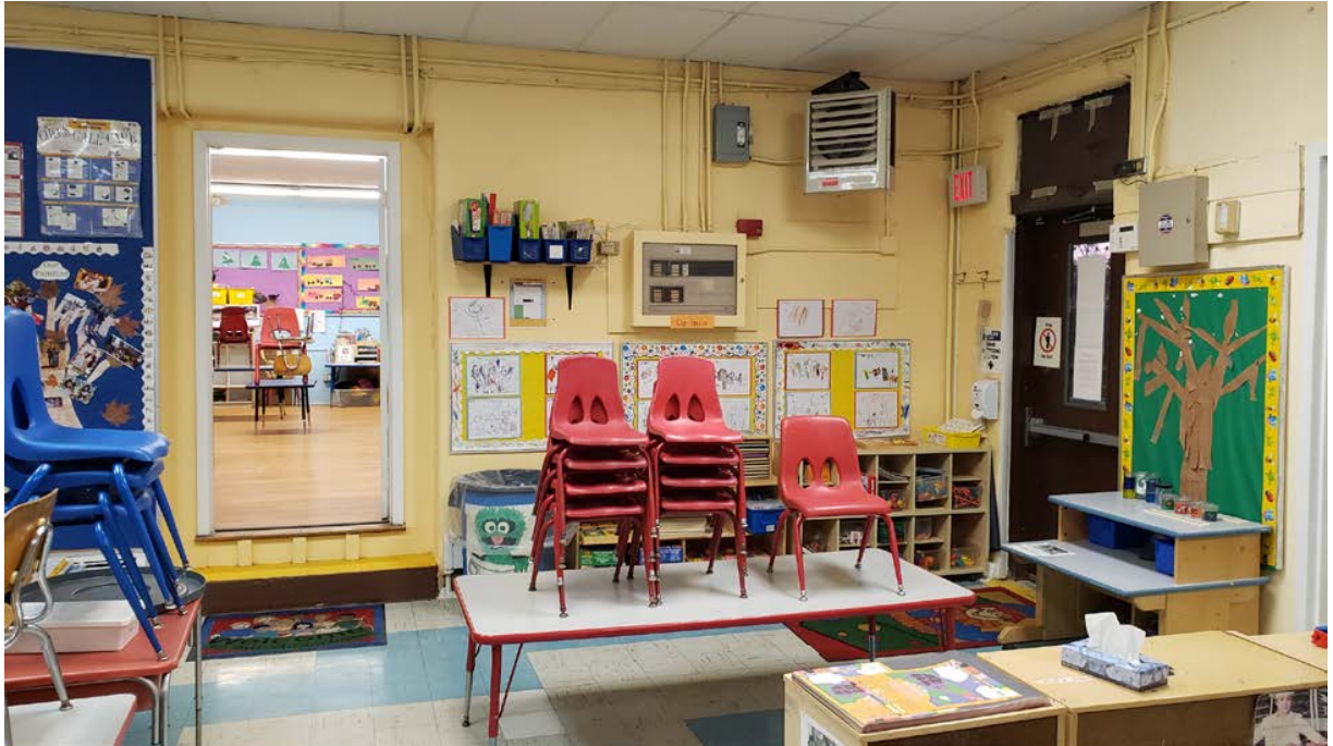
Asbestos containing 9"x9" Blue & White Floor Tiles and Mastic
