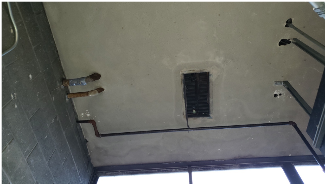
Asbestos containing Elbows to Original Fiberglass Pipe Insulation, White
