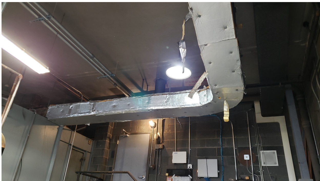
Asbestos containing Mastic to Fiberglass Duct Insulation Clamps, Brown
