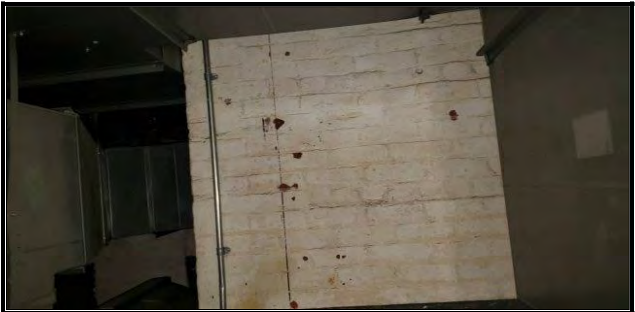
Photo 4: Non-ACM Chimney Brick Mortar (Gray) -Gym Building
