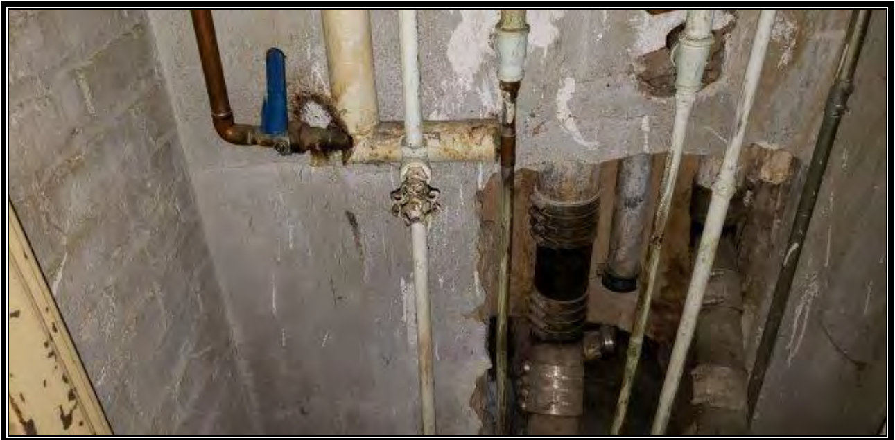
Photo 22: Fiberglass Pipe Insulation and Metal Pipes
