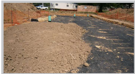
Fig. 20 Pushing backfill parallel to the Geogrid prevents the grid from shoving.
