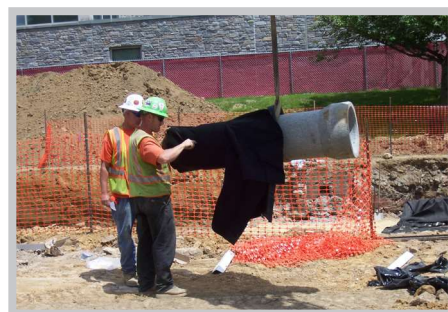
Fig. 16 Install boots onto pipes prior to connecting them to the R-Tank, leaving the clamps loose for final adjustment later
