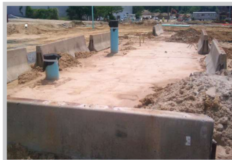
Fig. 22 Secured R-Tank® installation using Jersey barriers
