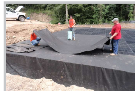
Fig. 13 Encapsulate R-Tanks® with geotextile
