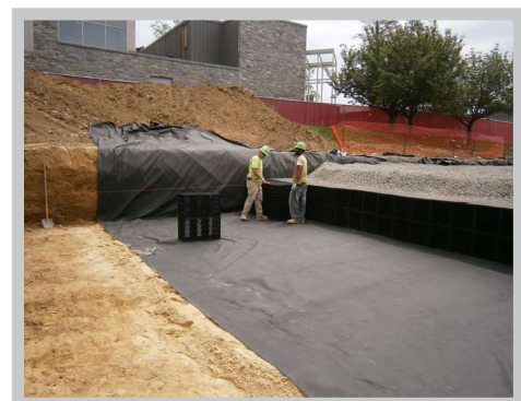
Fig. 3 Pull wrinkles out of geotextiles so material lays flat
