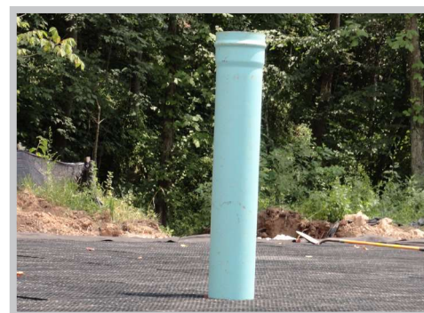
Fig. 10 Installed maintenance port
