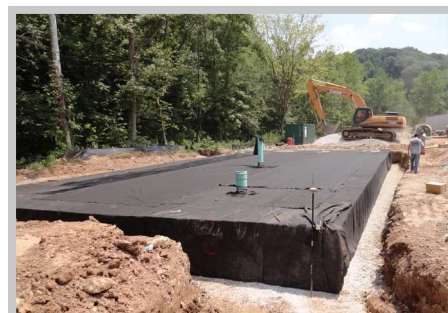
Fig. 15 Finished envelope should lay flat against R-Tank®
