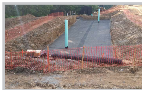
Fig. 21 Secure the installation with temporary fencing
