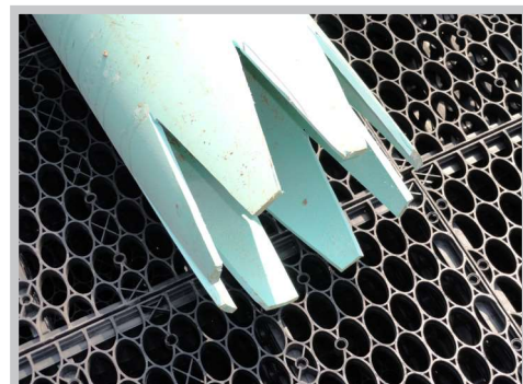
Fig. 9 Cut 8" notches into the bottom of maintenance port
