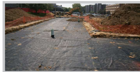
Fig. 19 Overlap geogrid 18" or as required by plans.
