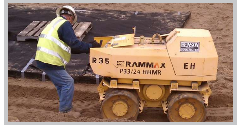
Fig. 17 Vibratory compaction of side backfill is ALWAYS REQUIRED, regardless of what backfill material is used.
