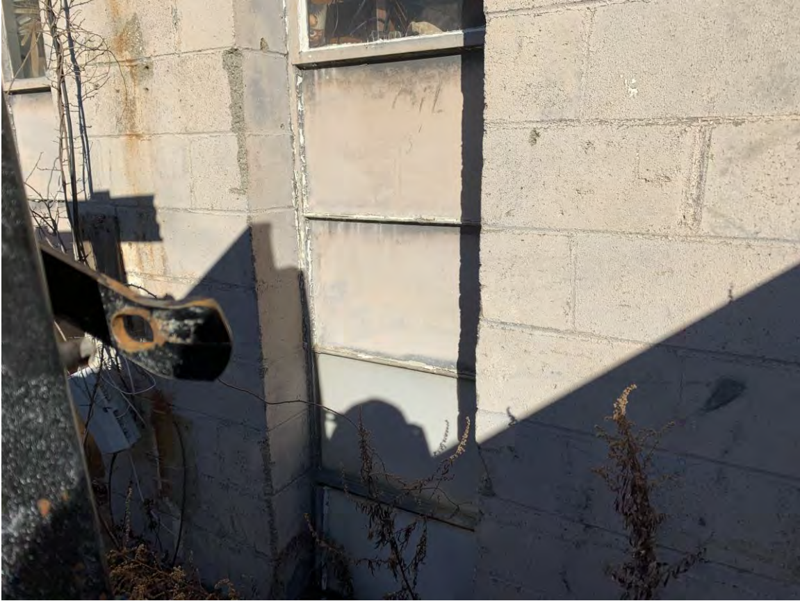
ACM Window Glazing & Transite Panels
