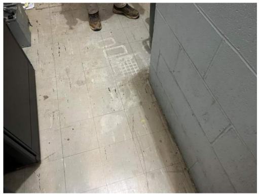
Above: Server Room 22C ACM 9"x9" Floor Tile & Mastic Below: Fan Room ACM Pipe Insulation & Mudded Joint Packing/Fittings/Elbows/Etc.
