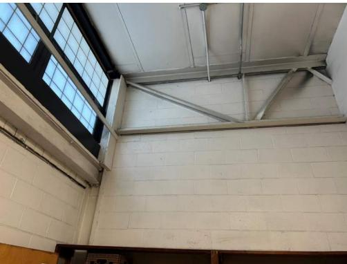
Above: Example of White Beams Positive for Lead Below: Example of Red Beams Positive for Lead
