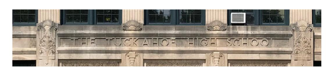
CLEAN EXIST CAST STONE ELEMENT, INCLUDING FRIEZE PANELS, BAS RELIEF CARVINGS, BANDING, SCHOOL NAME ELEMENT PANELS, & COLUMNS. CONTRACTOR SHALL ENSURE ALL JOINTS ARE PROPERLY SEALED SHOULD MORTAR OR SEALANT BE DISPLACED DURING **CLEANING - SEE SPECS FOR CLEANING** INSTRUCTIONS - TYP.
