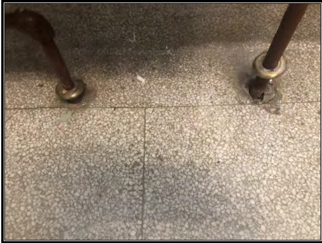
Photo 3: Non-ACM Firestop at Radiator Penetration (Tan)
