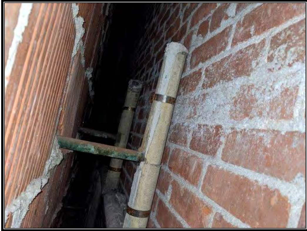
Photo 9: ACM Pipe Insulation (Grey)
