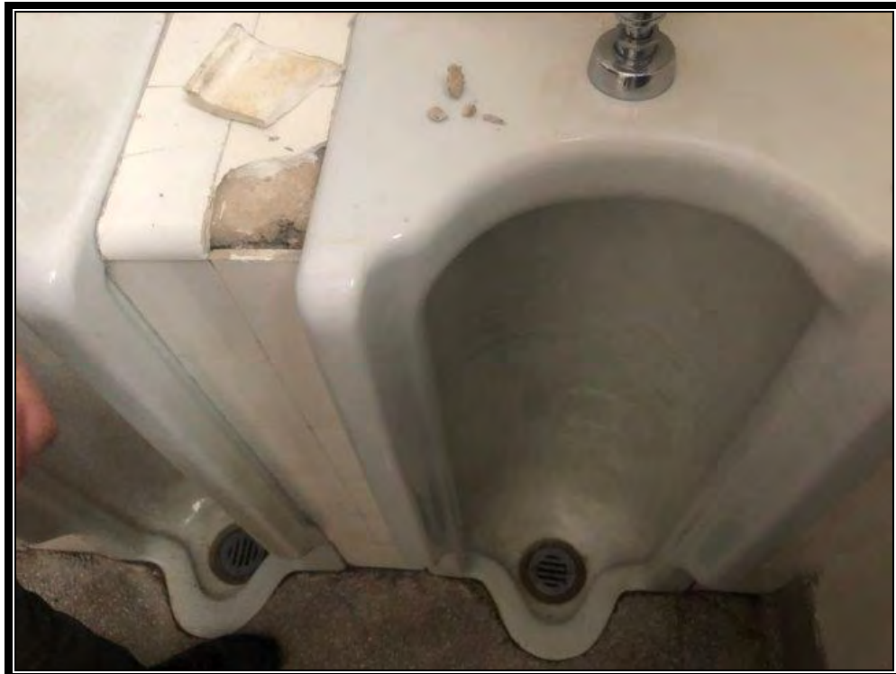
Photo 8: Non-ACM Grout to Ceramic Tile at Urinal (White) and Backing to Ceramic Tile at Urinal (White)
