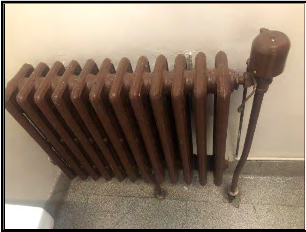
Photo 2: Non-ACM Textured Paint to Radiator (Brown)
