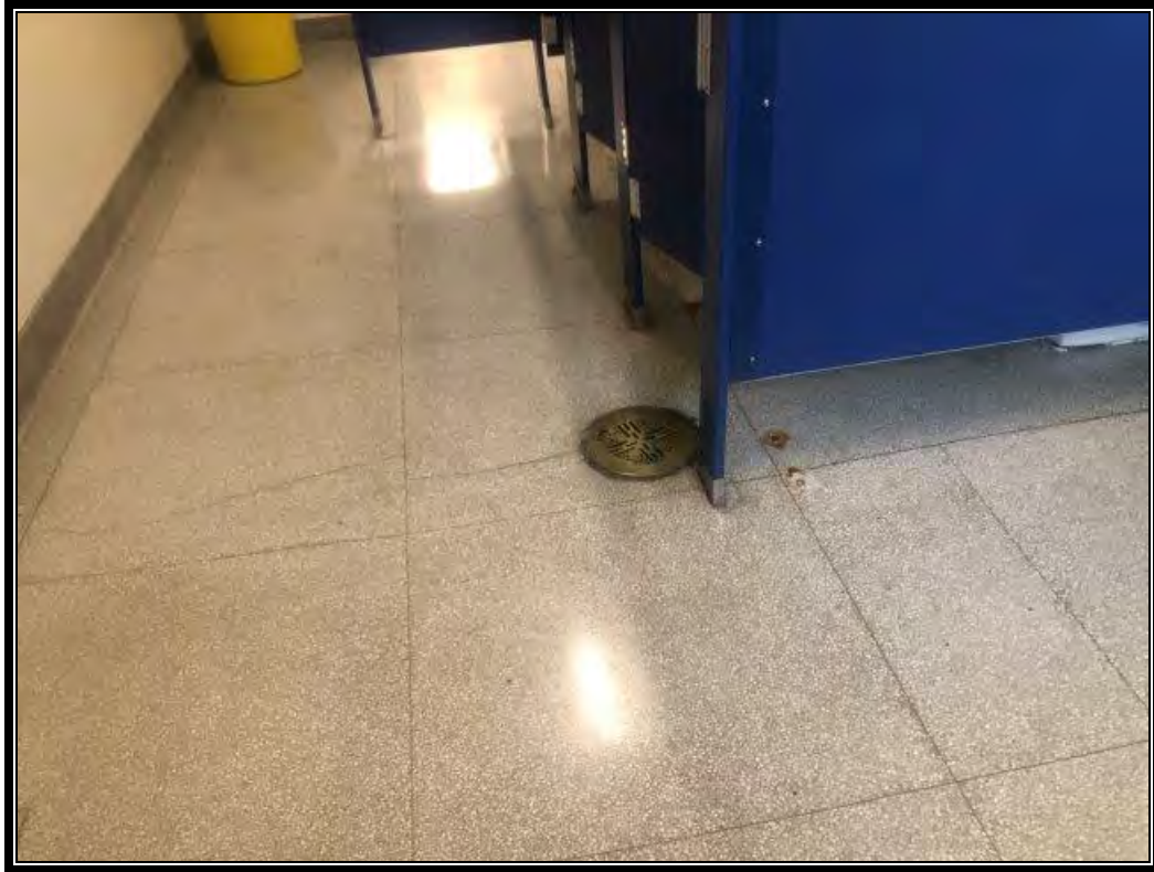
Photo 1: Non-ACM Sealant to Drain (Grey)
