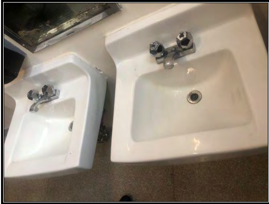
Photo 5: Non-ACM Fixture Caulk (White)
