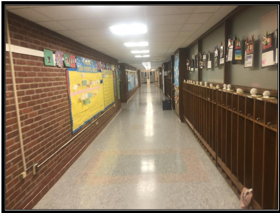
Photo 6: Non-ACM Brick Mortar and 12x12 Floor Tile
