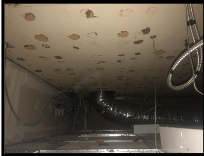
Photo 3: Non ACM Glue Dots on Ceiling
