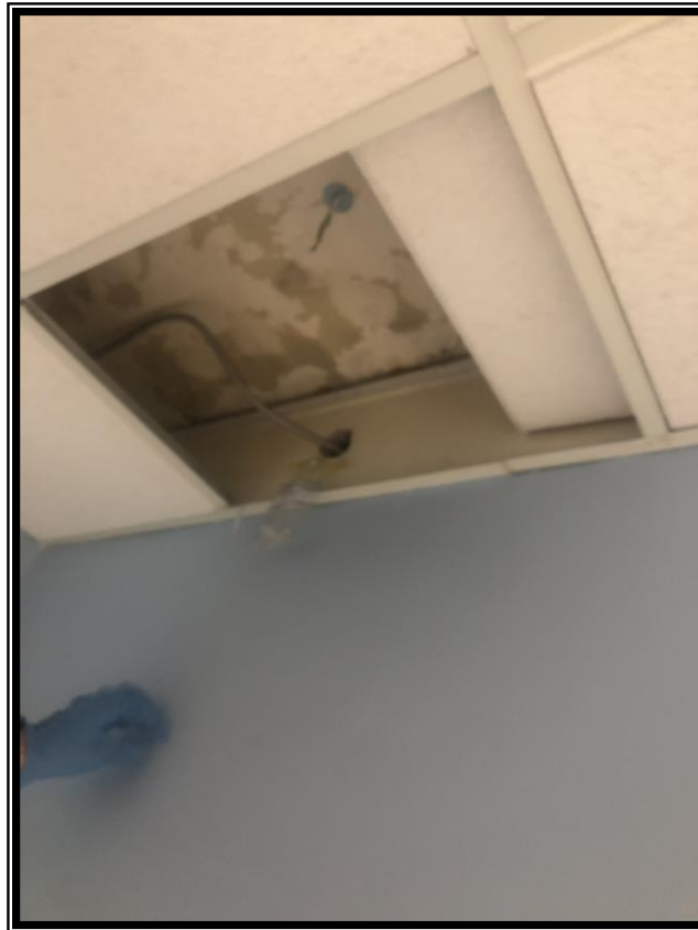
Photo 4: Non-ACM Plaster Wall and Ceiling. Also Showed Non ACM Ceiling Tiles 2'x2'
