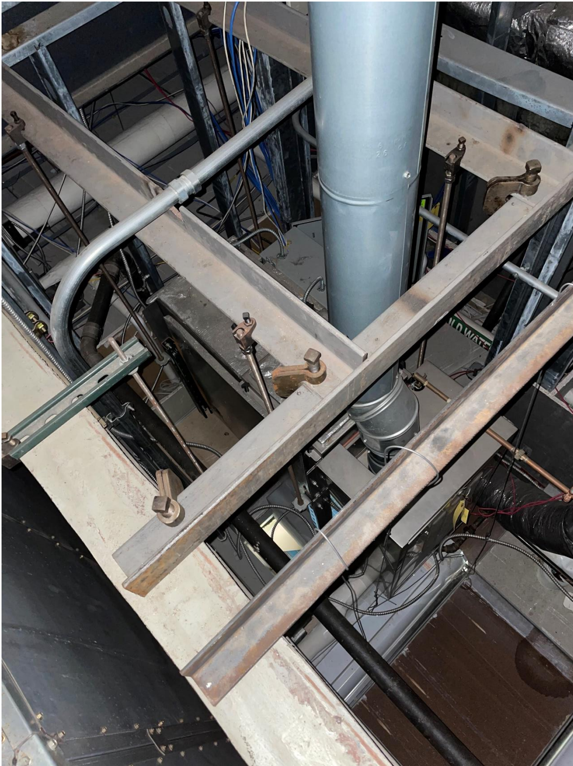
Image 6 – Existing Humidifier Above Toilet Rooms to be Removed
