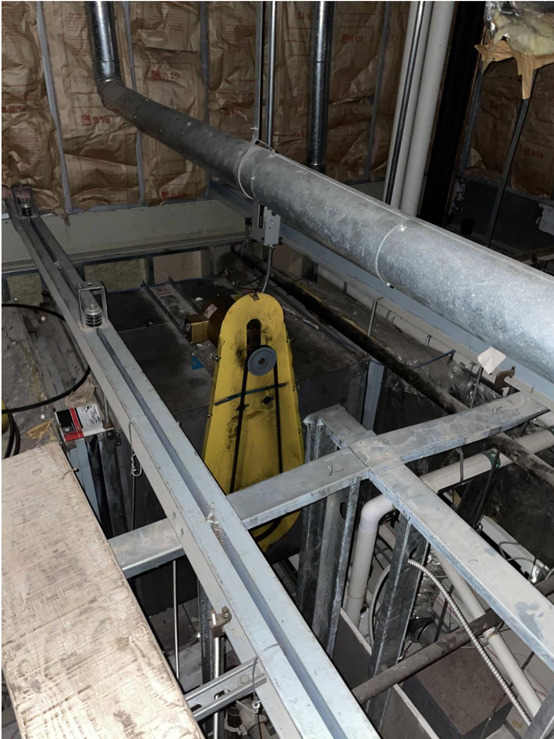
Image 7 – Existing Humidifier Above Toilet Rooms to be Removed
