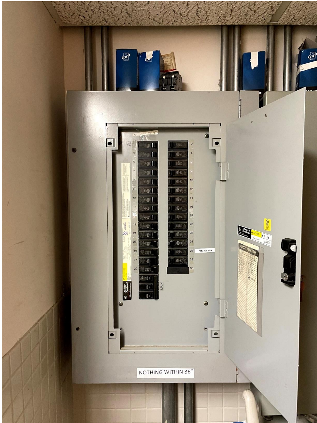
Image 1 – Existing Lighting Panel L-1
