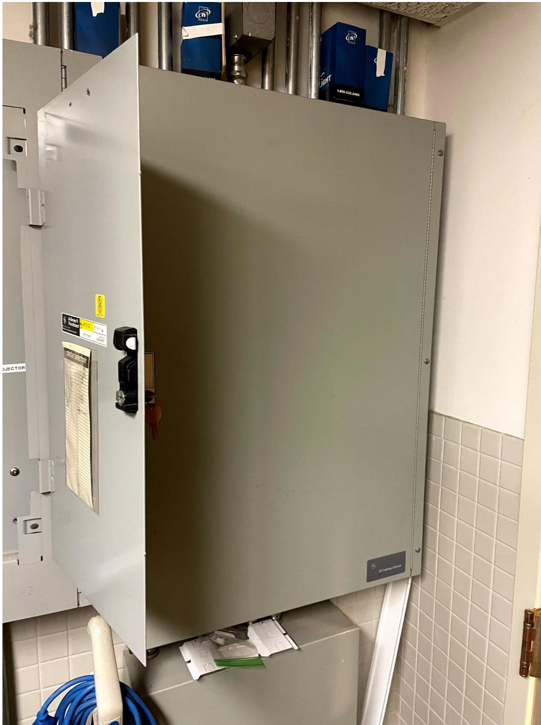
Image 3 – Existing Lighting Control Panel
