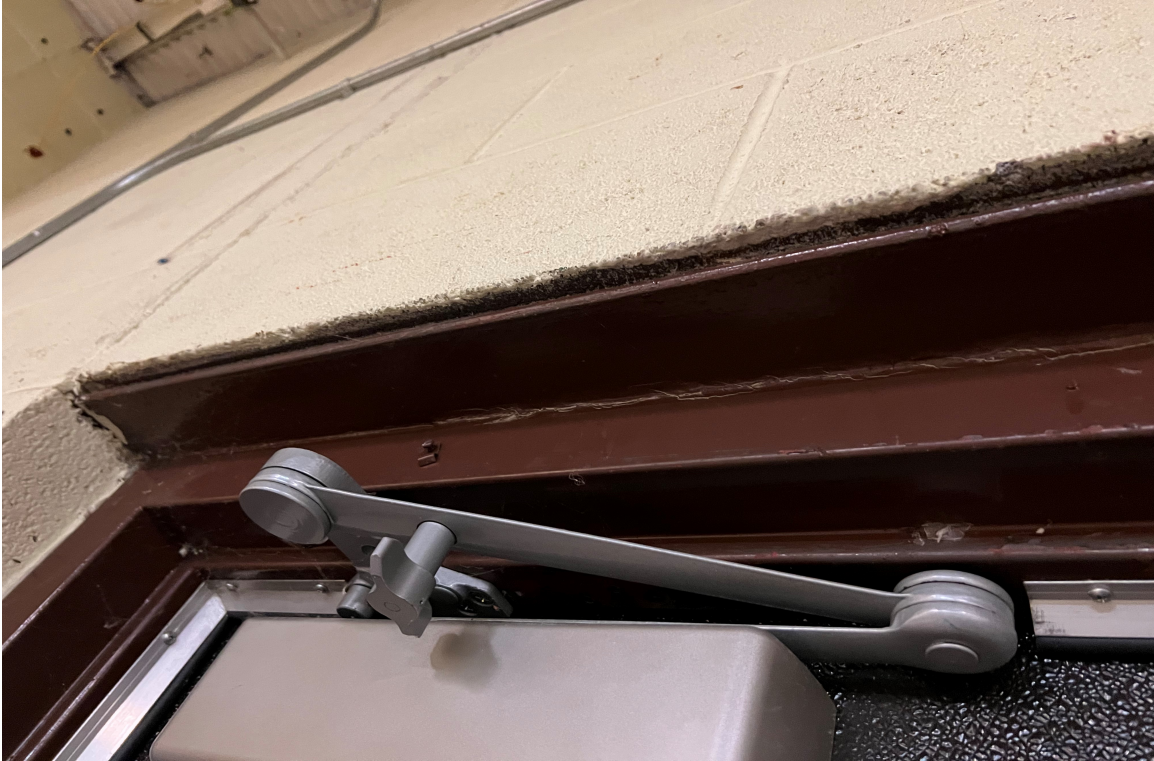
ABOVE: WEIGHT ROOM STORAGE – LBP EXTERIOR DOOR LINTEL
