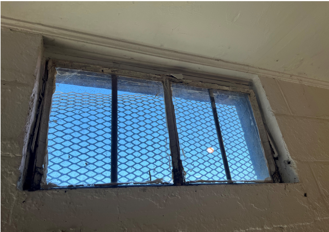
ABOVE: FIELD HOUSE – ACM CEMENTITIOUS PANELS BELOW: FIELD HOUSE – ACM WINDOW GLAZING
