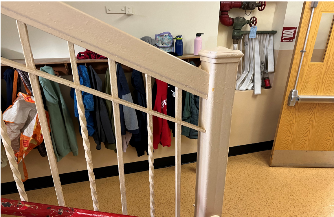
ABOVE: LBP WALL PLASTER & DOORWAY WINDOW FRAME BELOW: LBP STAIR RAILING
