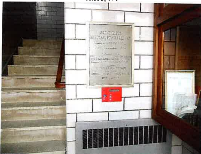
Space Identification # 1001 - assay # 1 - Grey Ceramic Wall Tile (Lead Based Glazing)
