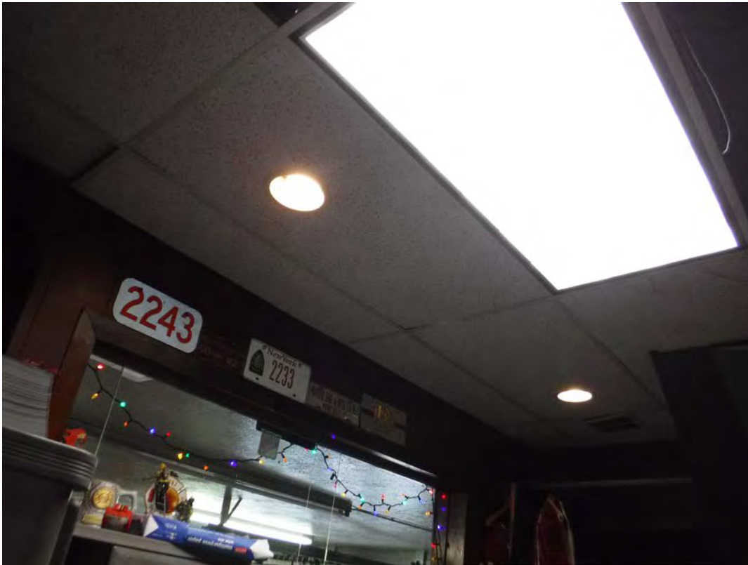
Interior, captain's office- non-asbestos containing 2'x4' ceiling tile
