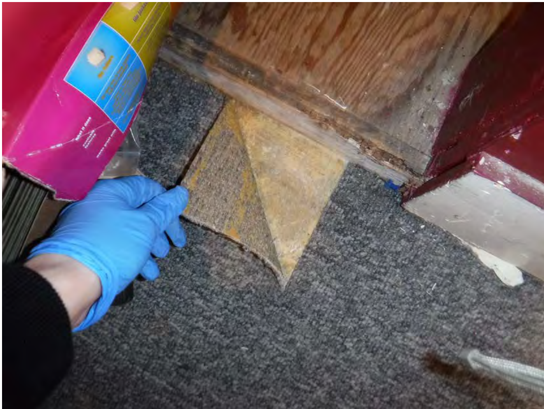
Interior, captain's office- non-asbestos containing carpet mastic
