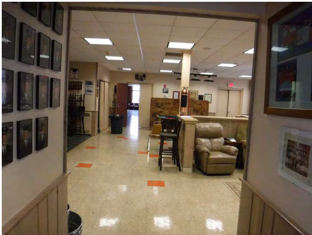
Interior, 2 nd floor- asbestos containing floor tile
