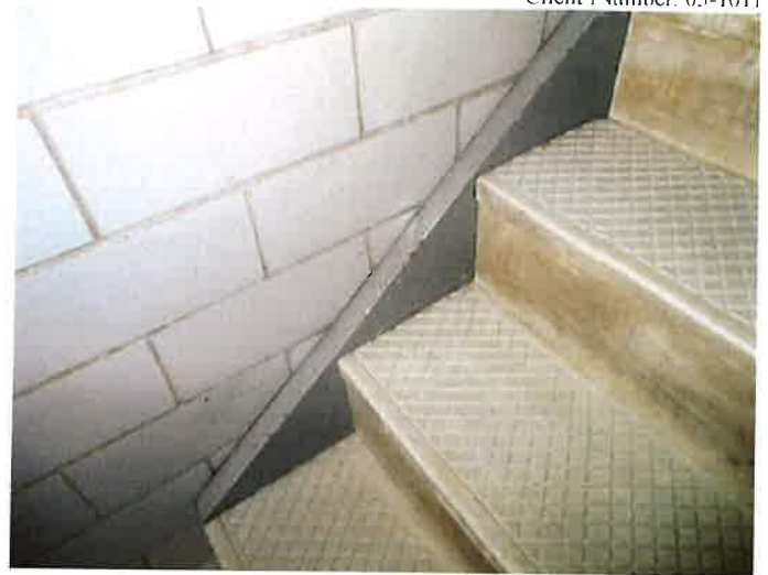
Space Identification # 1001 – assay # 7 - Staircase Stringer (Lead Based Paint)
