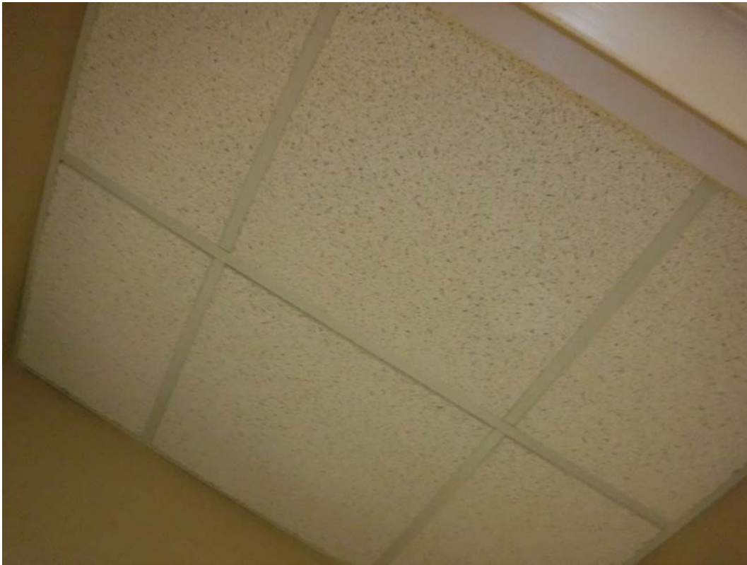
Interior, 2 nd floor- non-asbestos containing ceiling tile
