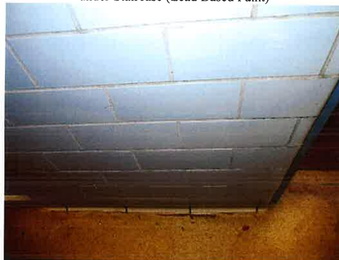
Space Identification # 1002 – Assay # 14 - Ceramic Wall Tile (Lead Based Glazing)
