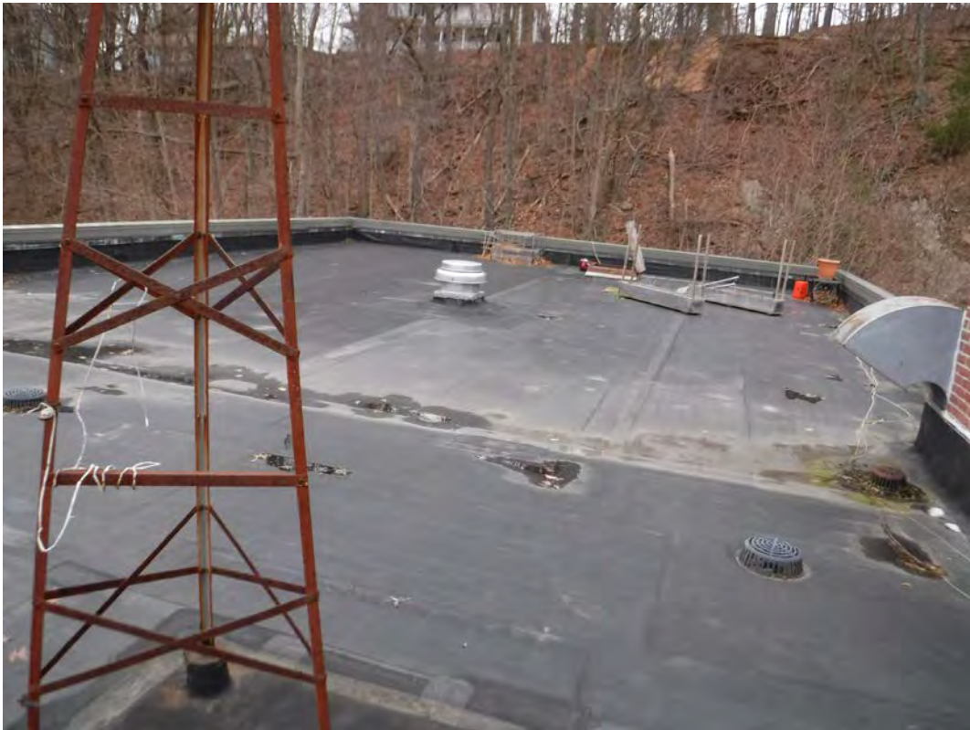
Non-asbestos containing roof membrane and flashing
