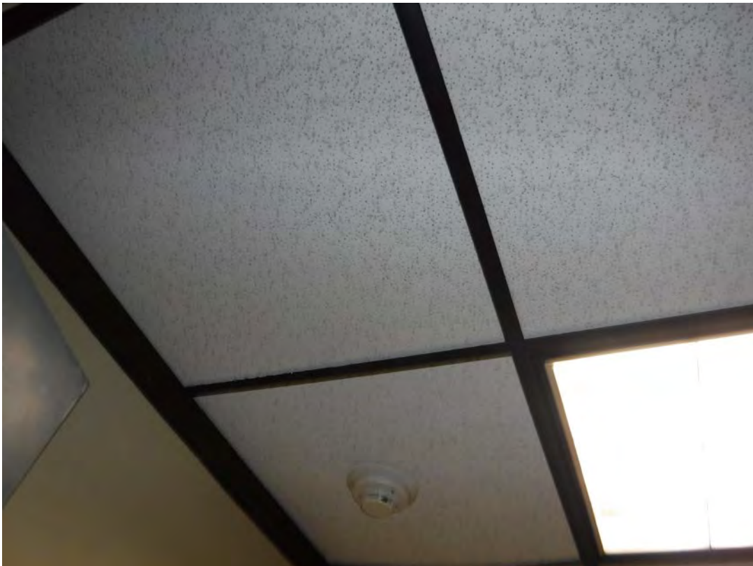
Interior, 1 st floor, dispatcher's office- non-asbestos containing 2'x2' ceiling tile
