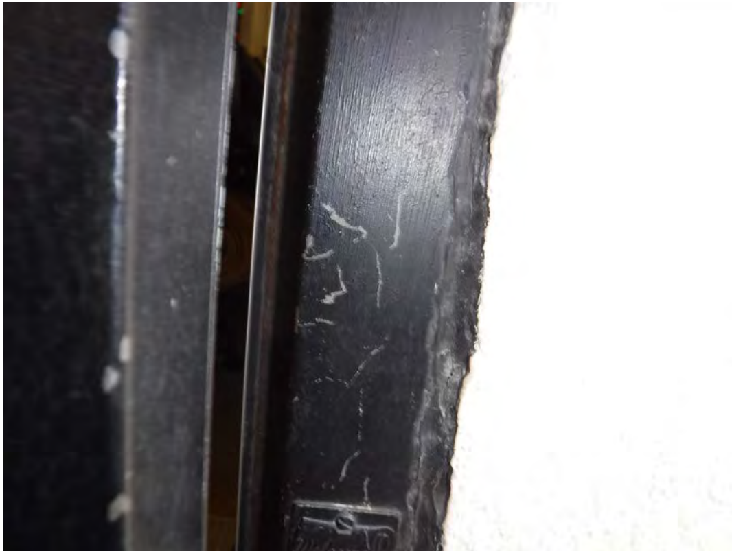
Exterior- non-asbestos containing door caulk
