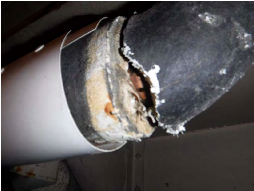
Interior, 1 st floor, dispatcher's office closet- asbestos containing pipe lagging and fitting
