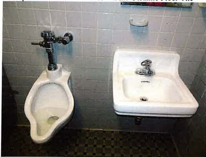
Space Identification #1005 – assay #'s 48 & 49 - White Urinal and Sink (Lead Based Glazing)
