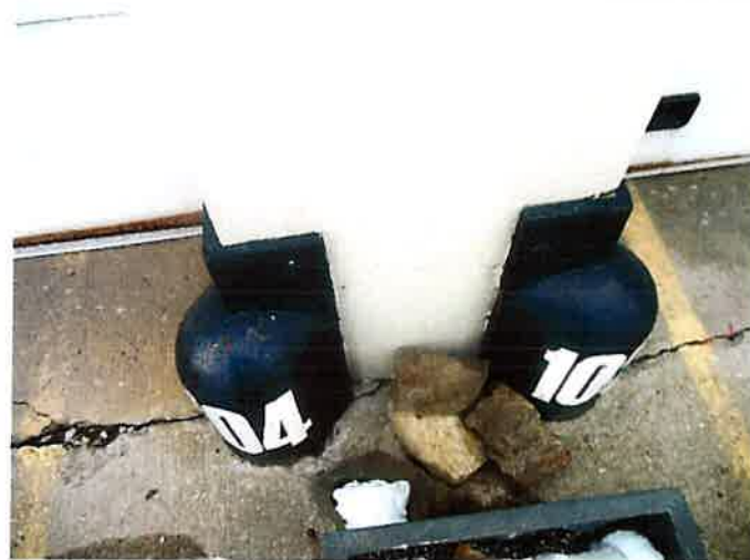
Exterior – Black Metal Corner Bumper (Lead Based Paint)
