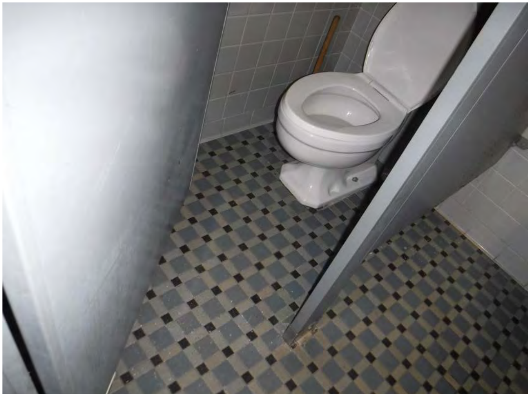
Interior- non-asbestos containing wall tile and floor tile grout
