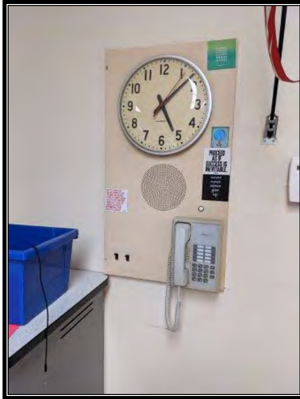
Photo 3: Non-ACM Gypsum Board (P.A. & Clock)
