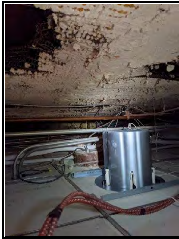
Photo 4: Non-ACM Ceiling Plaster in Ceiling Plenum
