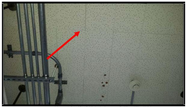
Photo # 01: 1'x1' Pinhole Pattern Ceiling Tile, White
