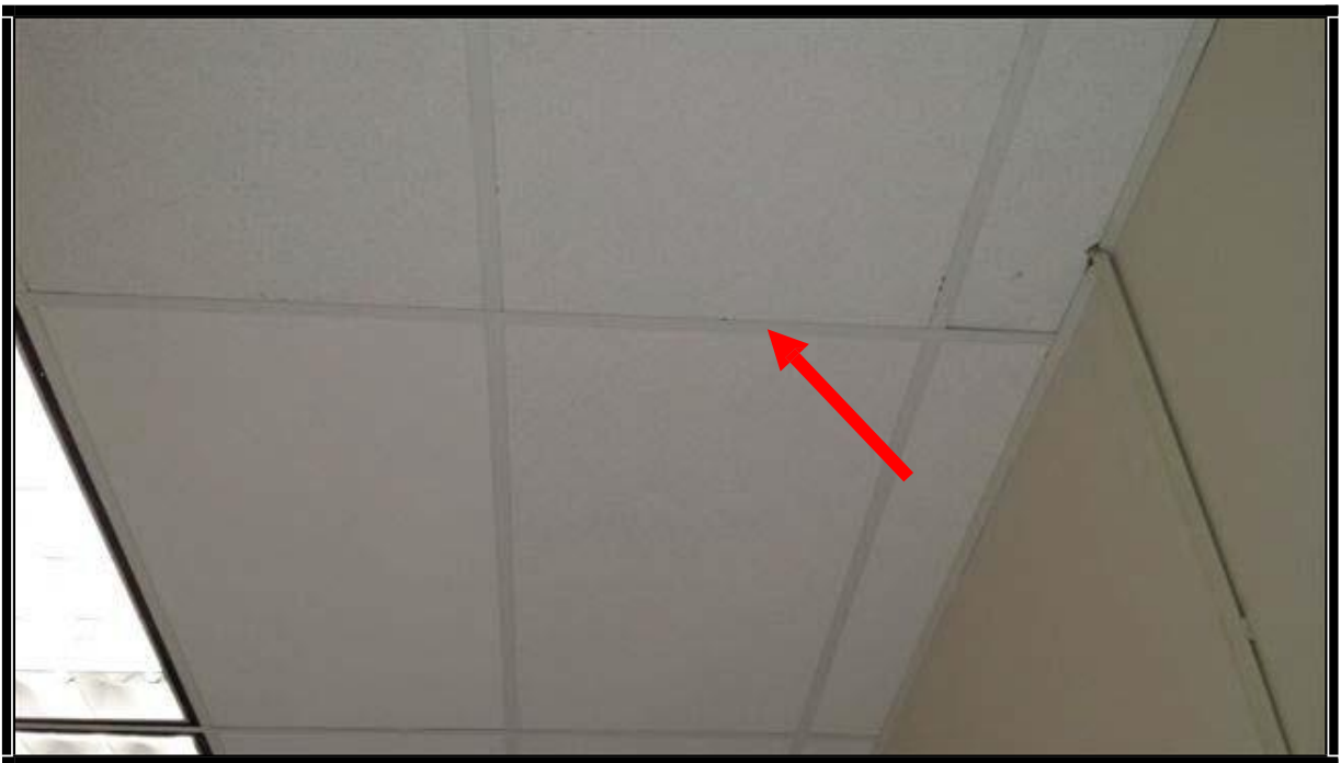
Photo # 04: 2'x4' Small Pinhole Ceiling Tile, White
