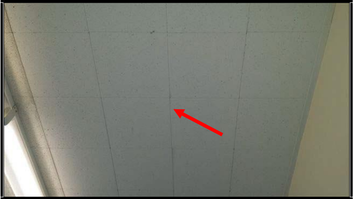
Photo # 05: 1'x1' Fissured Ceiling Tile, White
