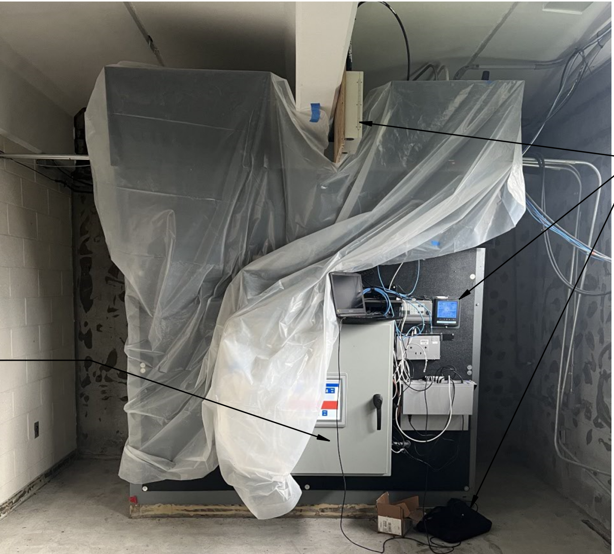
EXISTING SCADA PANEL & ASSOCIATED PERIPHERAL EQUIPMENT LOCATION DETAIL
