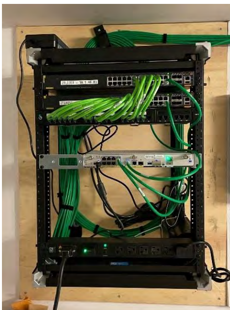
Illustration 1 – Example of Utility Room size Data Network Equipment Rack
