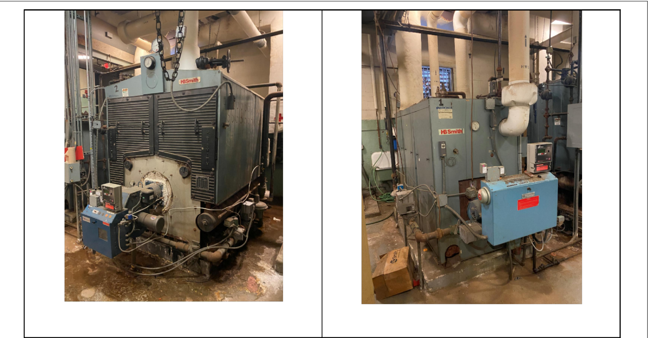
CAST IRON SECTIONAL BOILER TO BE REMOVED
