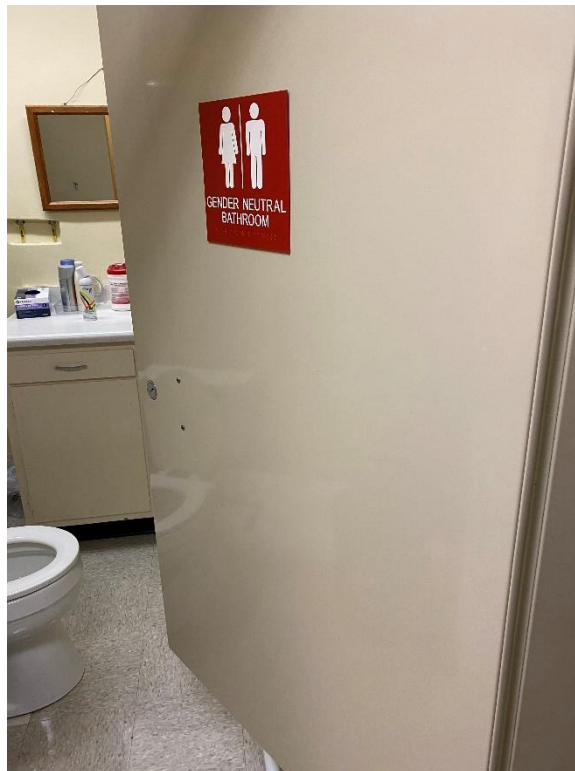
Uninsulated Metal Door
