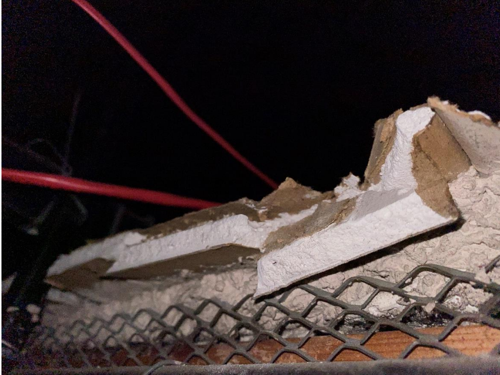
Drywall and Joint Compound
