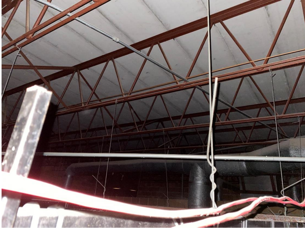
Plenum Showing Concrete Deck
