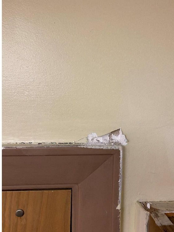
Wall Plaster White and Brown Coats
