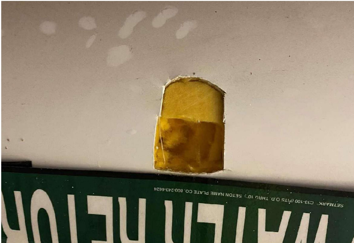
Photo 19: Yellow Insulation, Chiller Pipe Runs
