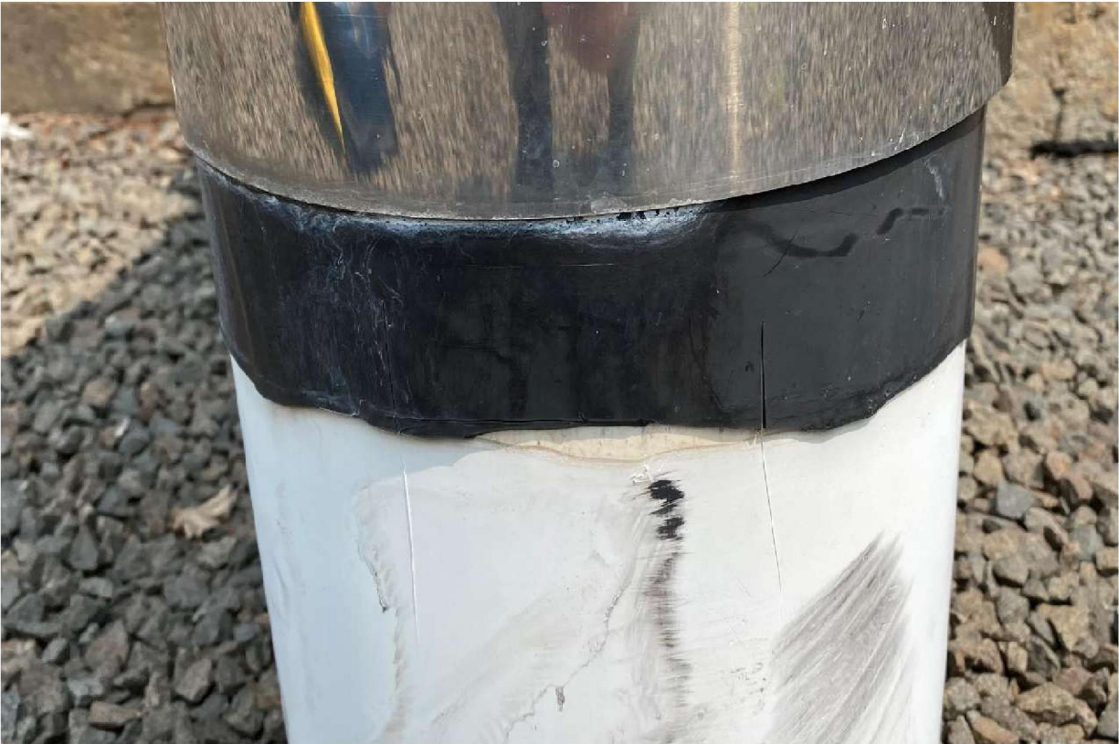
Photo 3: Double Wall Pipe Transition
