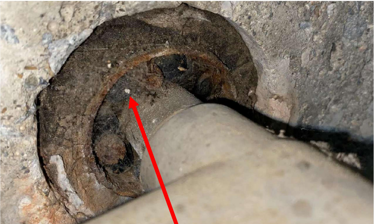
Photo 18: Underground Electrical Line Putty
