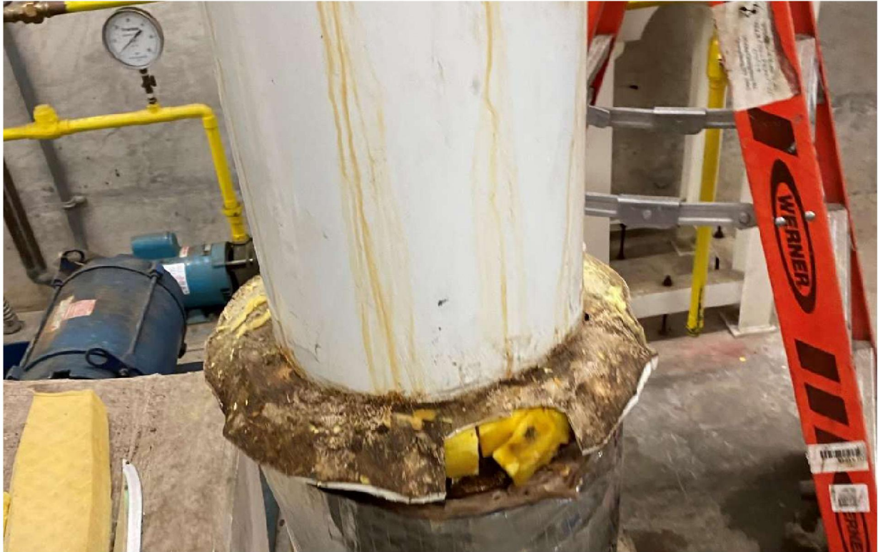
Photo 15: Solid Plastic Jacket, Brown Insulation, and Yellow Pipe Run Insulation
