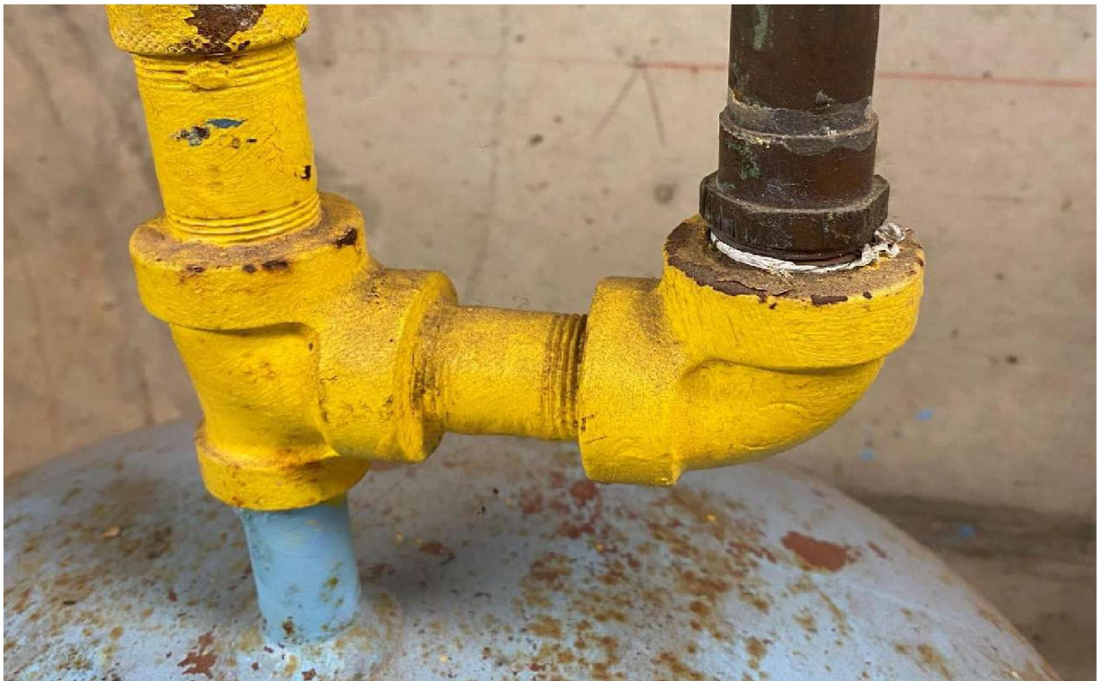
Photo 20: Yellow Pipe Paint, Interior Auxiliary Chilled Water Equipment (Lead-Based Paint)
