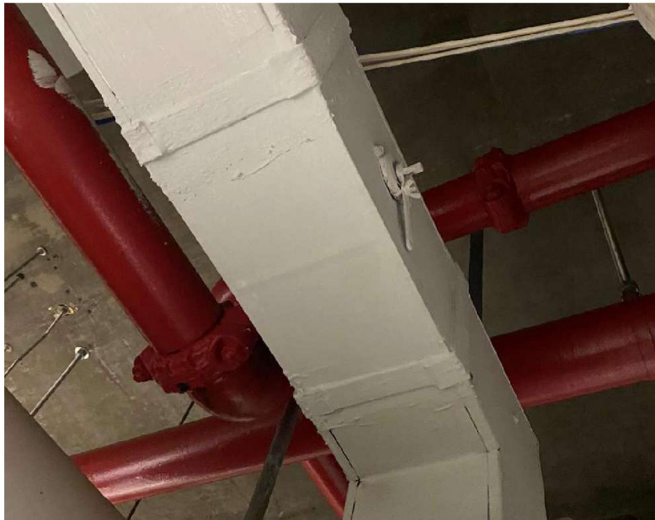
Photo 6: Grey Mastic, Supply Duct
