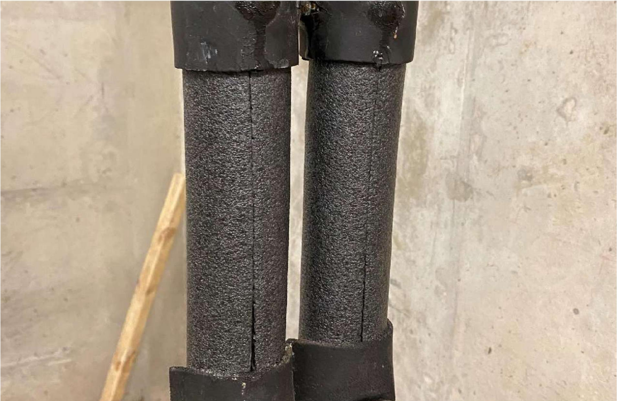
Photo 17: Black Spray Foam Insulation, Chiller Condenser Lines
