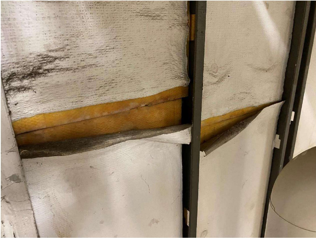
Photo 13: Yellow Insulation and White Jacket, Chiller Room Walls
