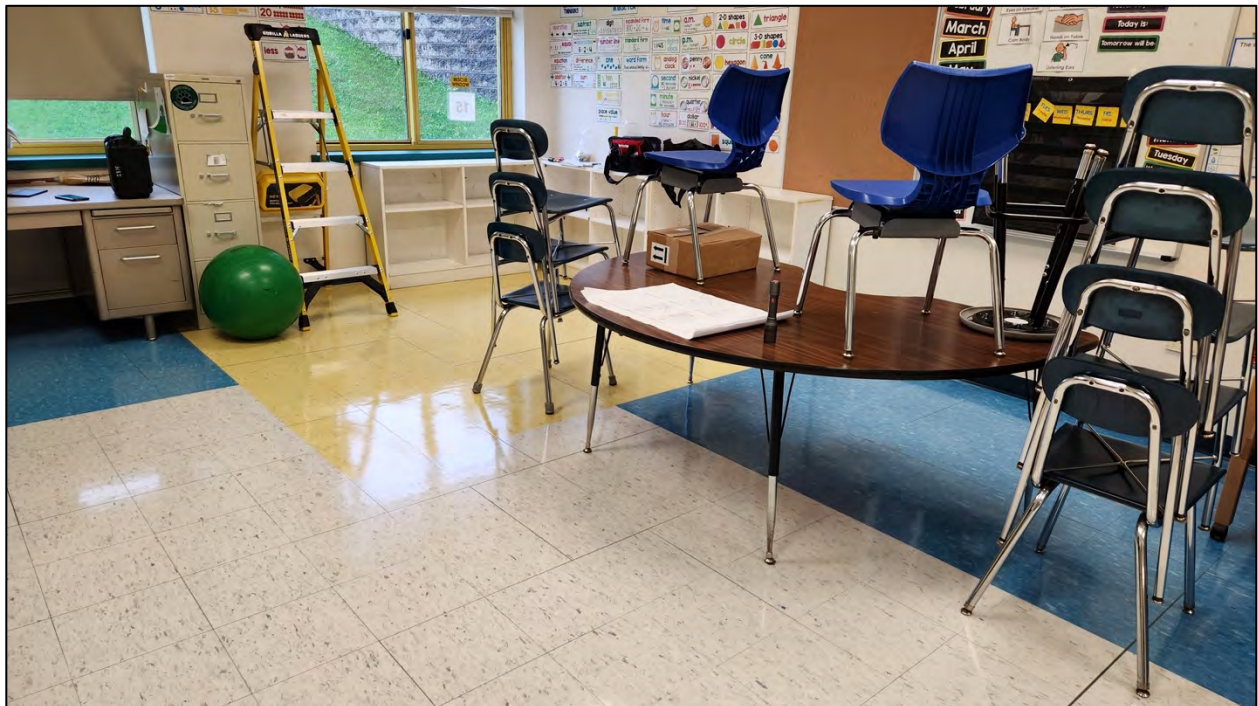
Non-asbestos containing 12"x12" Floor Tiles & Mastic, various colors (Rooms 015, 146 & Cafeteria)
