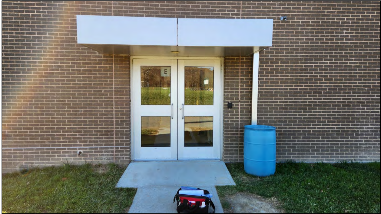
Non-asbestos containing Exterior Window/Door Frame Caulk, Expansion Joint Caulk, Exterior Brick Mortar and Overhang Roofing Materials (Corridor 170 & Exit E)
