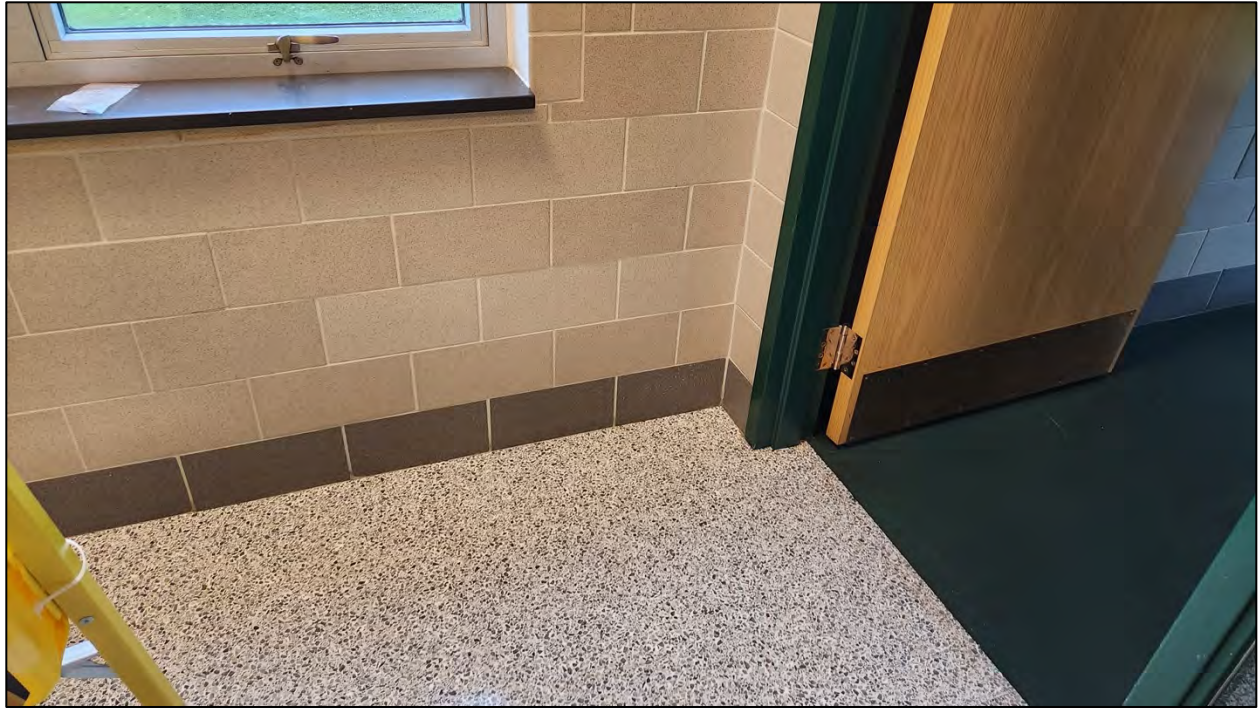
Non-asbestos containing Fritz Tile, Adhesive & Ceramic Wall Tile Mortar (Corridor 170 & Exit E)
