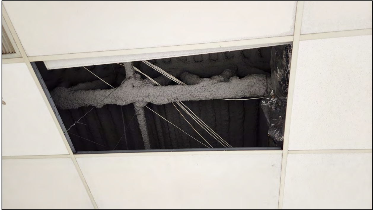
Non-asbestos containing Spray-on Fireproofing (Rooms 015, 146 & Cafeteria)
