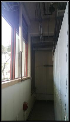
Photograph 3: Inside Electrical Room – Materials found inside the Electrical Room which may be affected by SOW were Non-ACM sheetrock, joint compound, fittings insulation, wrap around fiberglass pipe, cinderblock and 1'x1'pinhole ceiling tiles with mastic.
