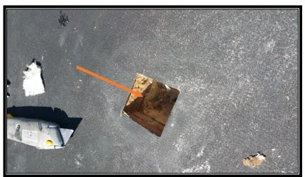
Photograph 2: Typical Roofing System for Roof G & Café Roof – Gypsum Planking on Metal Deck, Roofing Felt Paper, Brown Insulation, Roofing Rubber Membrane w/ Glue & Tar on Roofing Membrane.
