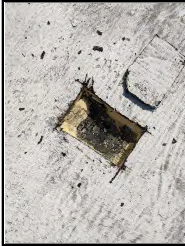
Photo 1: ACM Tar Vapor Barrier (Roof F)
