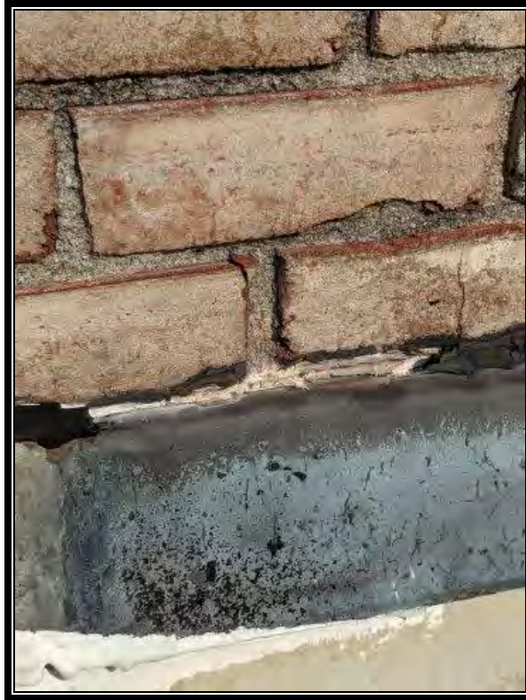
Photo 7: Non-ACM Metal Flashing Caulking, White/Tan
