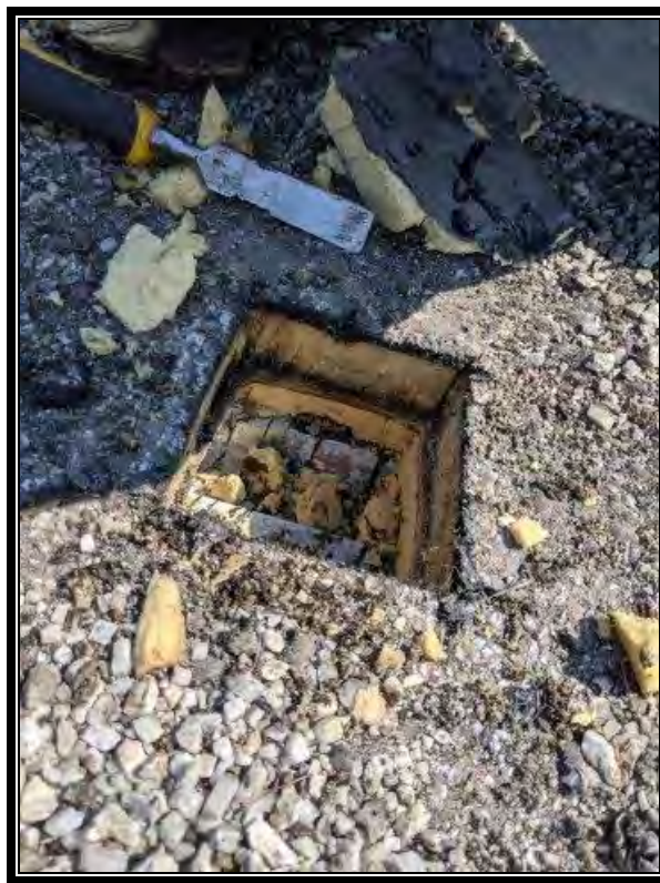
Photo 4: Non-ACM Roofing System (Roof Membrane, Old Roof Membrane, Roof Insulation, Tar on Metal Deck)
