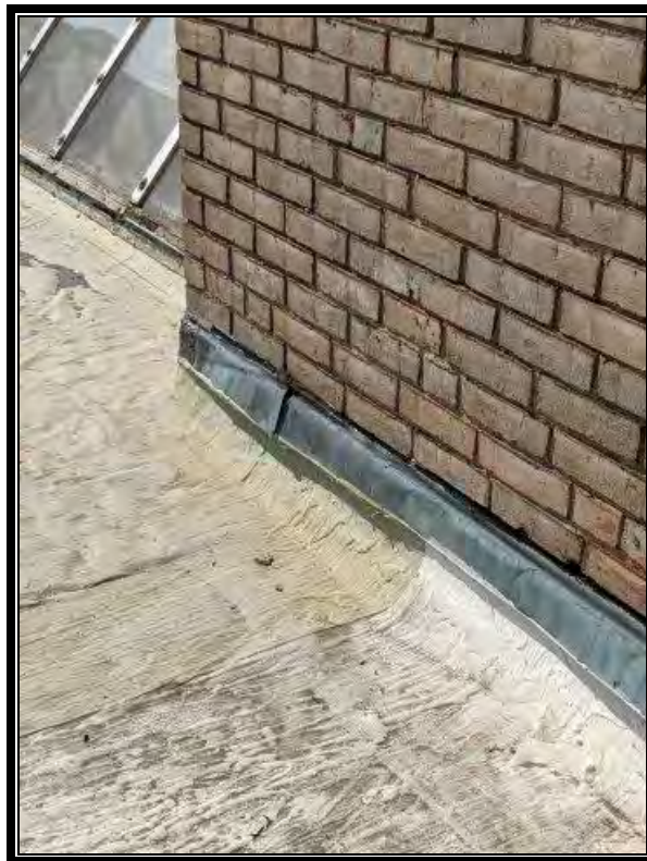
Photo 6: Non-ACM Metal Flashing Caulking, Black
