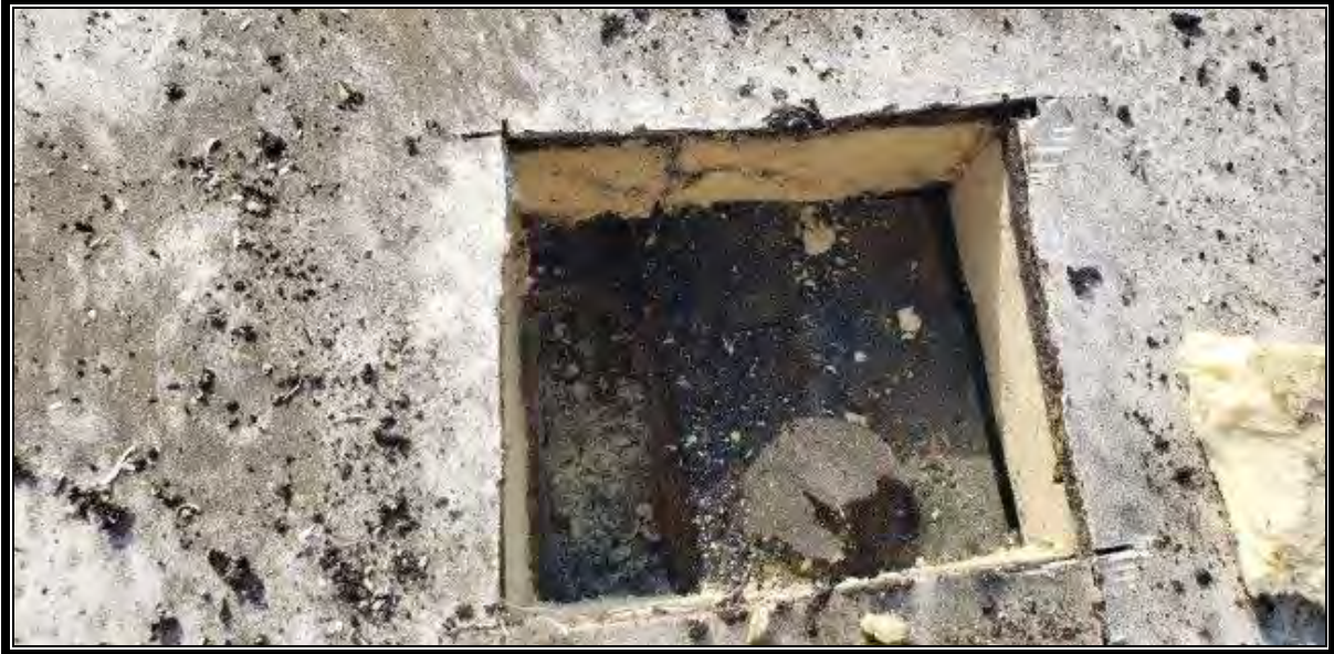
Photo 3: Non-ACM Roofing System (Coating on Membrane, Roof Membrane, Tar on Metal Deck)
