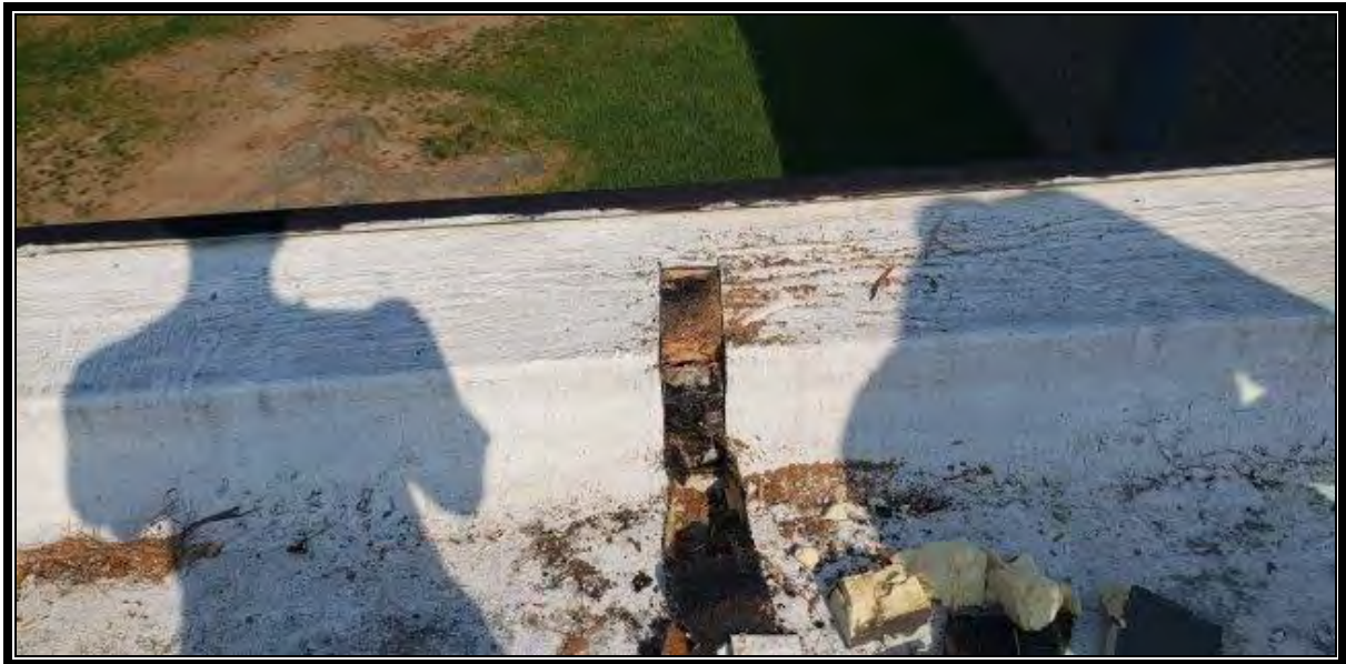
Photo 2: ACM Roof Flashing and Fiberboard Flashing Insulation.
