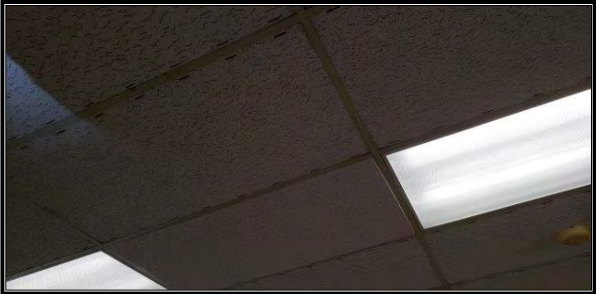
Photo 13: Non-ACM 2'x4 Ceiling Tile
