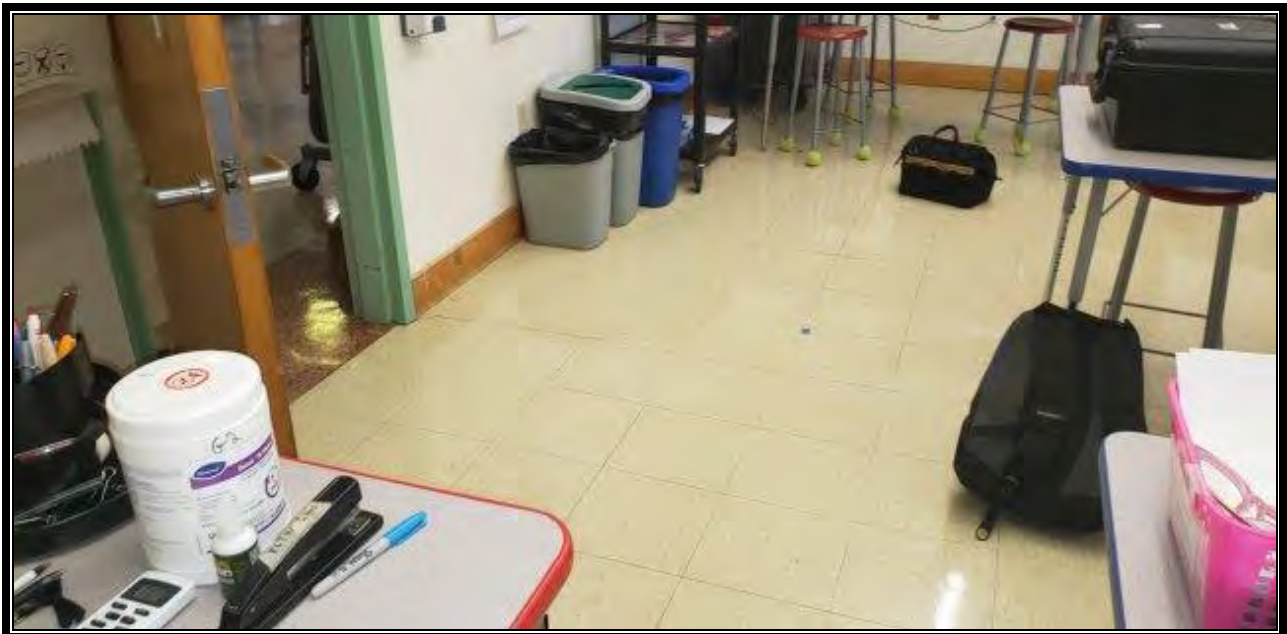
Photo 2: Non-ACM 12"x12" Floor Tile (Beige) and Associated Mastic (Black)
