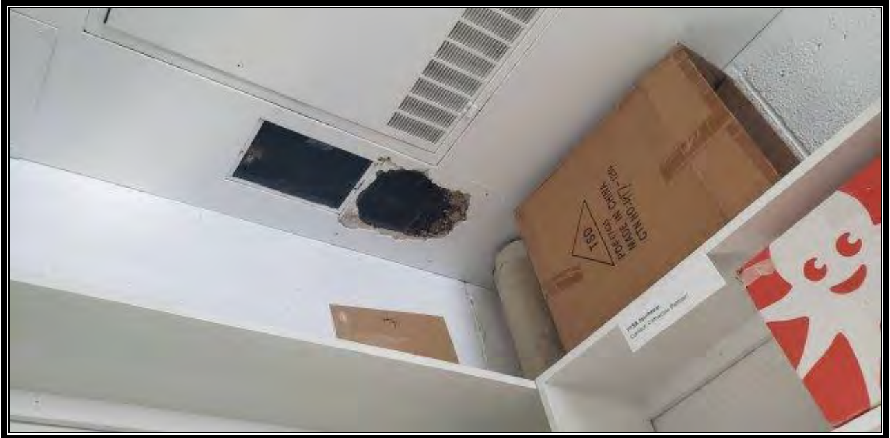
Photo 5: Non-ACM Ceiling Plaster (White & Brown Coats)
