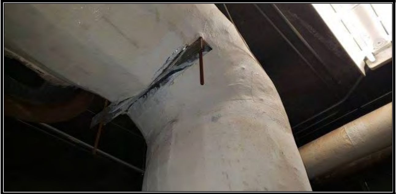
Photo 5: Non-ACM Fiberglass Boiler Breeching Canvas (Beige)-Gym Building
