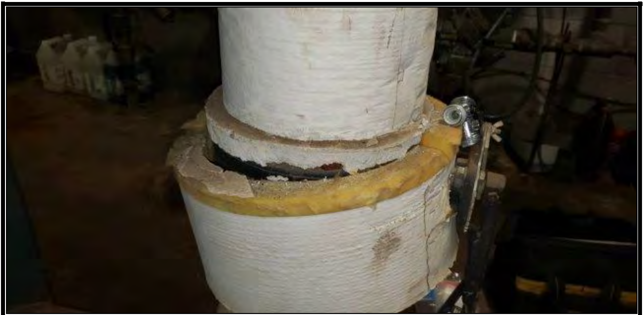
Photo 6: Non-ACM Fiberglass Pipe Edge Cementitious Sealant (Gray) -Gym Building
