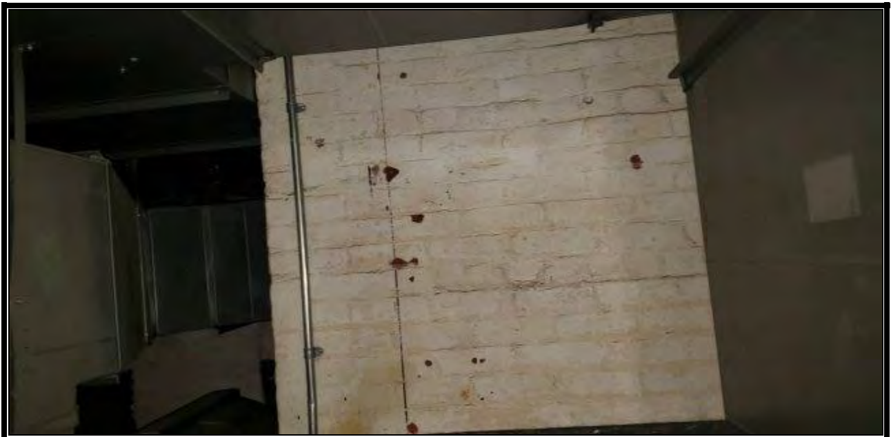
Photo 4: Non-ACM Chimney Brick Mortar (Gray) -Gym Building
