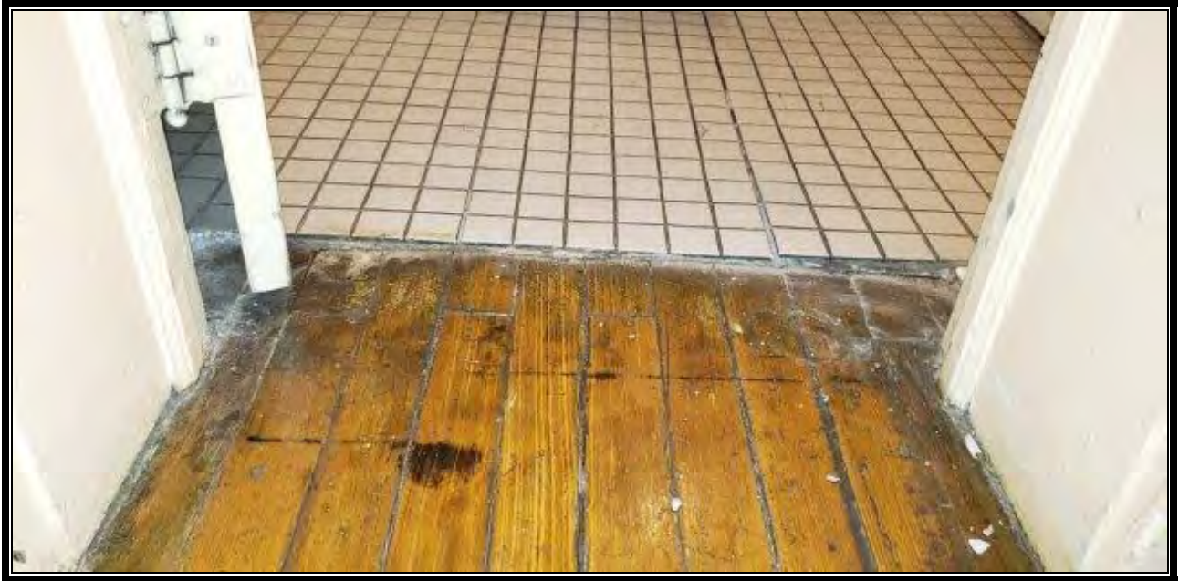
Photo 1: ACM 9"x9" Floor Tile (Brown) under Ceramic Floor Tile-Main Building
