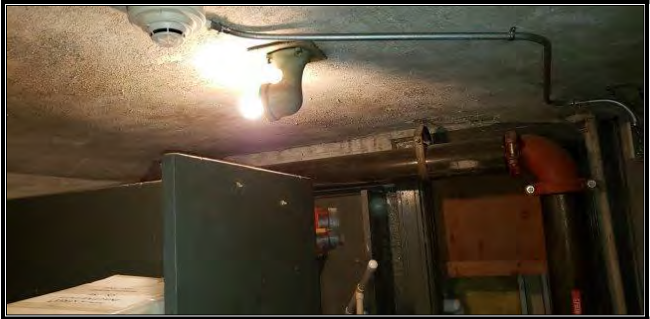
Photo 11: Non-ACM Cementitious Ceiling Material (Gray)-Main Building
