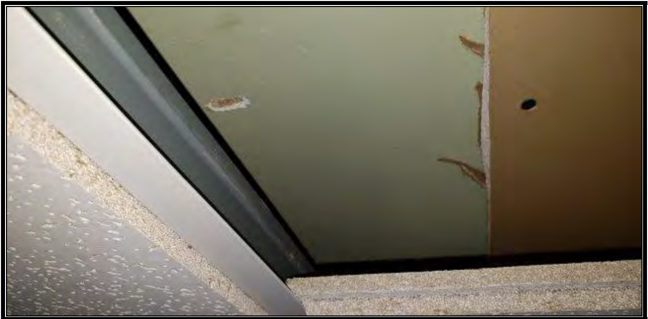
Photo 10: Non-ACM Wall Plaster (White and Brown Coats)-Main Building
