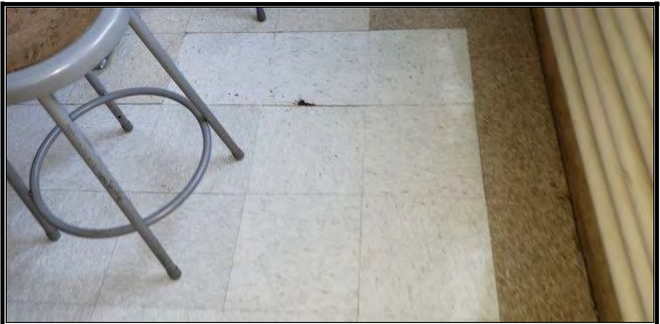
Photo 18: Non-ACM 12"x12" Floor Tiles (White) and Associated Mastic (Brown/Yellow)
