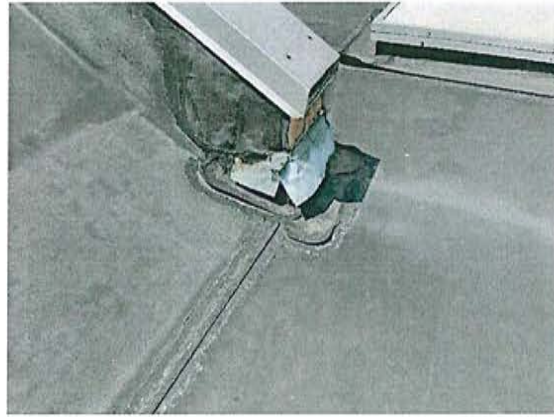
Damaged counter flashing.
