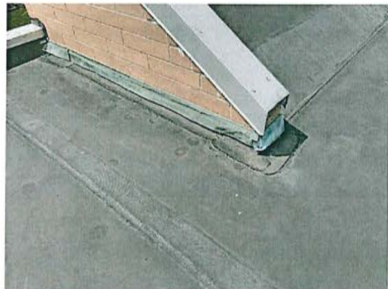
Damaged counter flashing.
