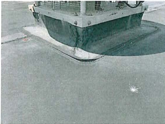
Failing Seam.
