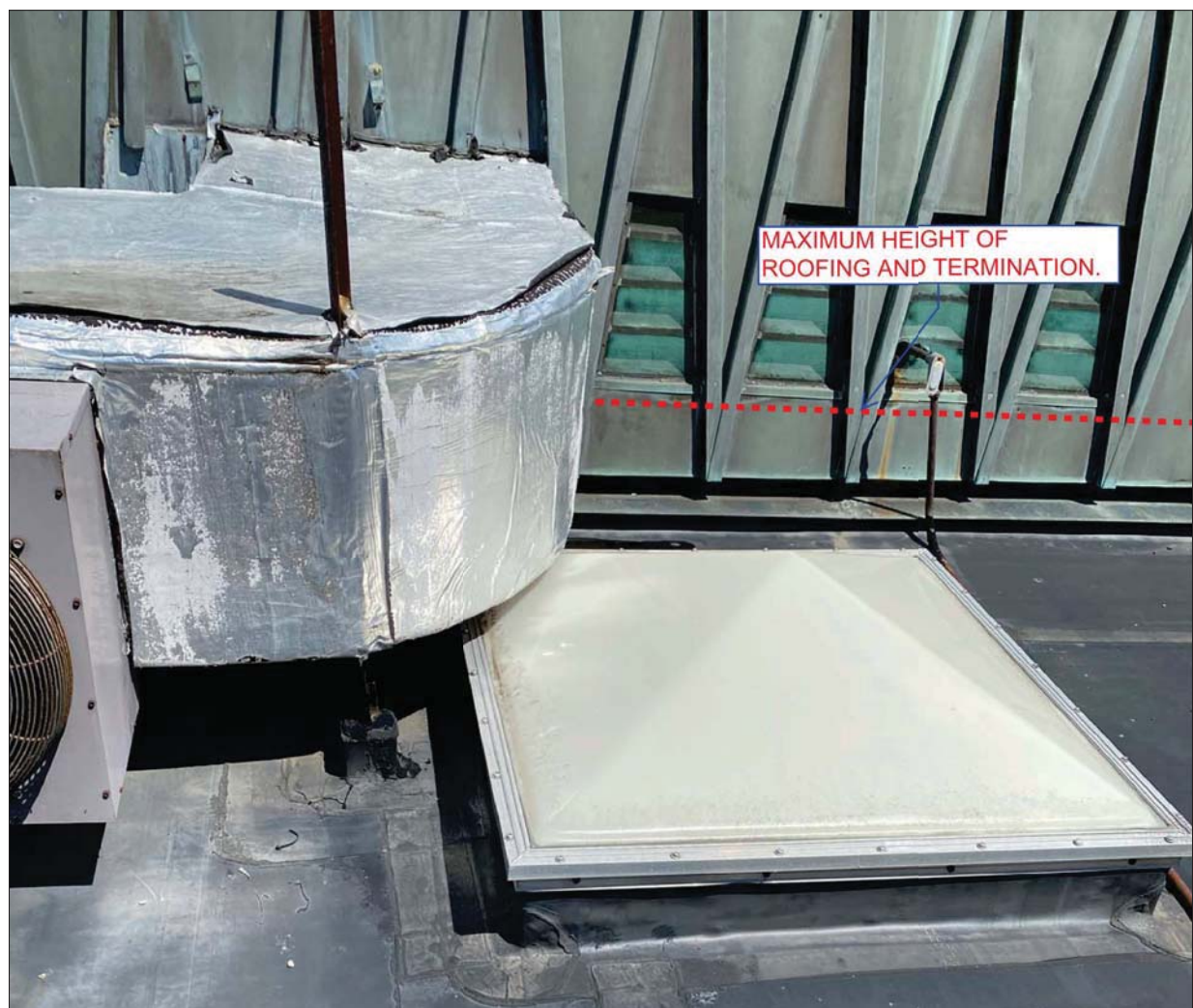
P2 PHOTO 2 AT ROOF "R8" EXISTING WALL VENTS A103 SCALE: NOT TO SCALE
