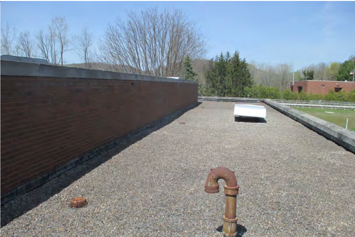
Photo #5 - View of the lower roof level on the Blower building. The roof system has ballast on top of a rigid ISO insulation board on top of the asbestos-containing built-up roofing on the concrete roof deck.
