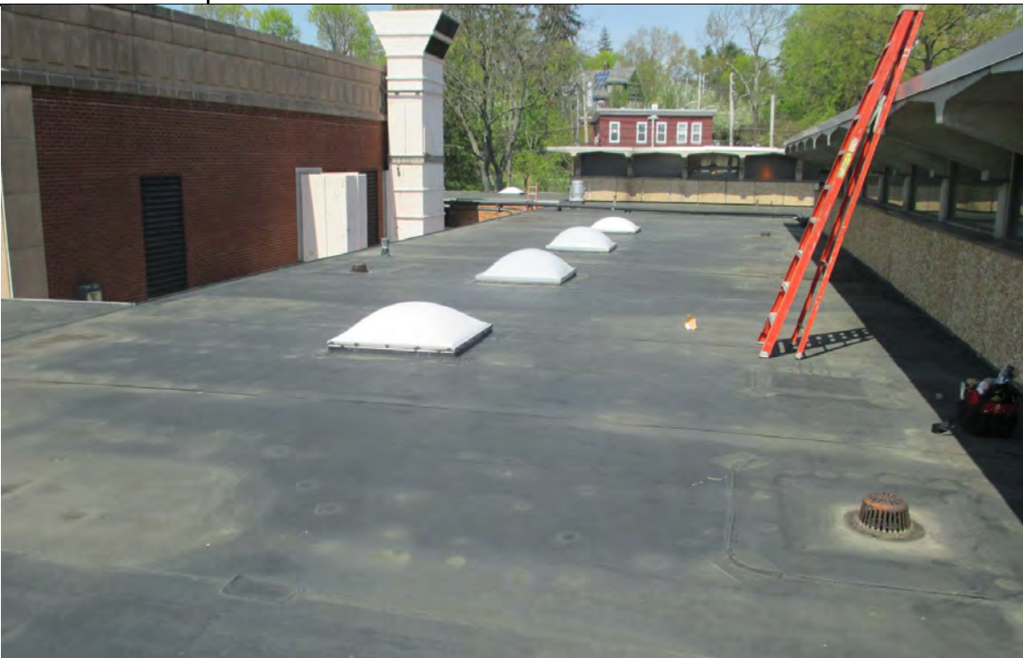
Photo #6 - View of the middle roof area between the Influent and Effluent Wing roofs. There are four (4) skylights on this level in addition to the eight (8) that are on the Influent Wing roof. The ladder to the right gains access to the upper roof level on the middle/Effluent Wing roof.
