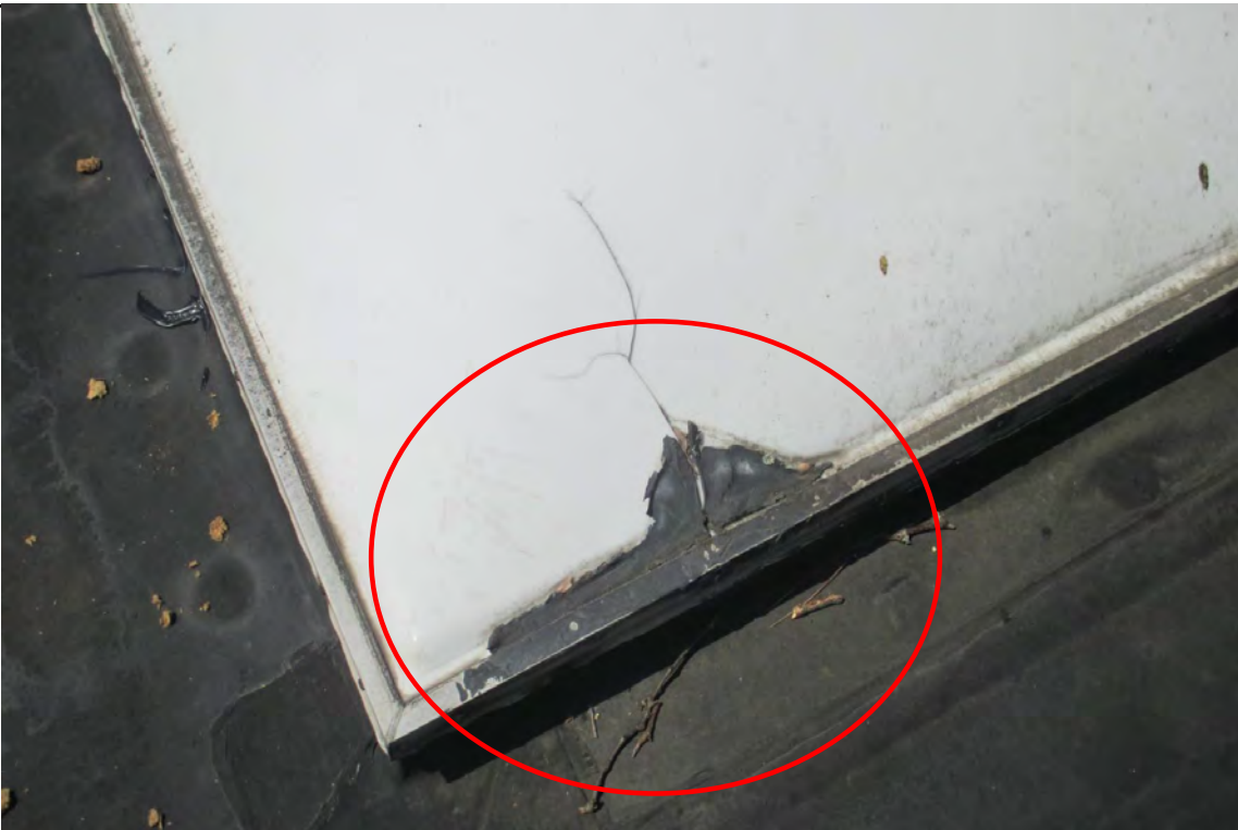
Photo #3 - View of the asbestos-containing roof patch tar (red circle) that was found on most of the skylight domes.
