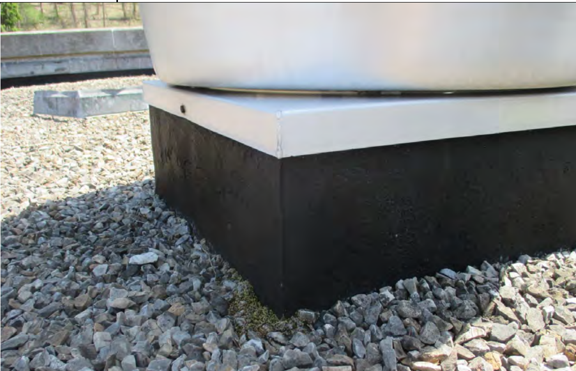
Photo #4 - Close-up view of the curb to the mechanical equipment on the Administration building roof. The asbestos-containing roof flashing tar exists around the curbs to the mechanical equipment and roof hatch.
