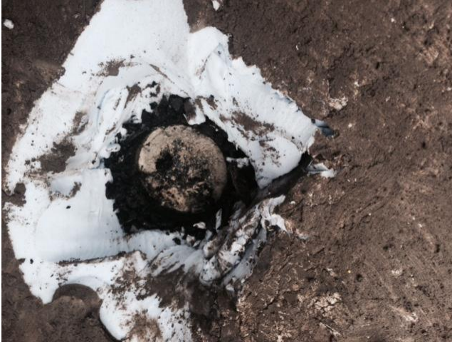
Photo exhibits 2" of EPS insulation over a 4 ply built up membrane and concrete deck.
