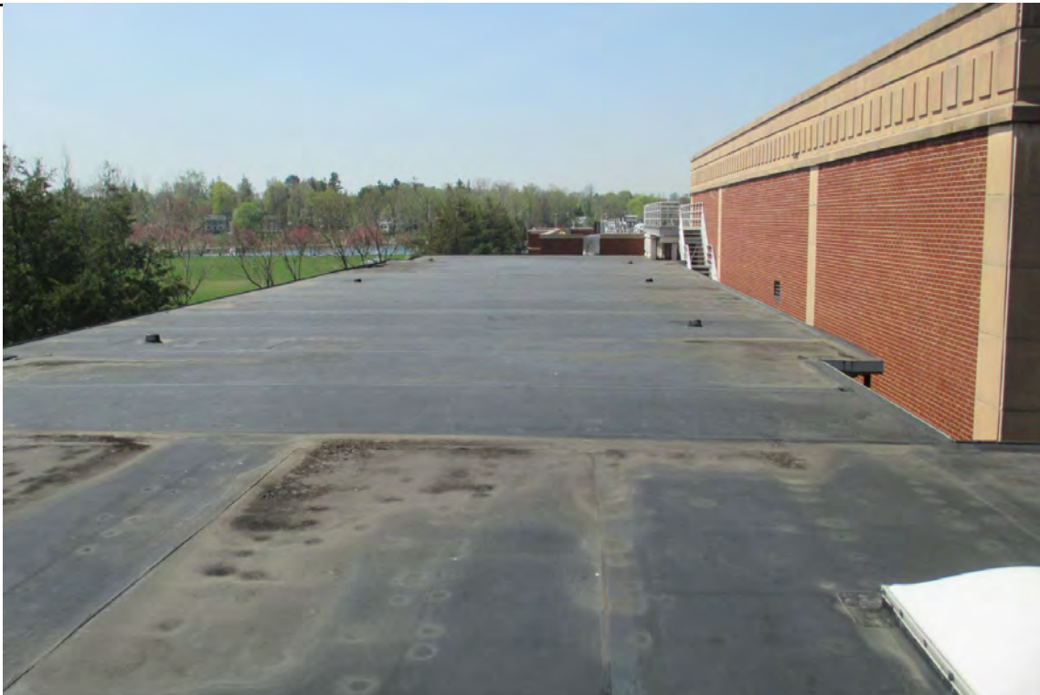
Photo #5 - View of the Effluent Wing roof looking south. As noted before, the roofing system was homogeneous amongst all roof levels on the Primary building. (EPDM membrane layer, rigid ISO insulation board, tar paper on concrete roof deck).
