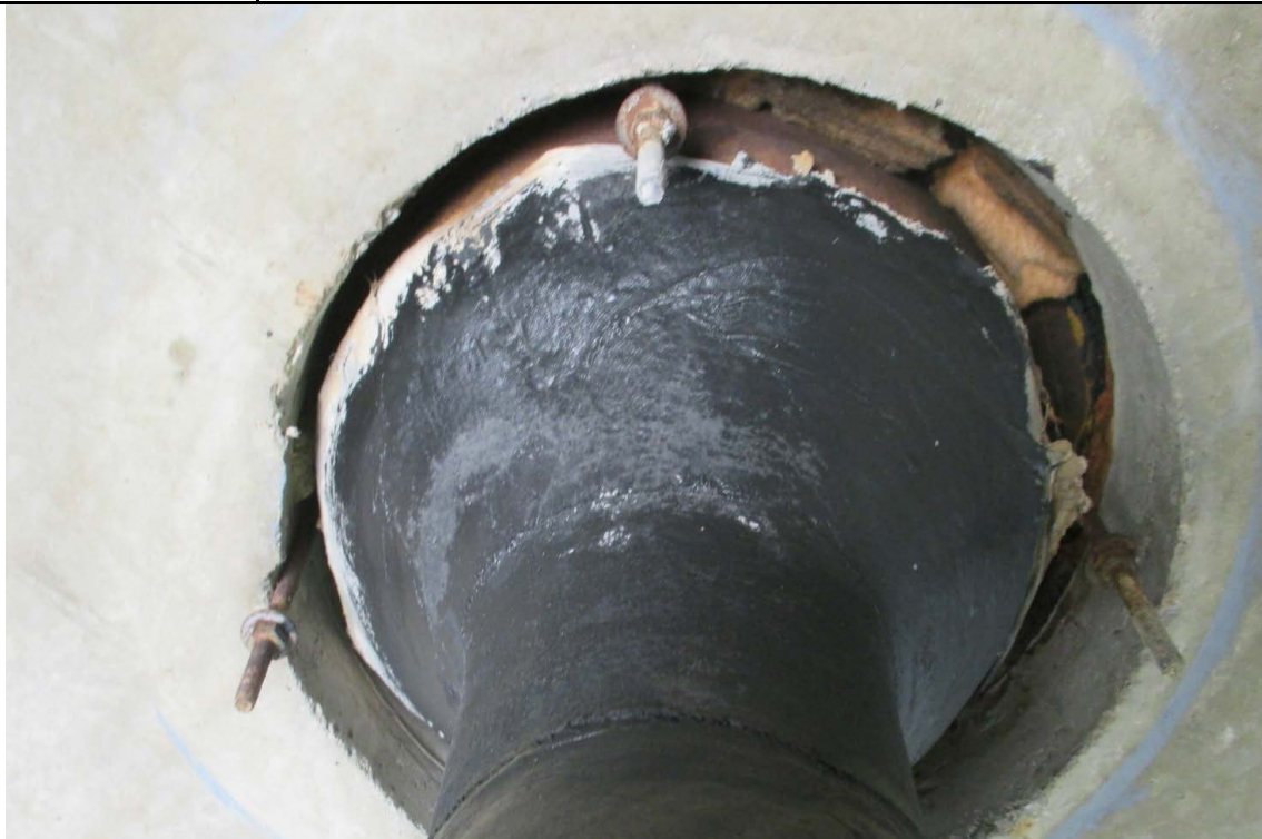
Photo #10 - Typical view of the roof drain insulation found within the Influent/Effluent Wings and middle building areas. The non-ACM roof drain insulation was homogeneous on all roofs.
