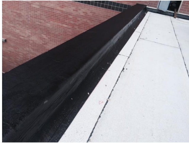
Photo exhibits the JM Perma Flash application to perimeter coping stones on recent DPW project.
