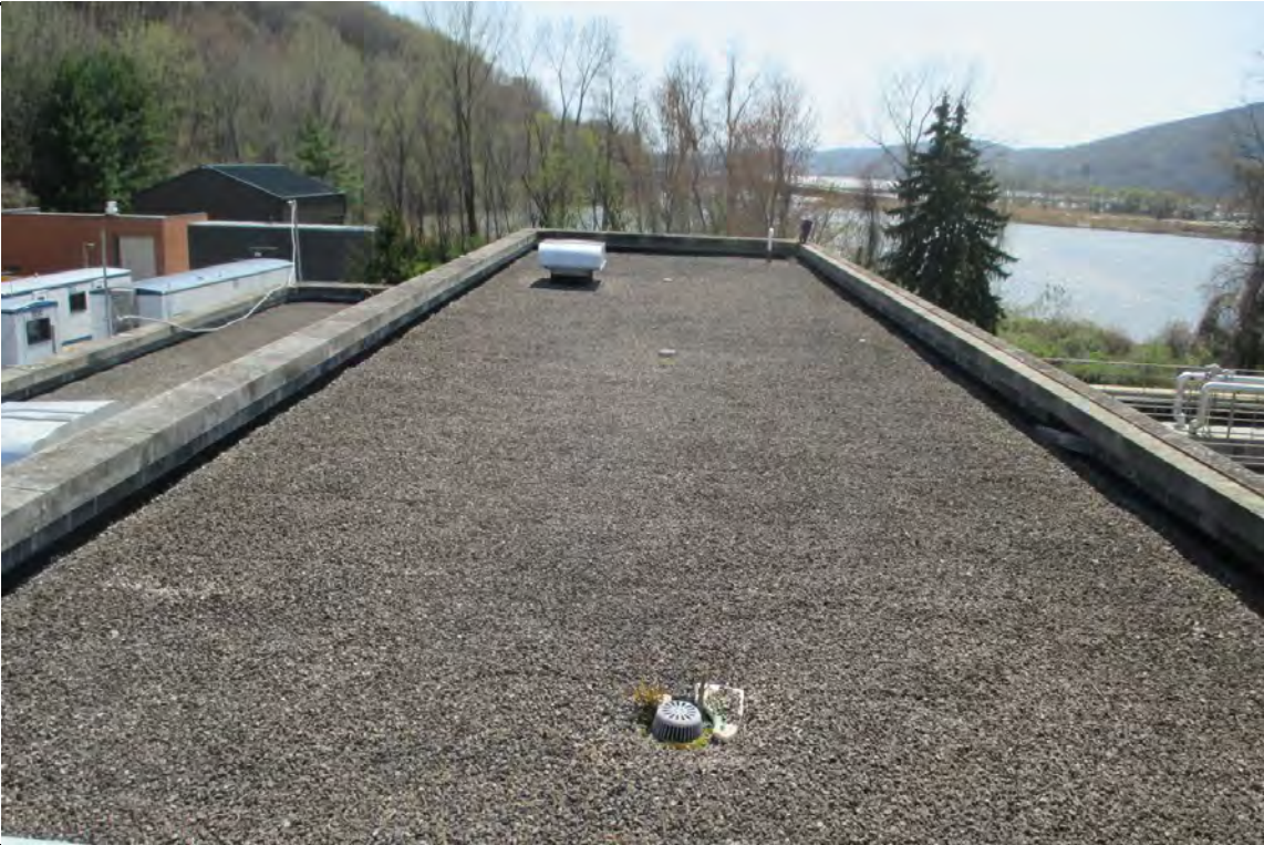
Photo #7 - View of the upper roof level on the Blower building. The roof system has ballast on top of a rigid ISO insulation board on top of the asbestos-containing built-up roofing on the concrete roof deck.
