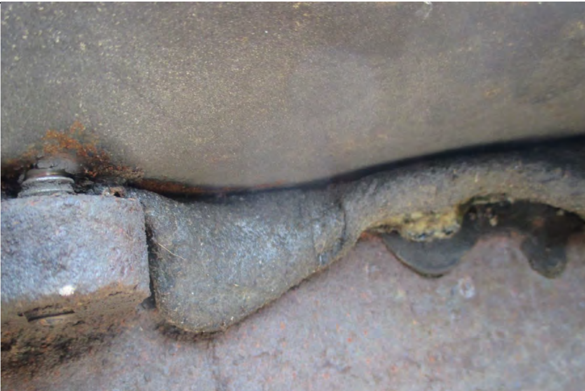
Photo #7 - View of the sealant found inside each of the roof drains.
