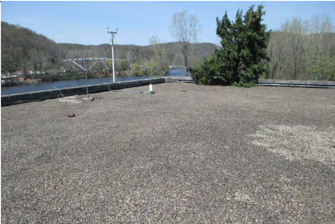
Photo #1 - General view of the roof on the Administration building. The system has ballast on top of a rigid ISO insulation board on top of the asbestos-containing built-up roofing which is on the concrete roof deck.
