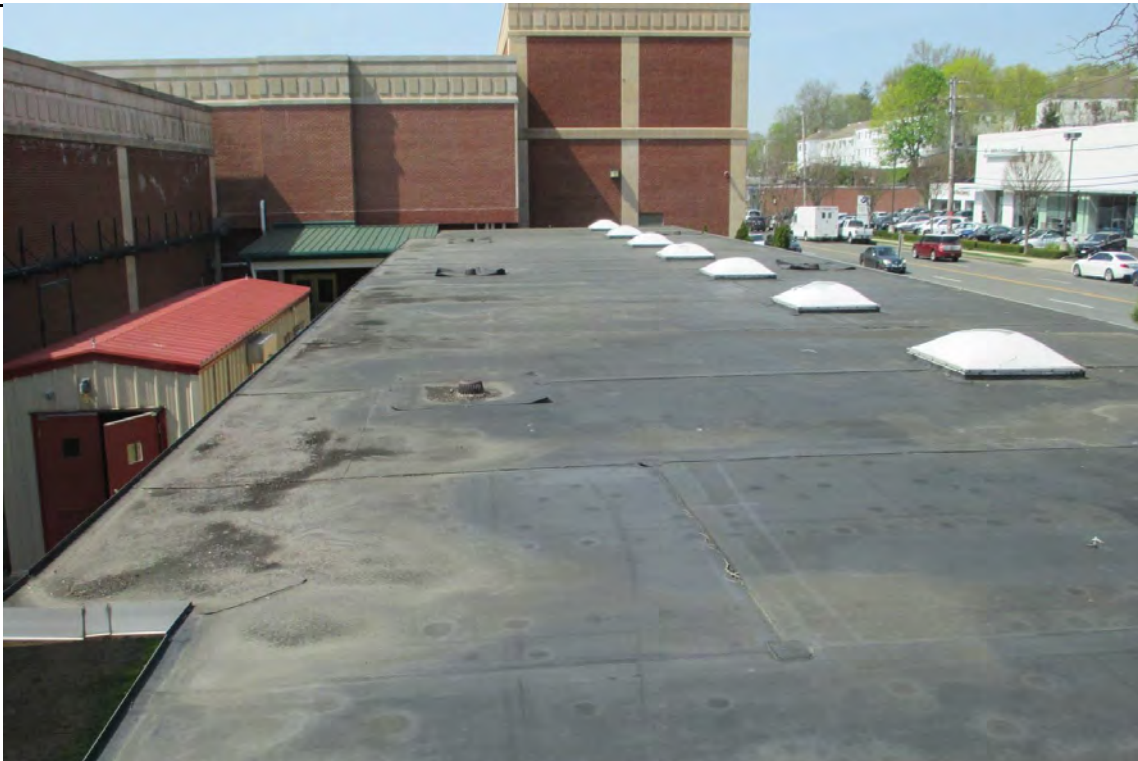
Photo #1 - View of the roof over the Influent Wing looking south. There are a total of eight (8) skylights on the Influent Wing roof, with some have asbestos-containing roof patch tar.
