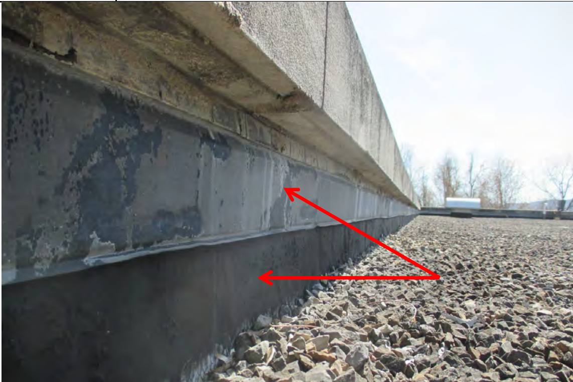
Photo #8 - View of the upper level of the Blower building roof. The upper red arrow shows the lead-containing metal flashing and the lower red arrow shows the asbestos-containing flashing tar.
