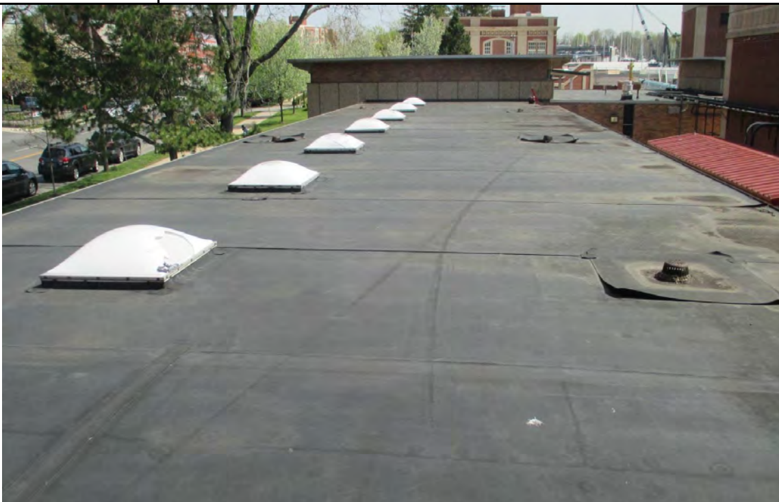
Photo #2 - View of the roof over the Influent Wing looking north. The roof system consists of a EPDM roof membrane top layer, a rigid ISO insulation board, and then a tar paper on the concrete roof deck. This roofing was exhibited in all areas of the roofing where Watts did core sampling.
