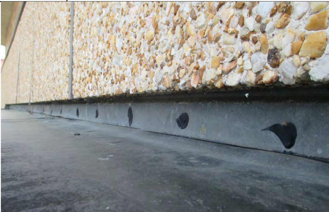
Photo #4 - View of the lead-containing metal flashing edge (view above is on the north end of the Influent Wing roof) that was found where the lower roof levels meet the raised walls to the upper roof levels (both the Influent and Effluent Wing roofs). Behind this metal flashing, there is asbestos-containing EPDM flashing tar.
