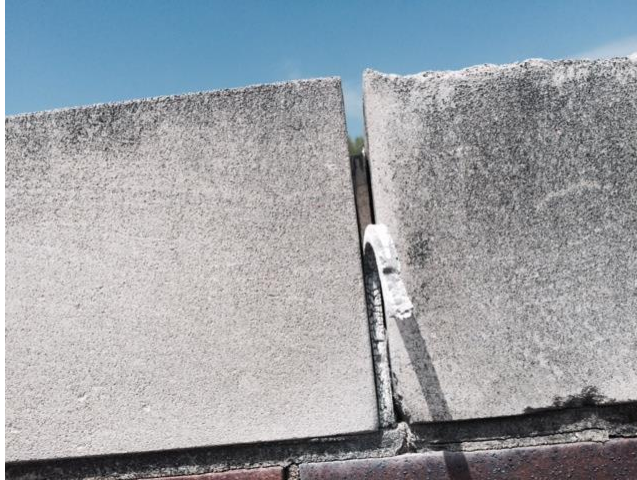
Open Coping Stone joints in need of being sealed.
