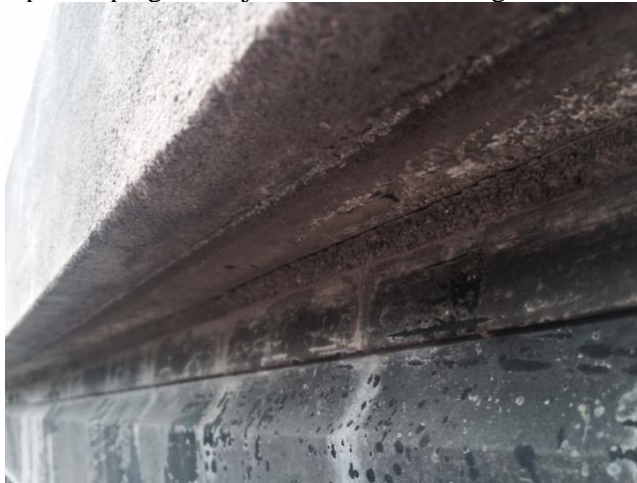
Open Coping Stone joints in need of being sealed.
