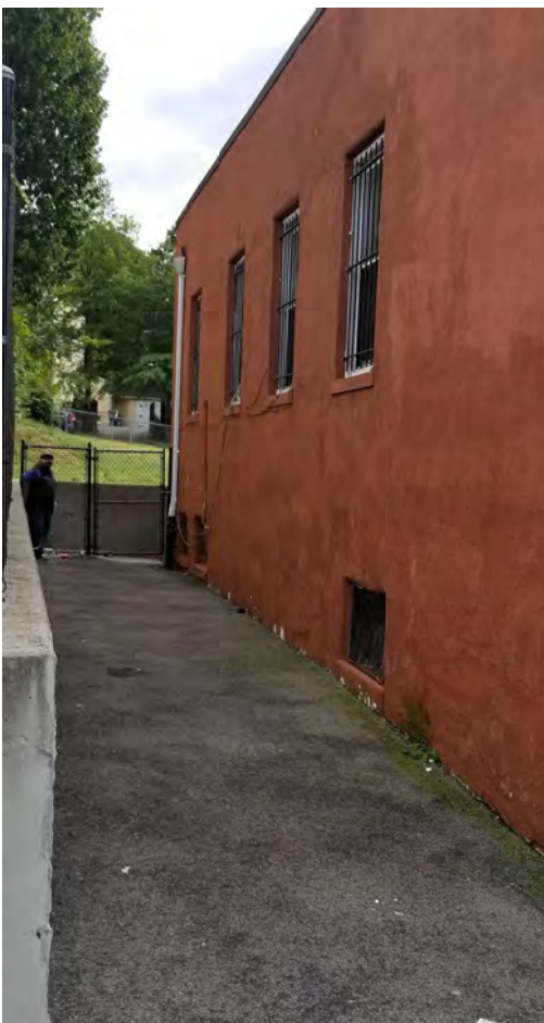
PHOTO No.4: OVERALL VIEW OF NORTH ELEVATION. EXISTING STUCCO FINISH TO BE REMOVED AND REPLACED IN ITS ENTIRETY.
