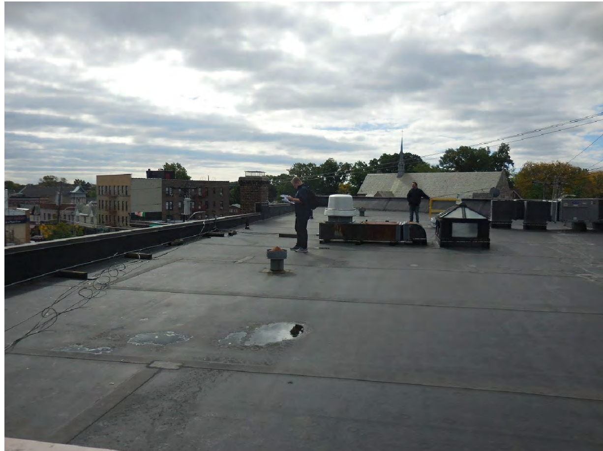
PHOTO No.9: MAIN ROOF, LOOKING SOUTH. EXISTING EPDM ROOFING TO BE REMOVED AND REPLACED.
