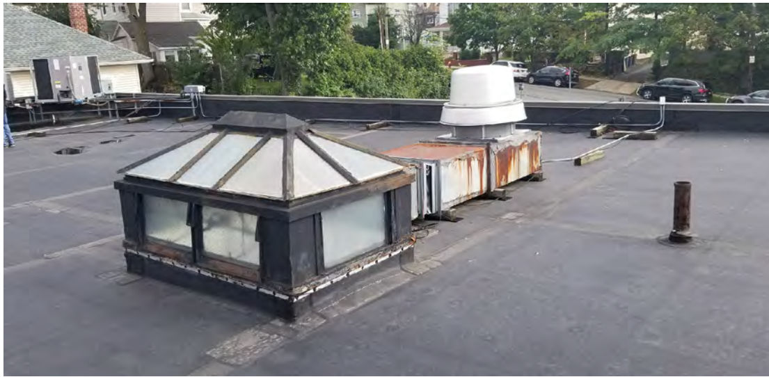
PHOTO No.15: SKYLIGHT ASSEMBLY TO BE REFURBISHED.SEE NOTE No.9 ON T-001.00.
