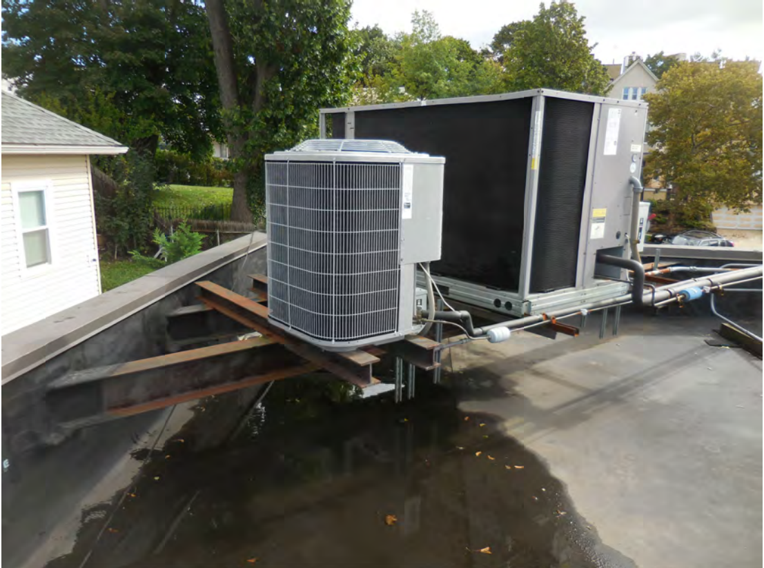
PHOTO No.12: ROOF EQUIPMENT AT NORTHEAST CORNER TO BE REMOVED AND RELOCATED. STEEL DUNNAGE SUPPORT TO BE REMOVED.
