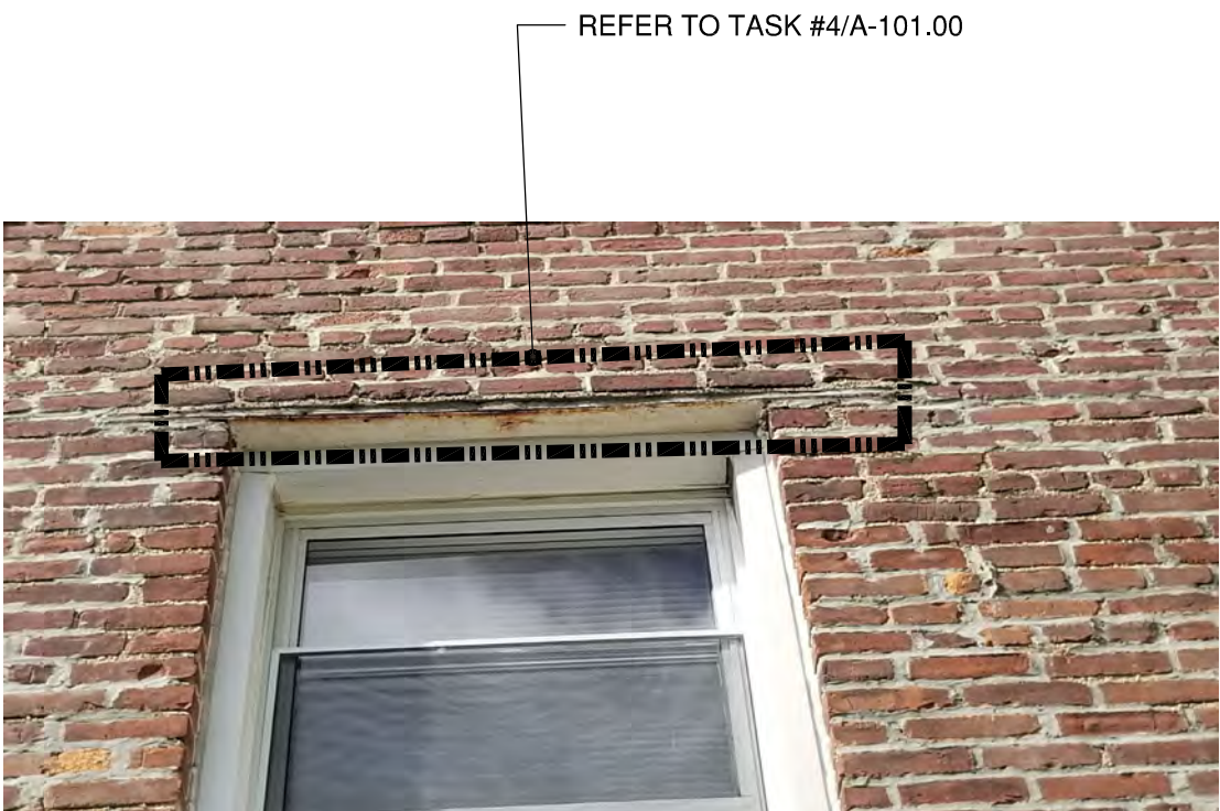
PHOTO No.6: CORRODED/DEFLECTED STEEL WINDOW LINTEL TO BE REMOVED/REPLACED WITH NEW GALVANIZED STEEL LINTEL. OPEN/ERODED MORTAR JOINTS TO BE RAKED OUT AND REPOINTED. NEW MORTAR TO MATCH EXISTING.
