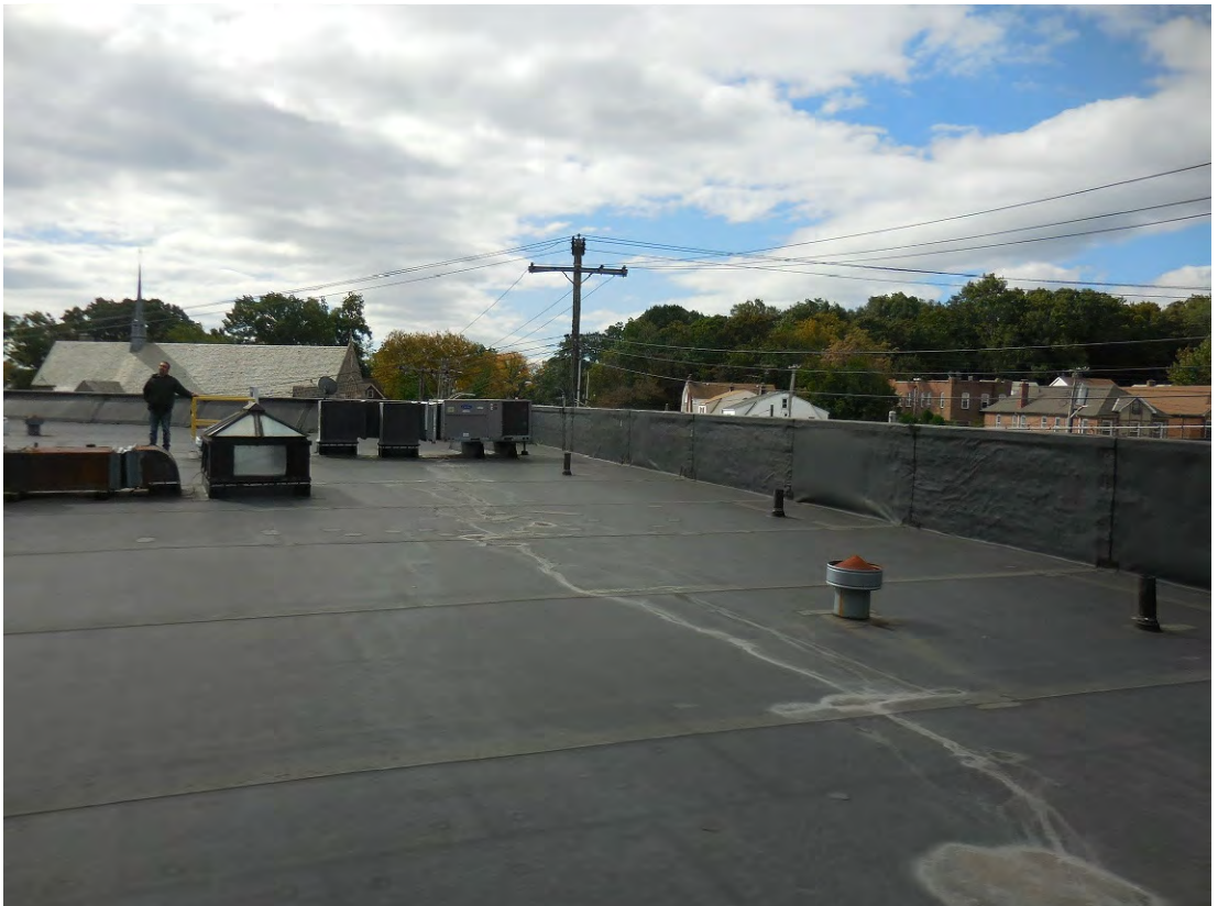
PHOTO No.10: MAIN ROOF, LOOKING SOUTH. EXISTING EPDM ROOFING TO BE REMOVED AND REPLACED.
