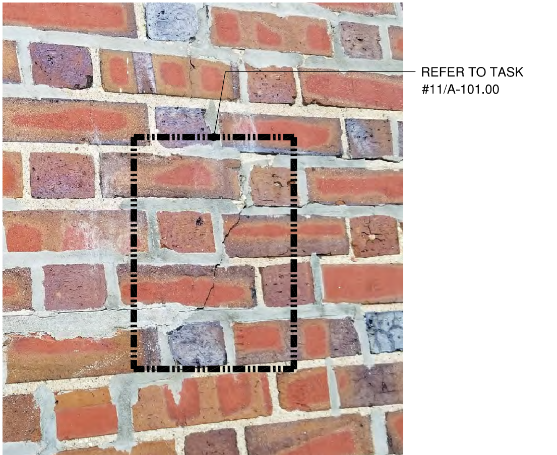
PHOTO No.7: DAMAGED BRICK MASONRY TO BE REMOVED/REPLACED WITH NEW BRICK TO MATCH EXISTING IN ALL RESPECTS.
