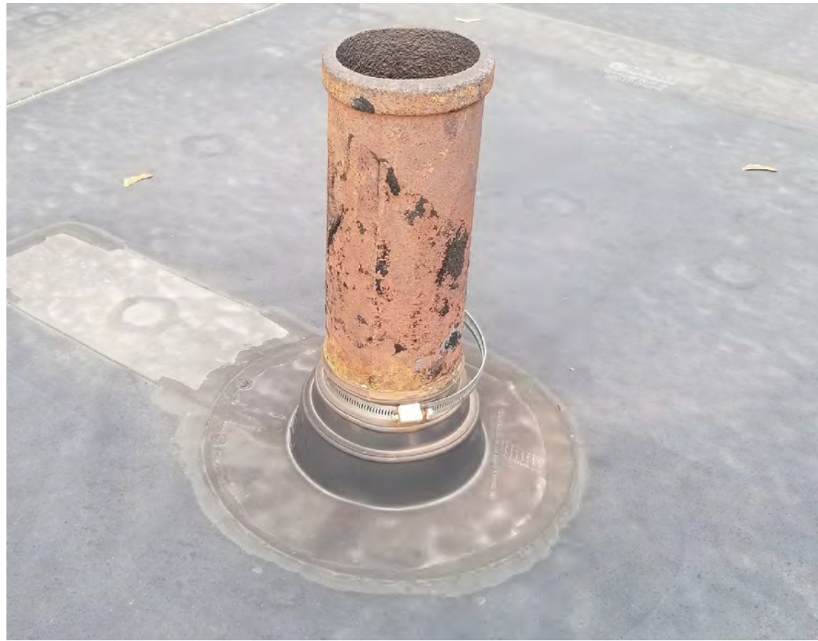
PHOTO No.13: ROOF VENT TO REMAIN. FLASH PER DETAIL 2/203.00.
