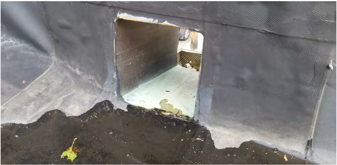
PHOTO No.16: ROOF SCUPPER TO BE FLASHED PER DETAIL 6/A-203.00.
