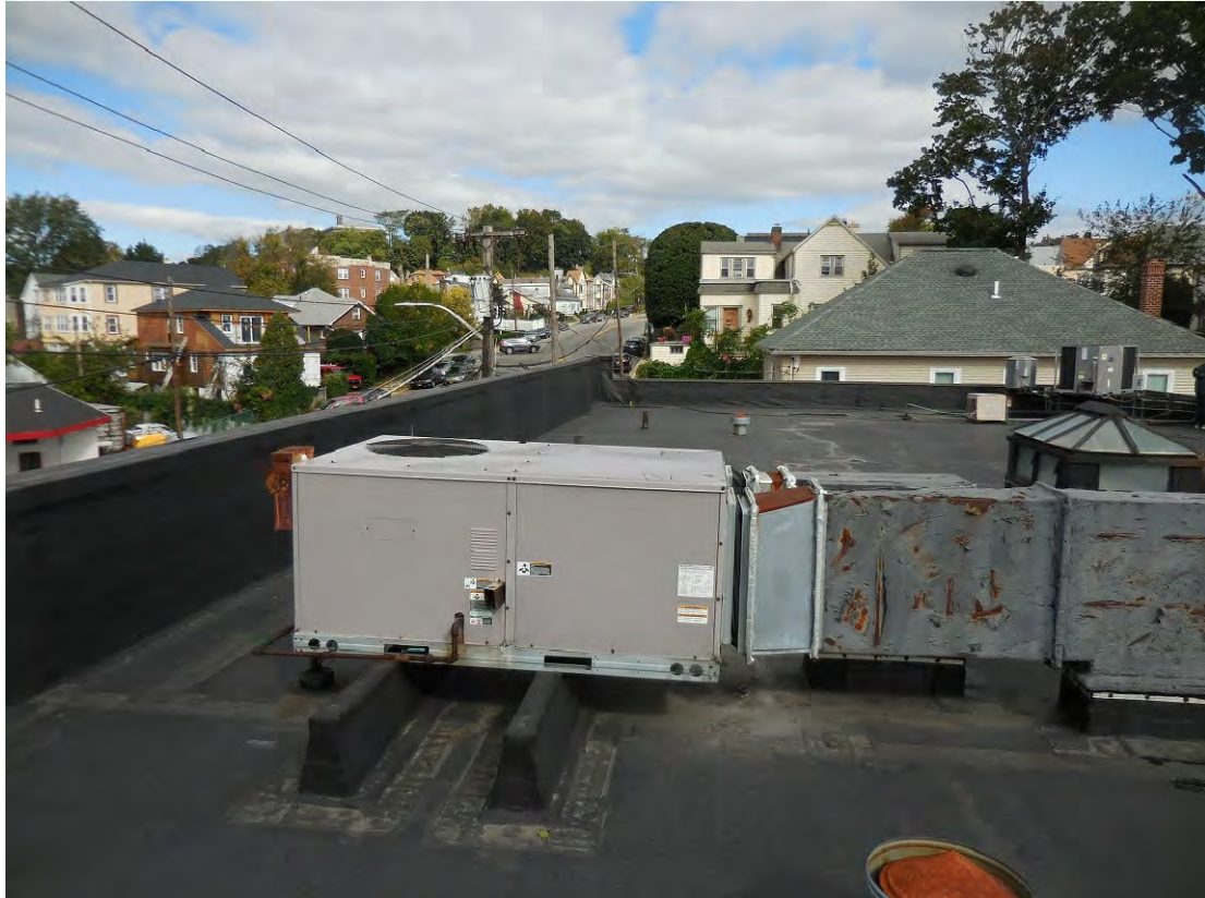
PHOTO No.11: MAIN ROOF-LOOKING NORTH. EXISTING EQUIPMENT CURBS TO BE REMOVED AND REPLACED WITH NEW INSULATED CORE CURBS. FLASH PER DETAIL 9/A-203.00.
