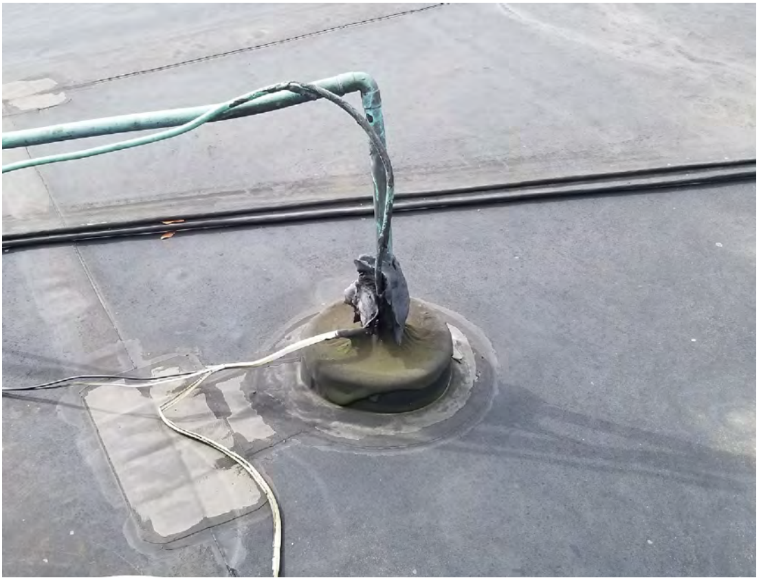
PHOTO No.14: PITCHPOCKET TO BE REMOVED. FLASH PENETRETION PER DETAIL 1/A-203.00.
