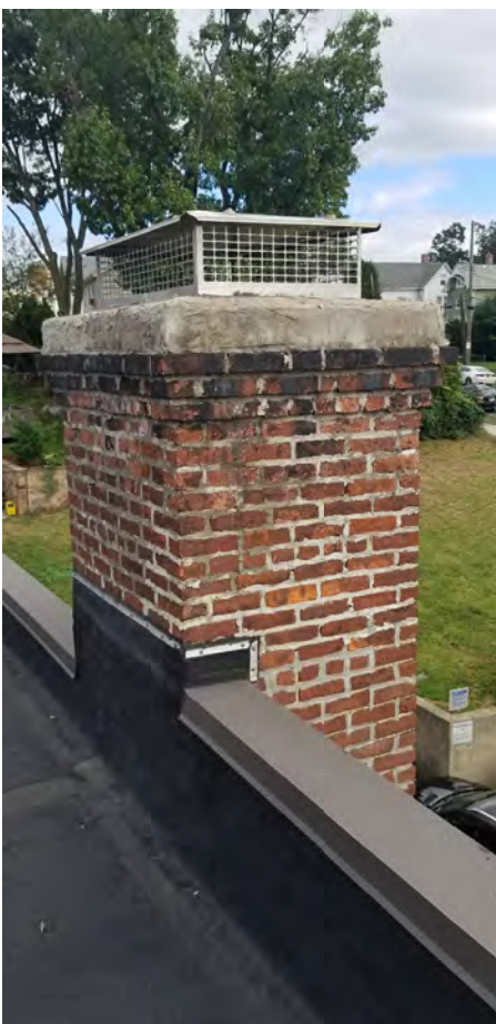
PHOTO No.8: EXISTING CHIMNEY TO REMAIN. PATCH CONCRETE TOP AS REQUIRED.
