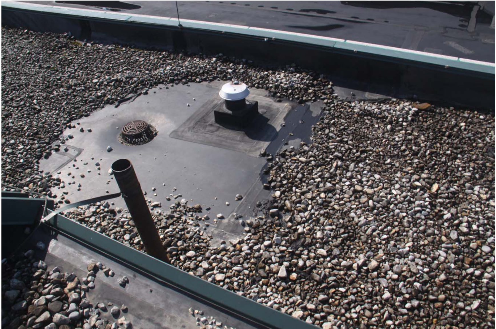
2219-00_19_0801 - ECs Roof [MP] (1043).JPG
