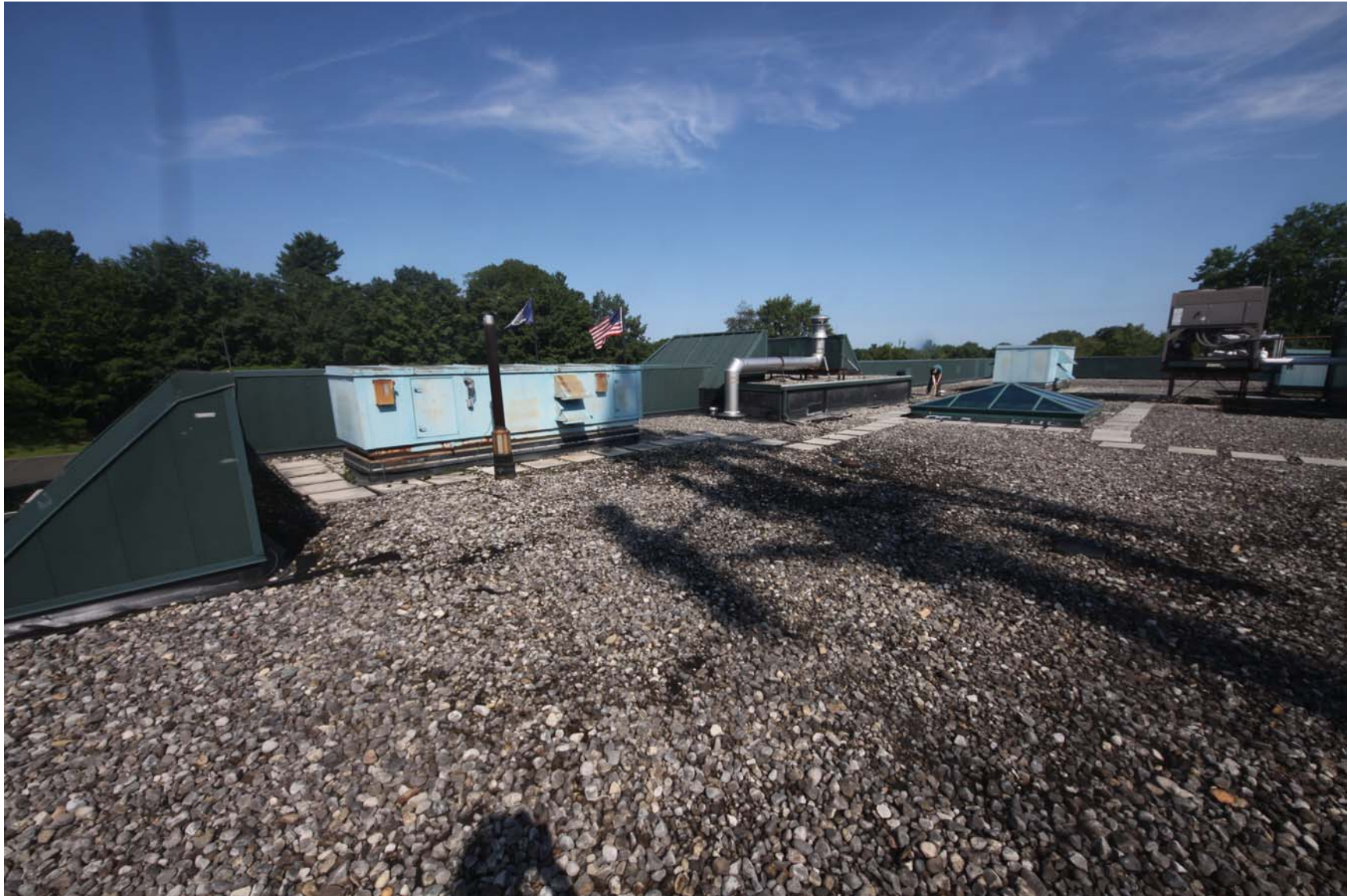
2219-00_19_0801 - ECs Roof [MP] (1177).JPG
