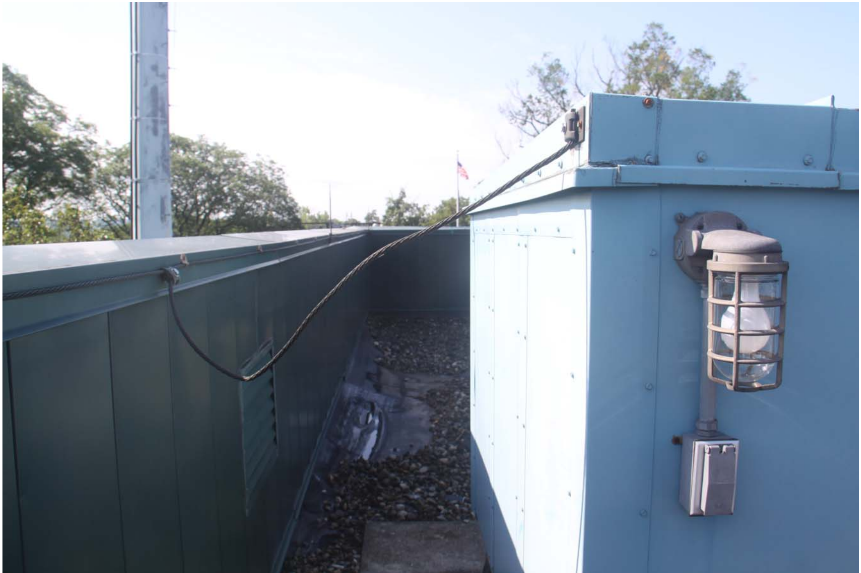
2219-00_19_0801 - ECs Roof [MP] (1033).JPG
