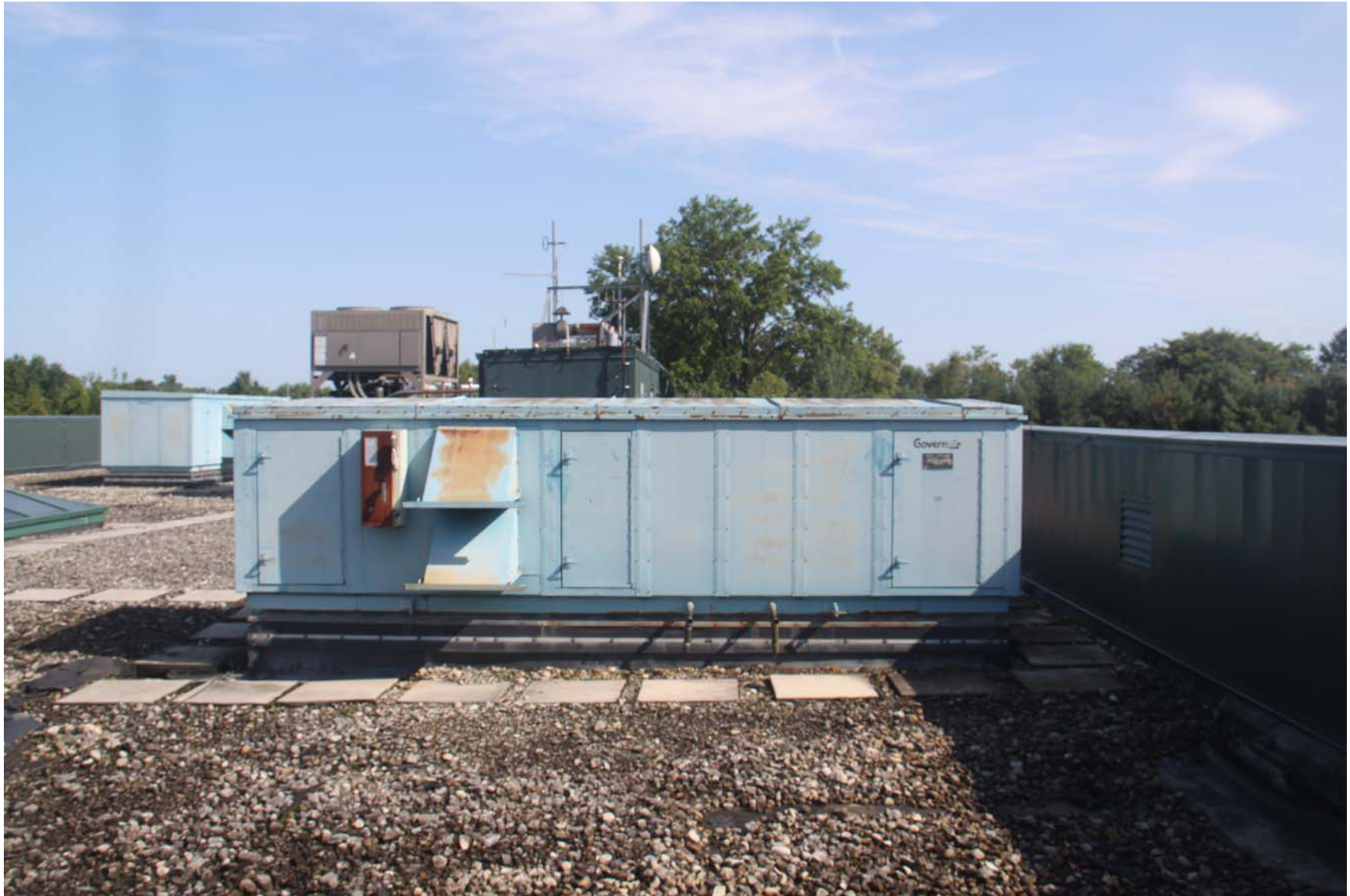
2219-00_19_0801 - ECs Roof [MP] (1040).JPG
