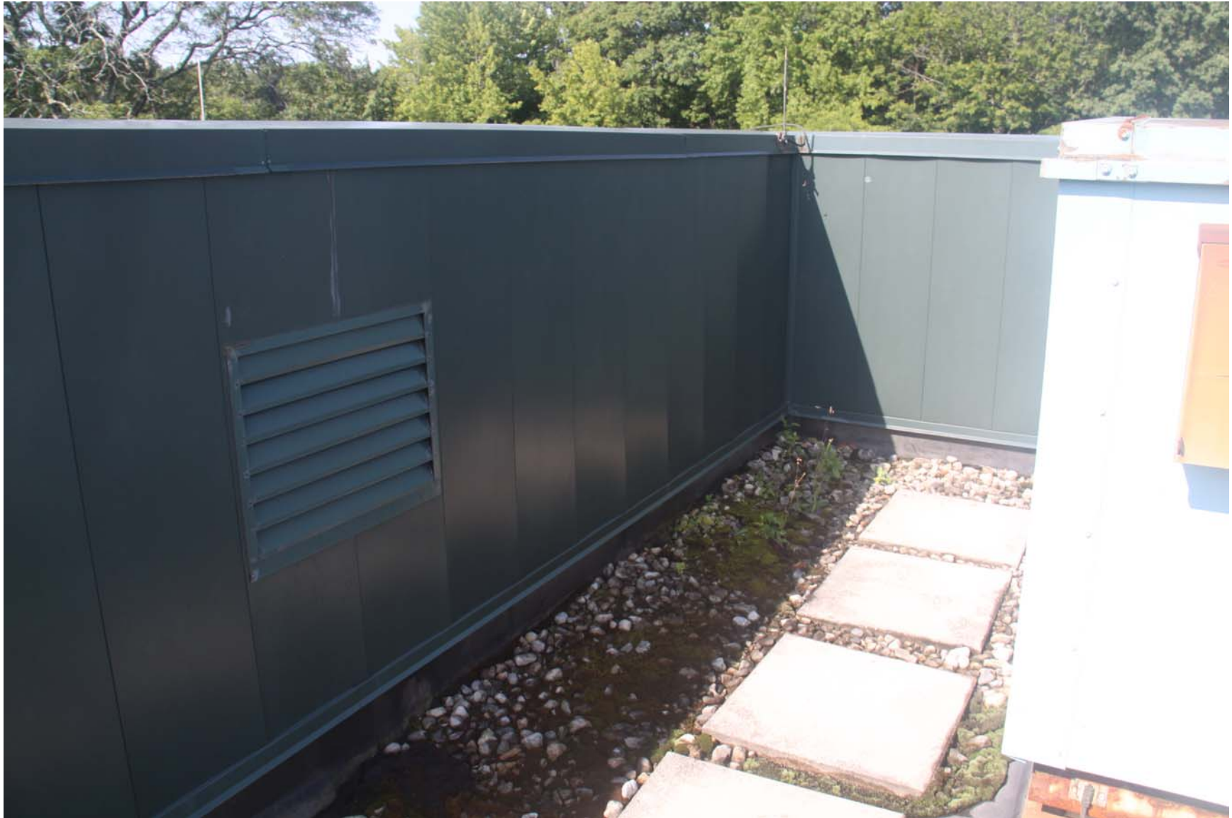
2219-00_19_0801 - ECs Roof [MP] (1085).JPG
