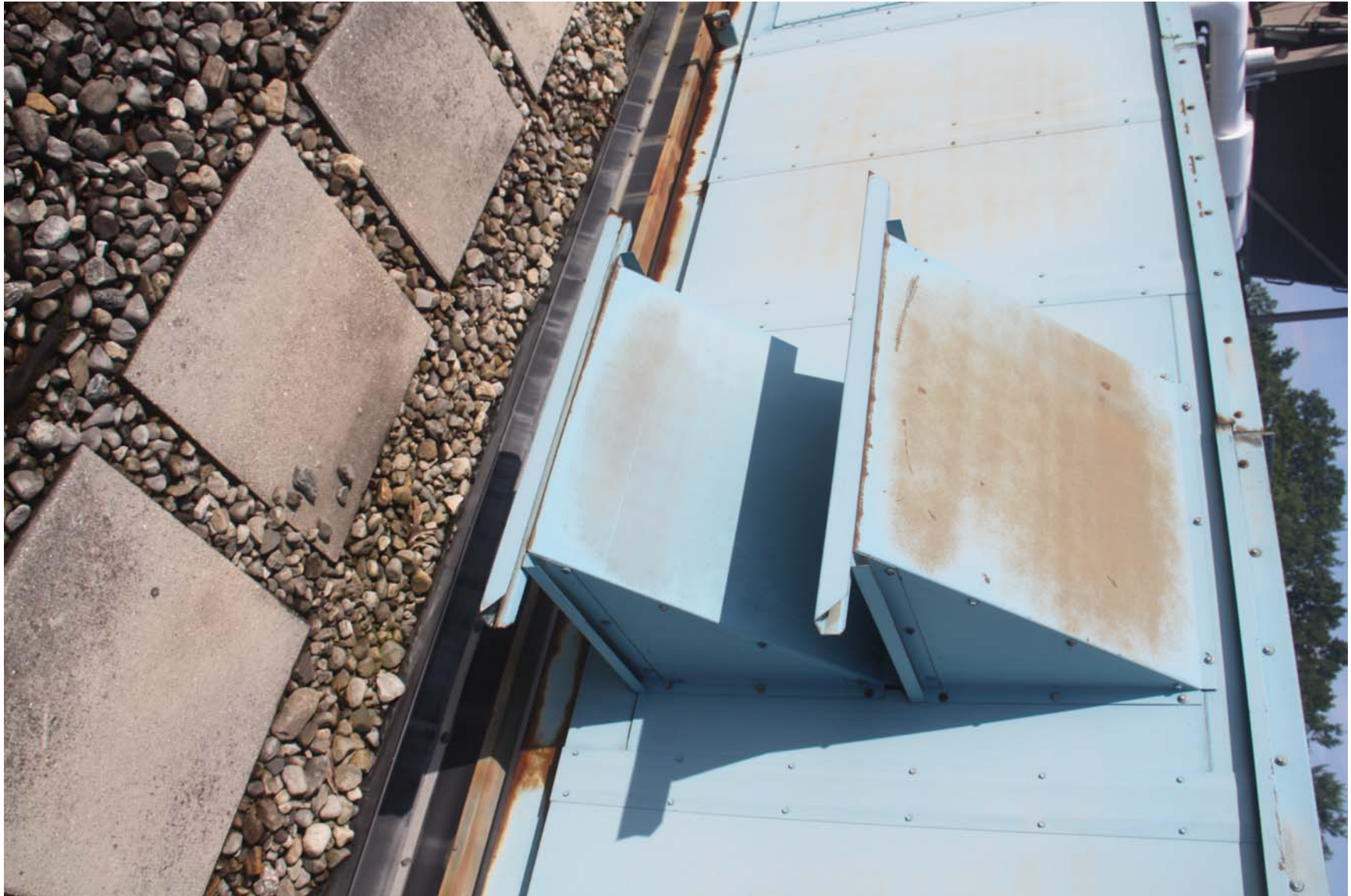
2219-00_19_0801 - ECs Roof [MP] (1016).JPG
