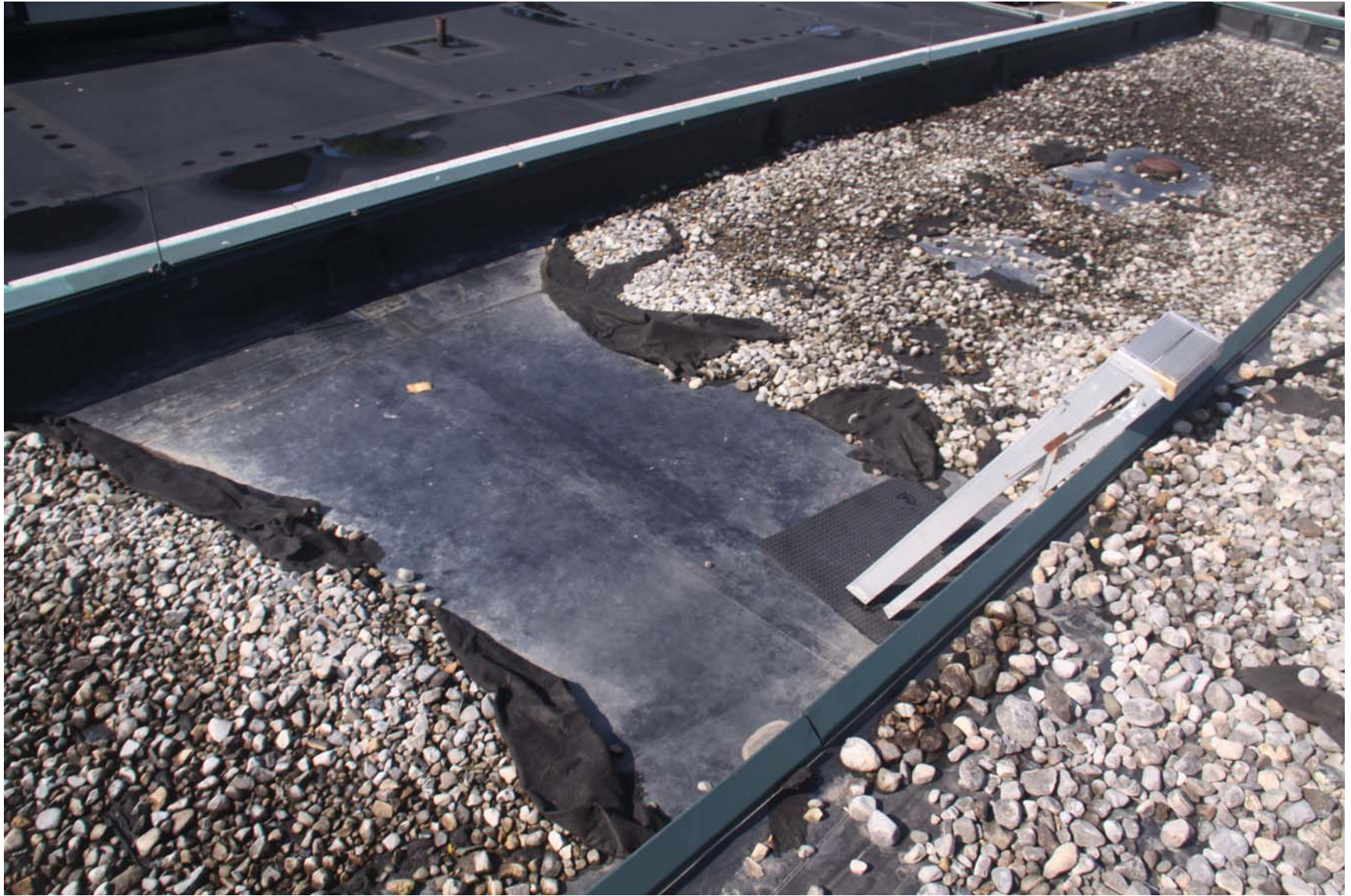
2219-00_19_0801 - ECs Roof [MP] (1045).JPG
