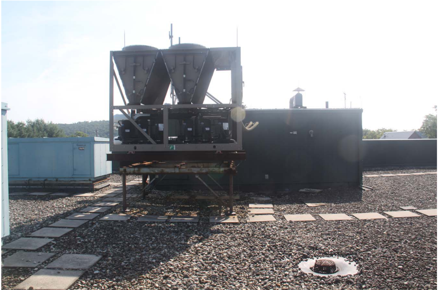
2219-00_19_0801 - ECs Roof [MP] (1117).JPG
