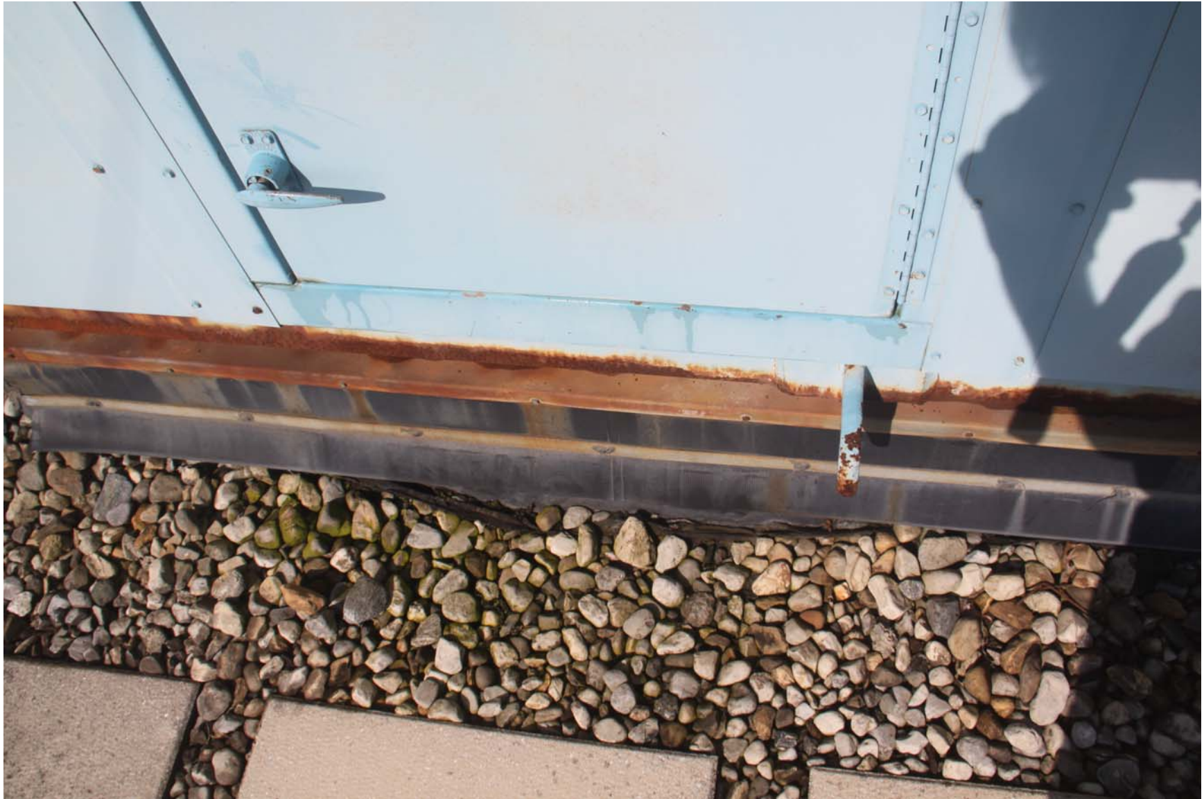
2219-00_19_0801 - ECs Roof [MP] (1018).JPG
