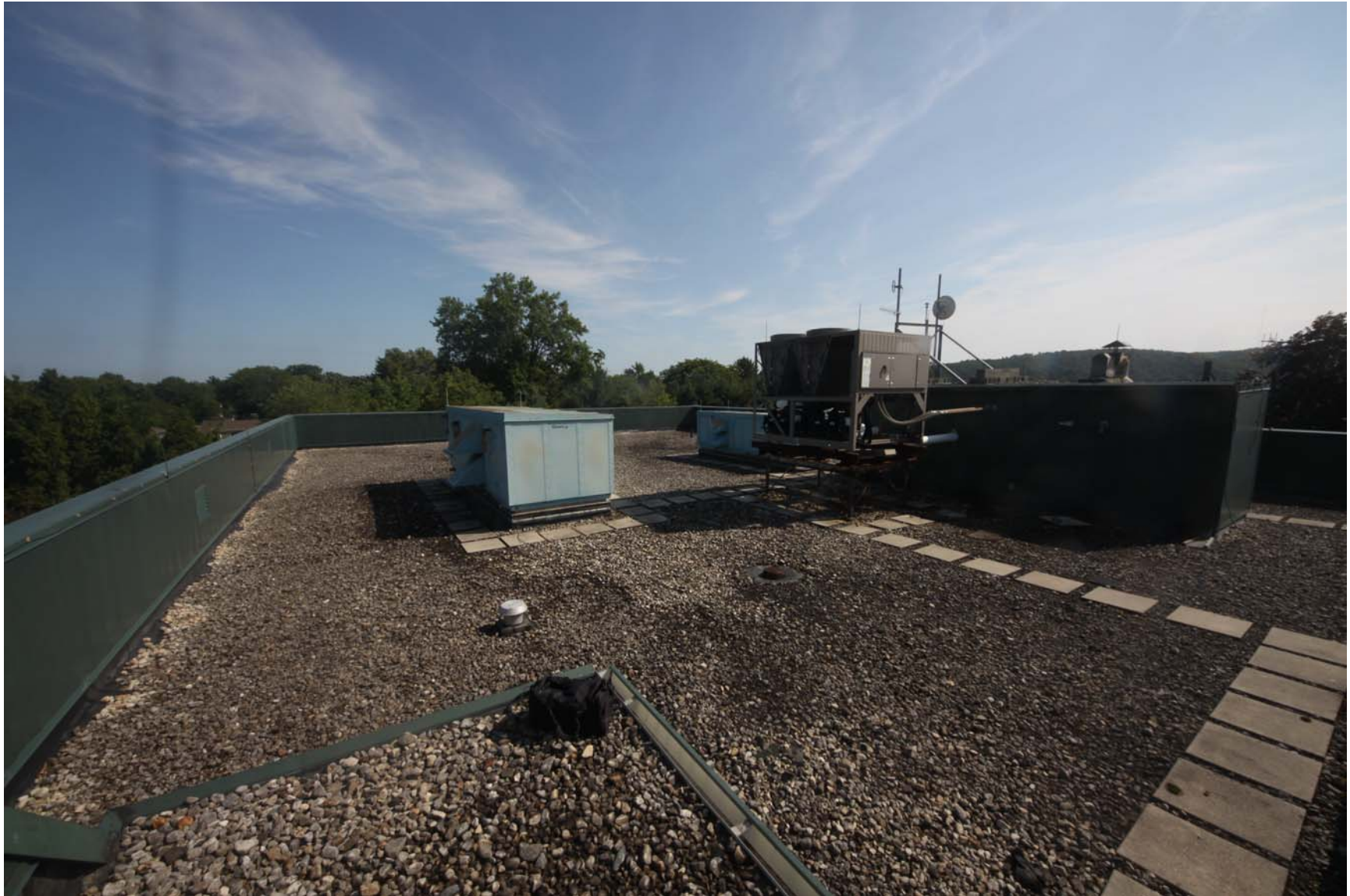
2219-00_19_0801 - ECs Roof [MP] (1160).JPG
