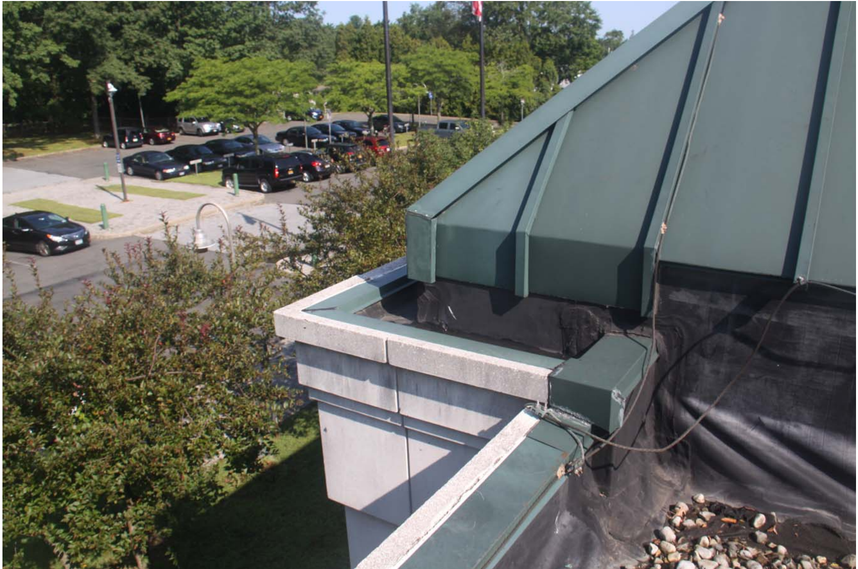
2219-00_19_0801 - ECs Roof [MP] (1064).JPG
