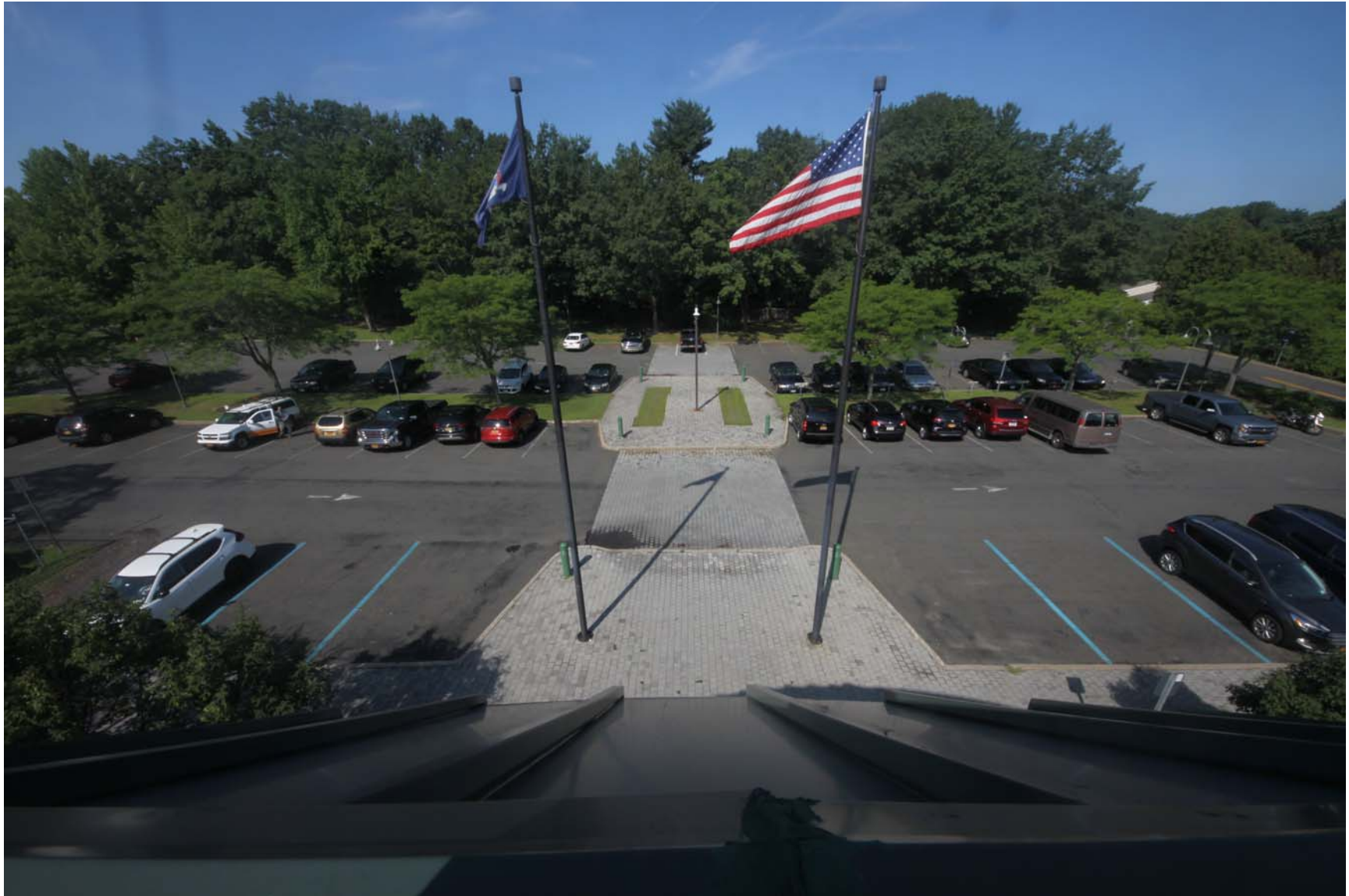
2219-00_19_0801 - ECs Roof [MP] (1156).JPG
