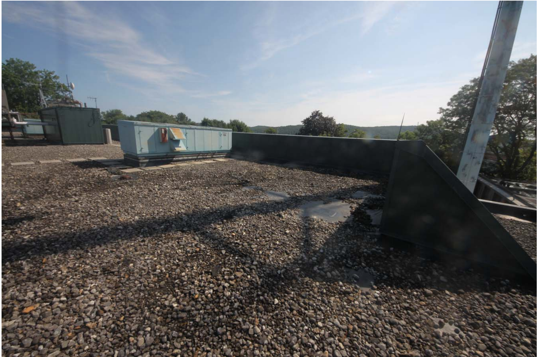
2219-00_19_0801 - ECs Roof [MP] (1178).JPG
