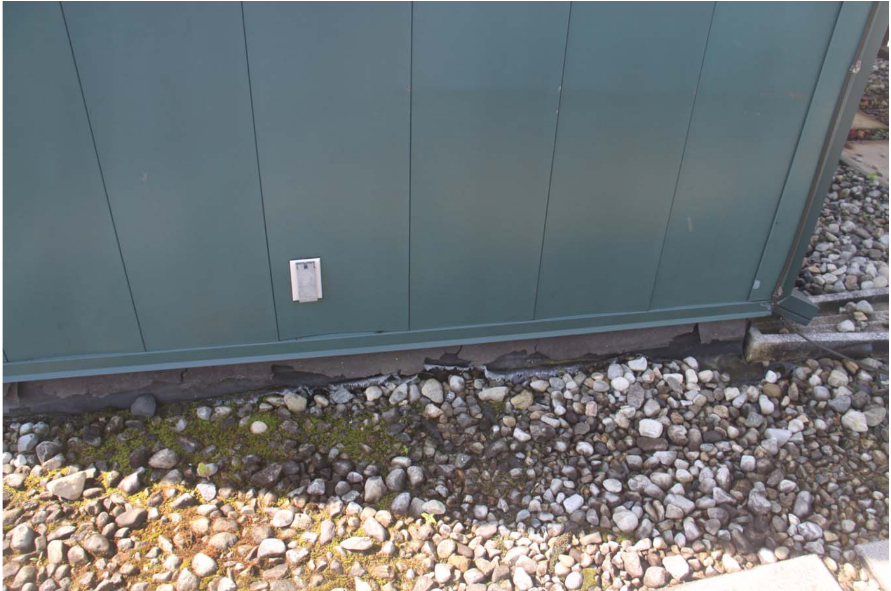
2219-00_19_0801 - ECs Roof [MP] (1019).JPG
