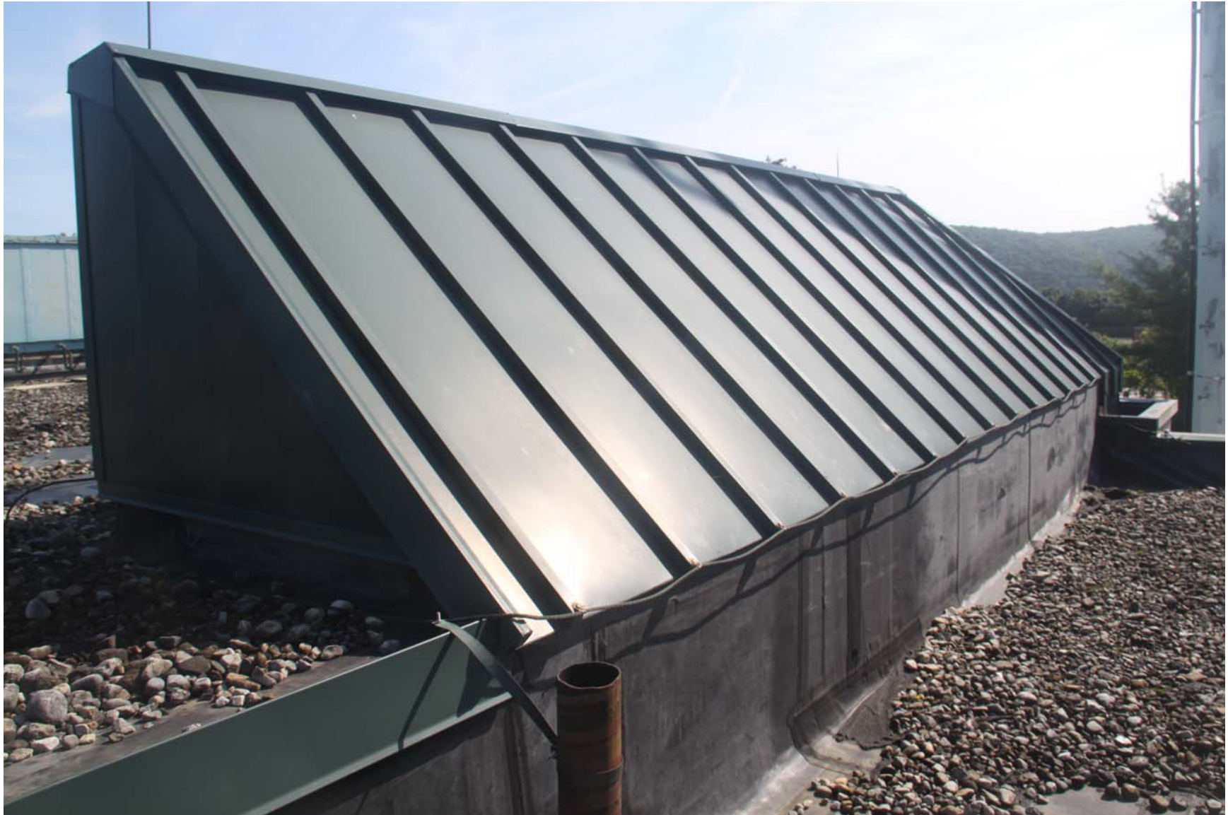
2219-00_19_0801 - ECs Roof [MP] (1074).JPG
