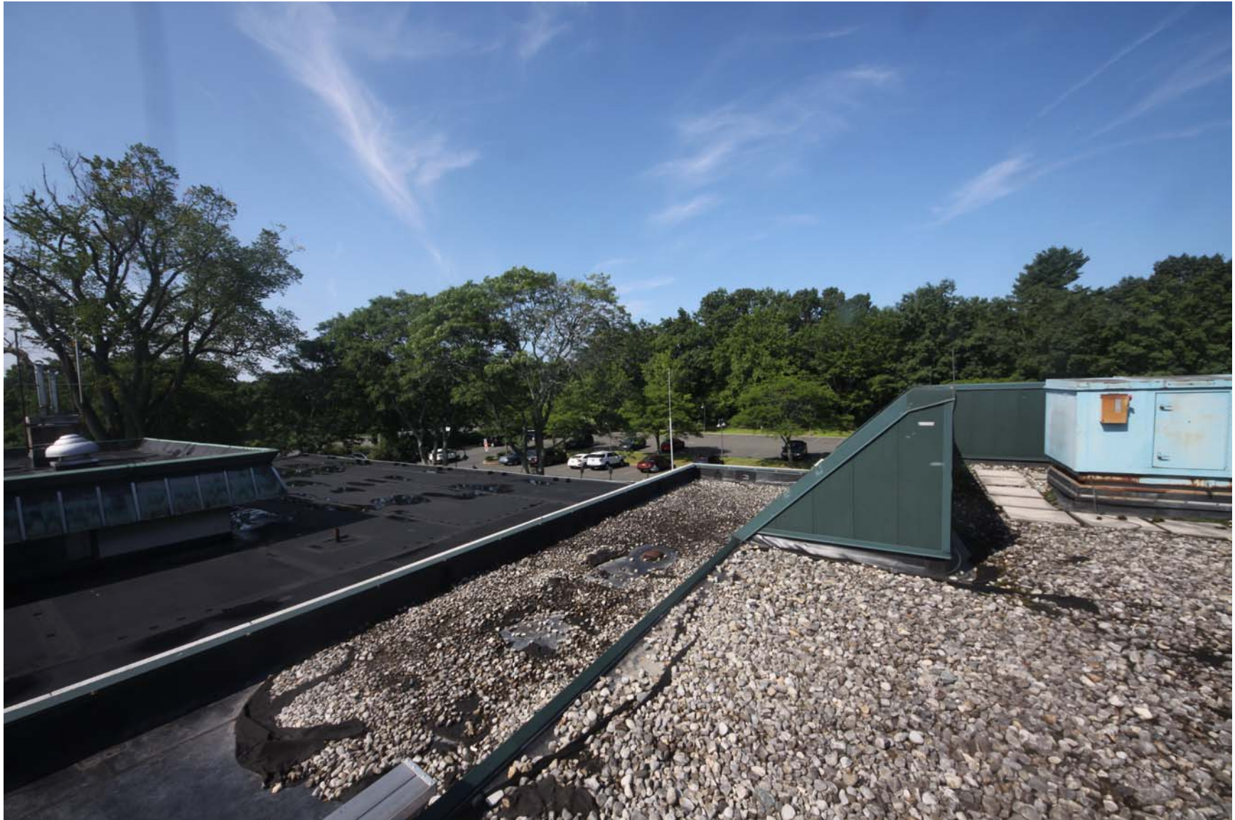
2219-00_19_0801 - ECs Roof [MP] (1179).JPG
