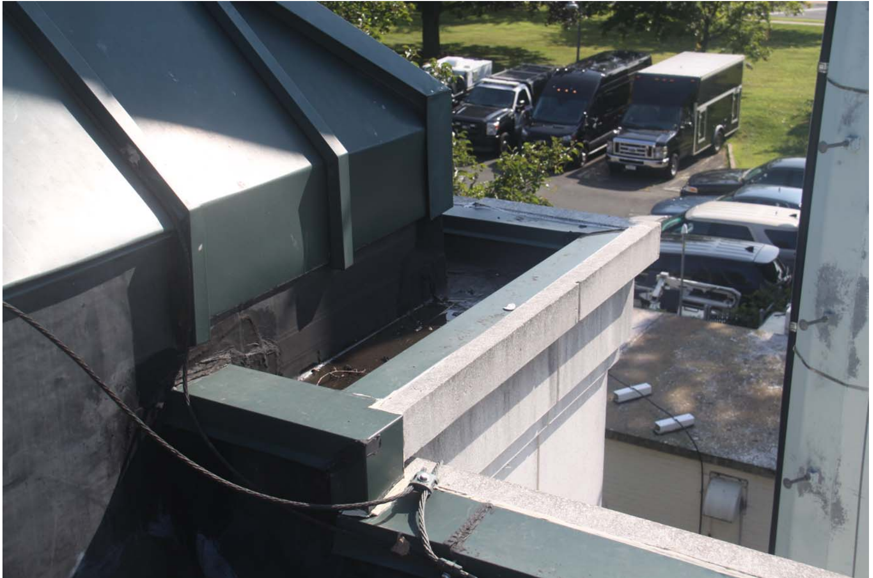
2219-00_19_0801 - ECs Roof [MP] (1080).JPG
