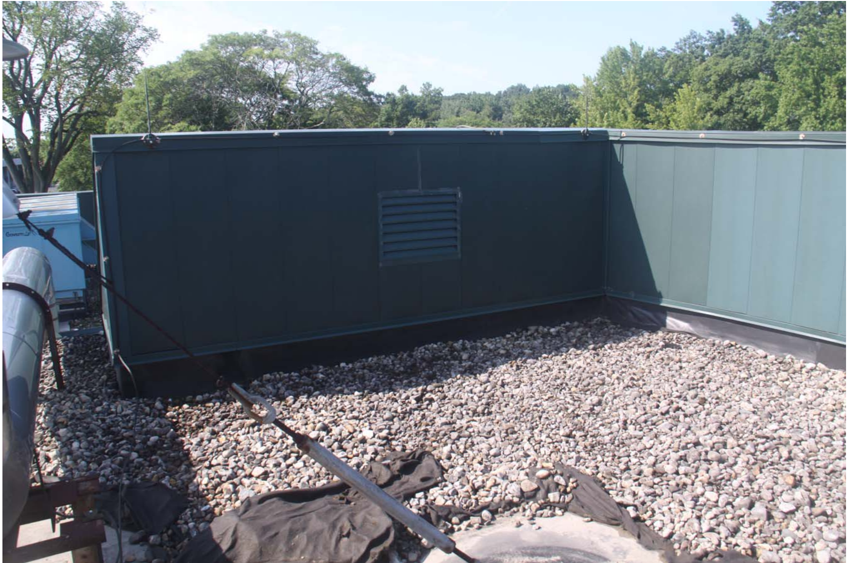
2219-00_19_0801 - ECs Roof [MP] (1135).JPG
