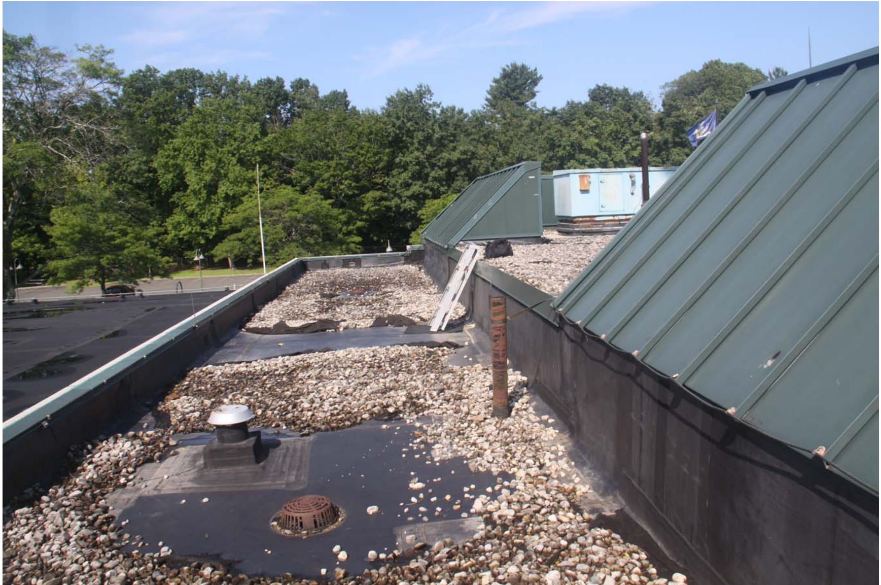
2219-00_19_0801 - ECs Roof [MP] (1079).JPG
