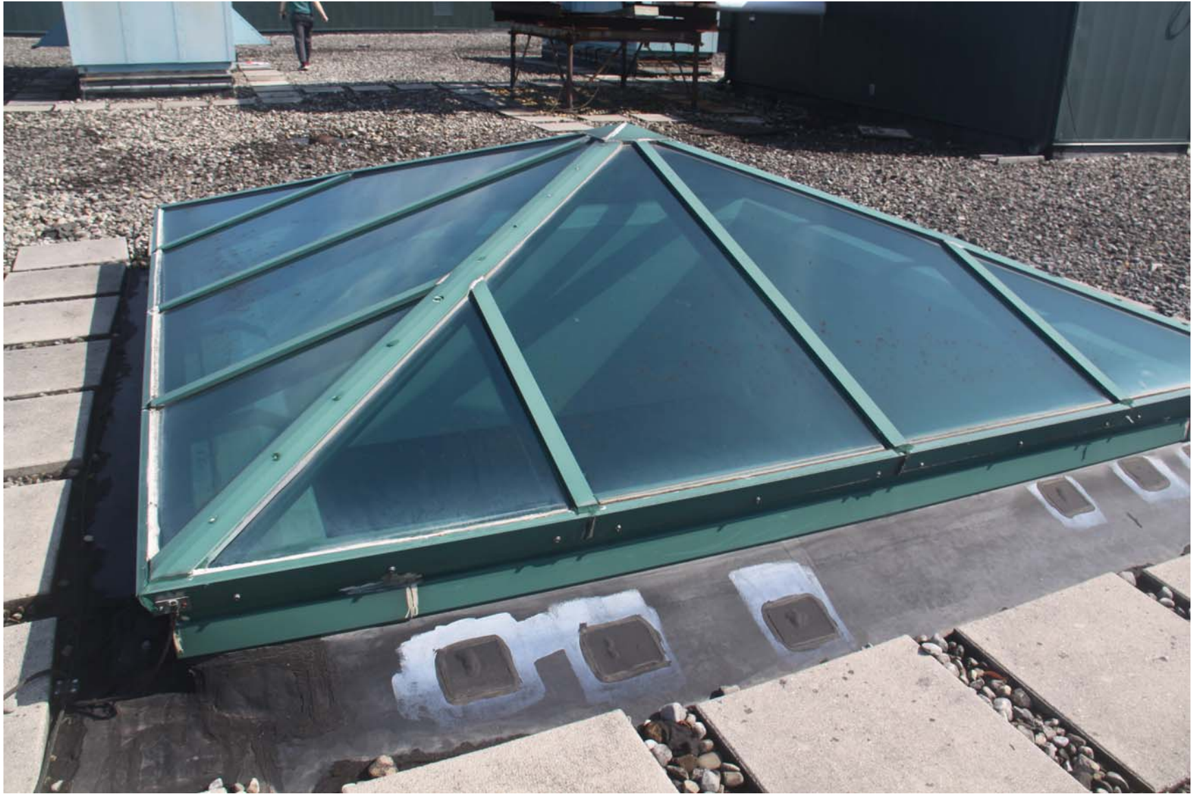
2219-00_19_0801 - ECs Roof [MP] (1101).JPG
