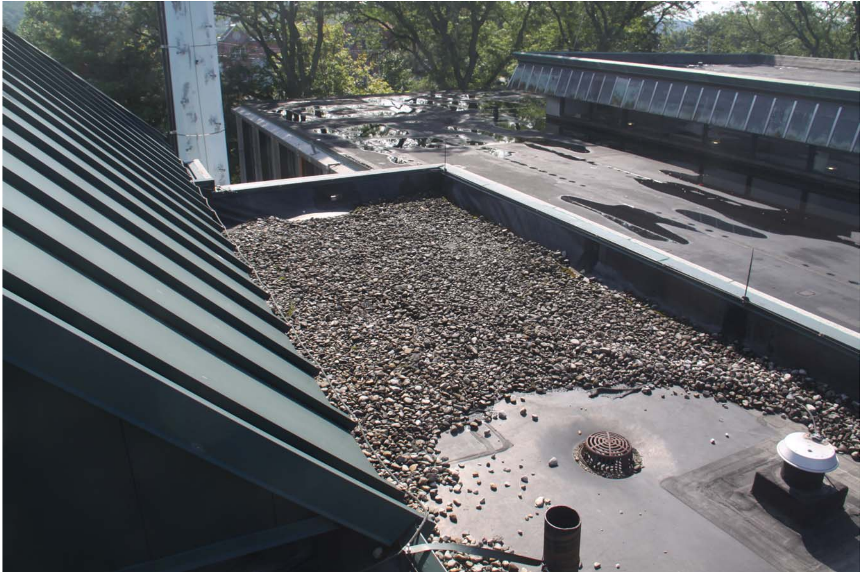
2219-00_19_0801 - ECs Roof [MP] (1042).JPG
