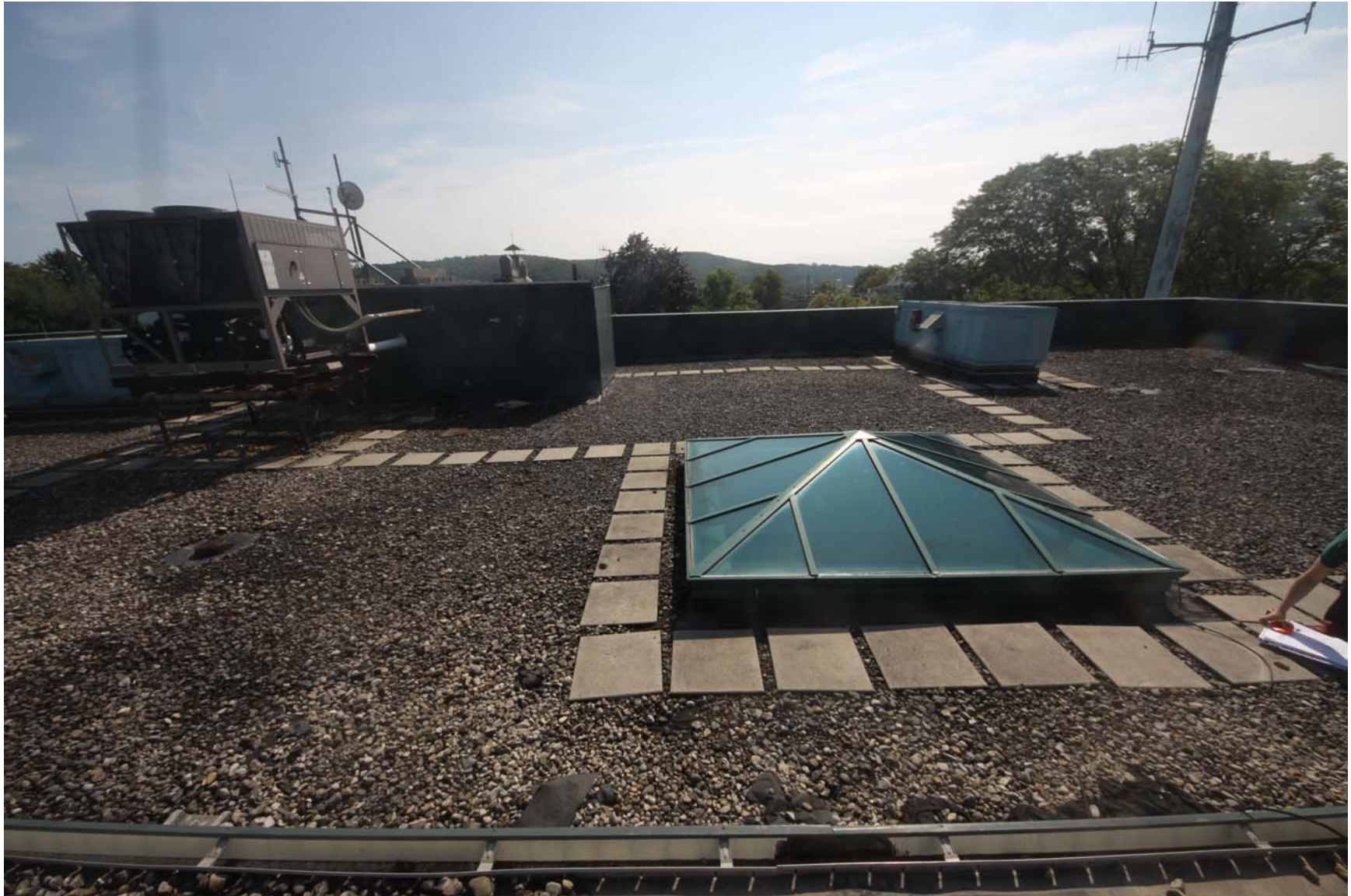
2219-00_19_0801 - ECs Roof [MP] (1161).JPG
