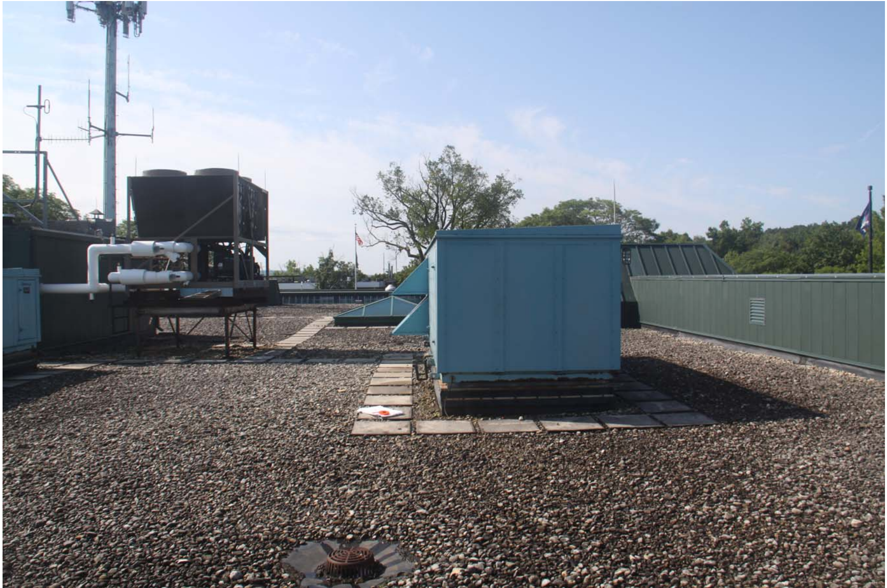
2219-00_19_0801 - ECs Roof [MP] (1127).JPG
