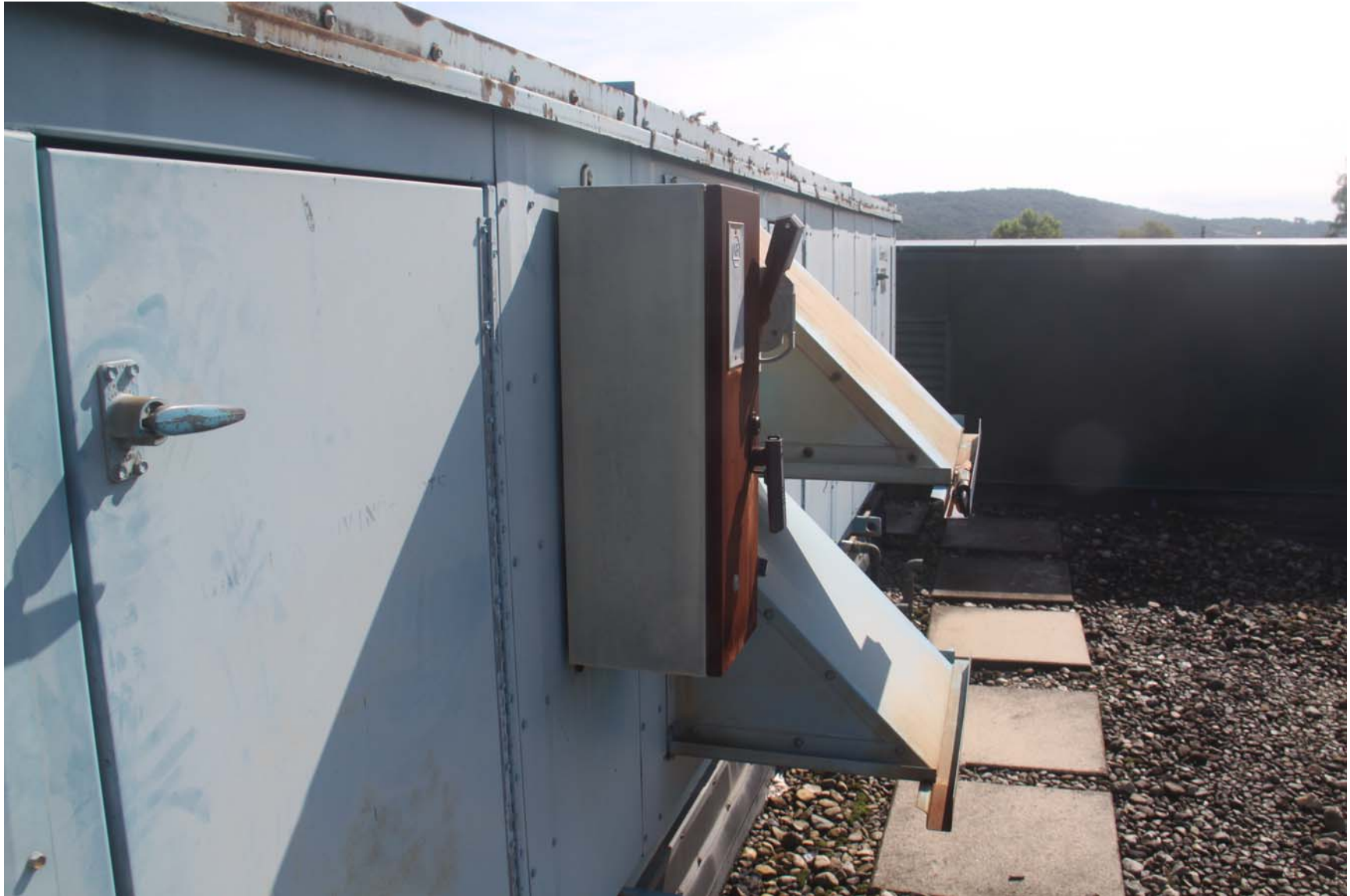
2219-00_19_0801 - ECs Roof [MP] (1036).JPG
