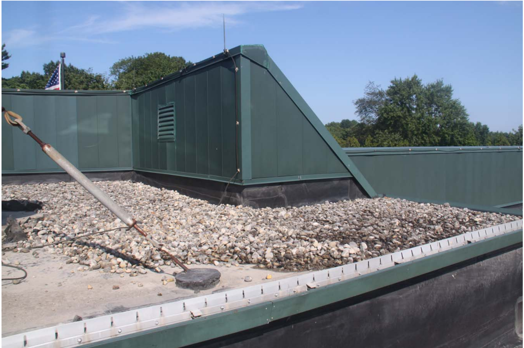
2219-00_19_0801 - ECs Roof [MP] (1106).JPG
