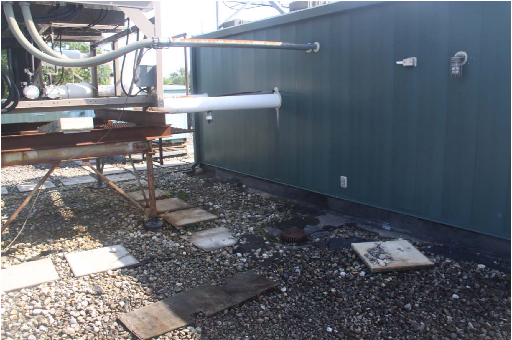
2219-00_19_0801 - ECs Roof [MP] (1111).JPG
