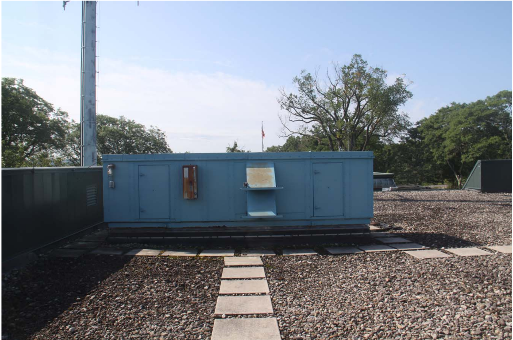
2219-00_19_0801 - ECs Roof [MP] (1028).JPG
