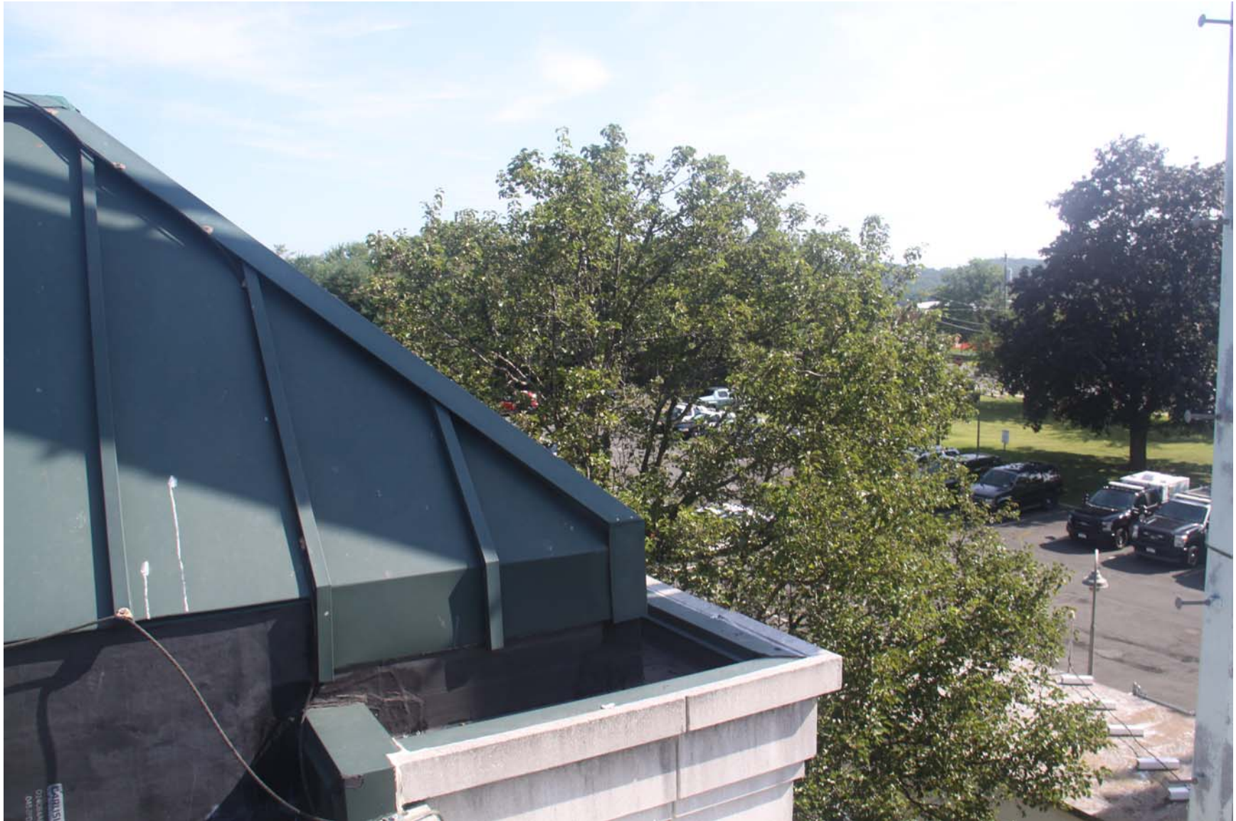
2219-00_19_0801 - ECs Roof [MP] (1075).JPG
