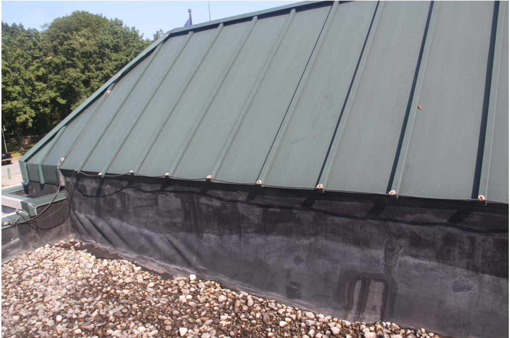
2219-00_19_0801 - ECs Roof [MP] (1066).JPG
