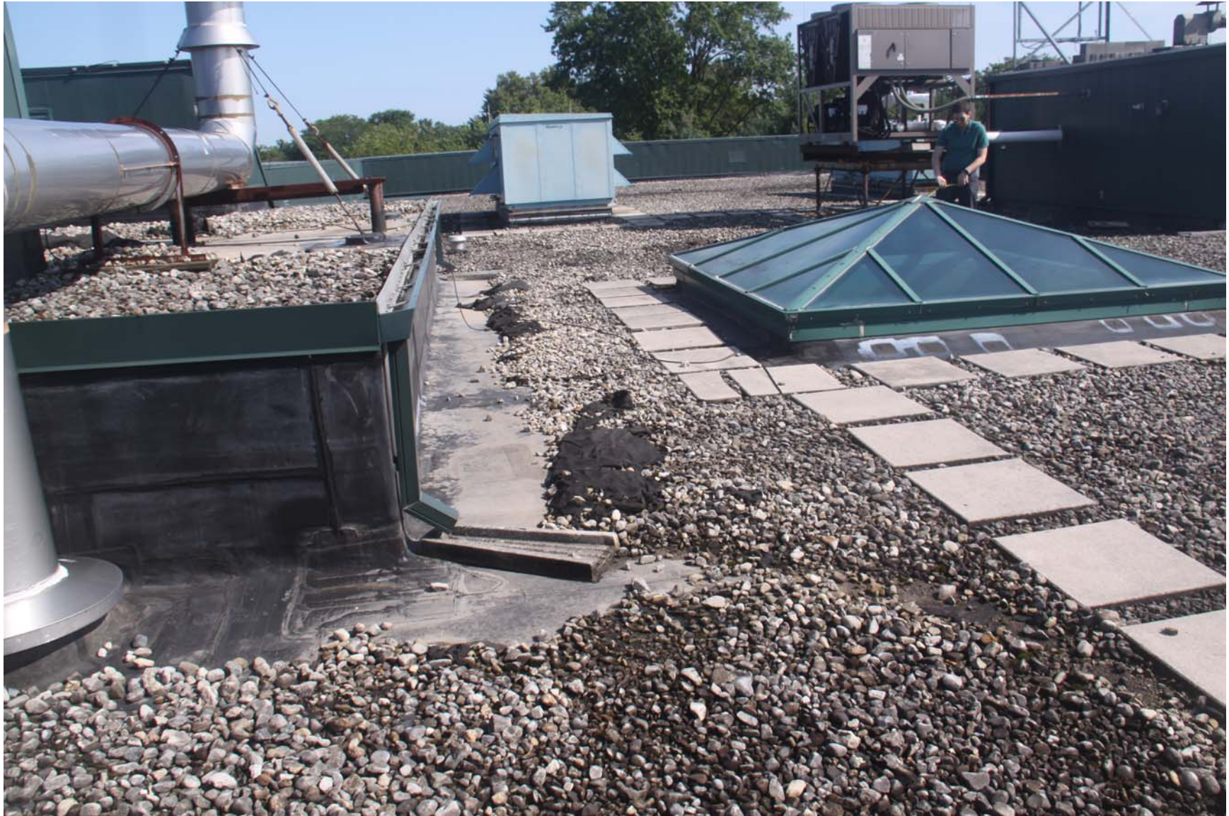
2219-00_19_0801 - ECs Roof [MP] (1097).JPG
