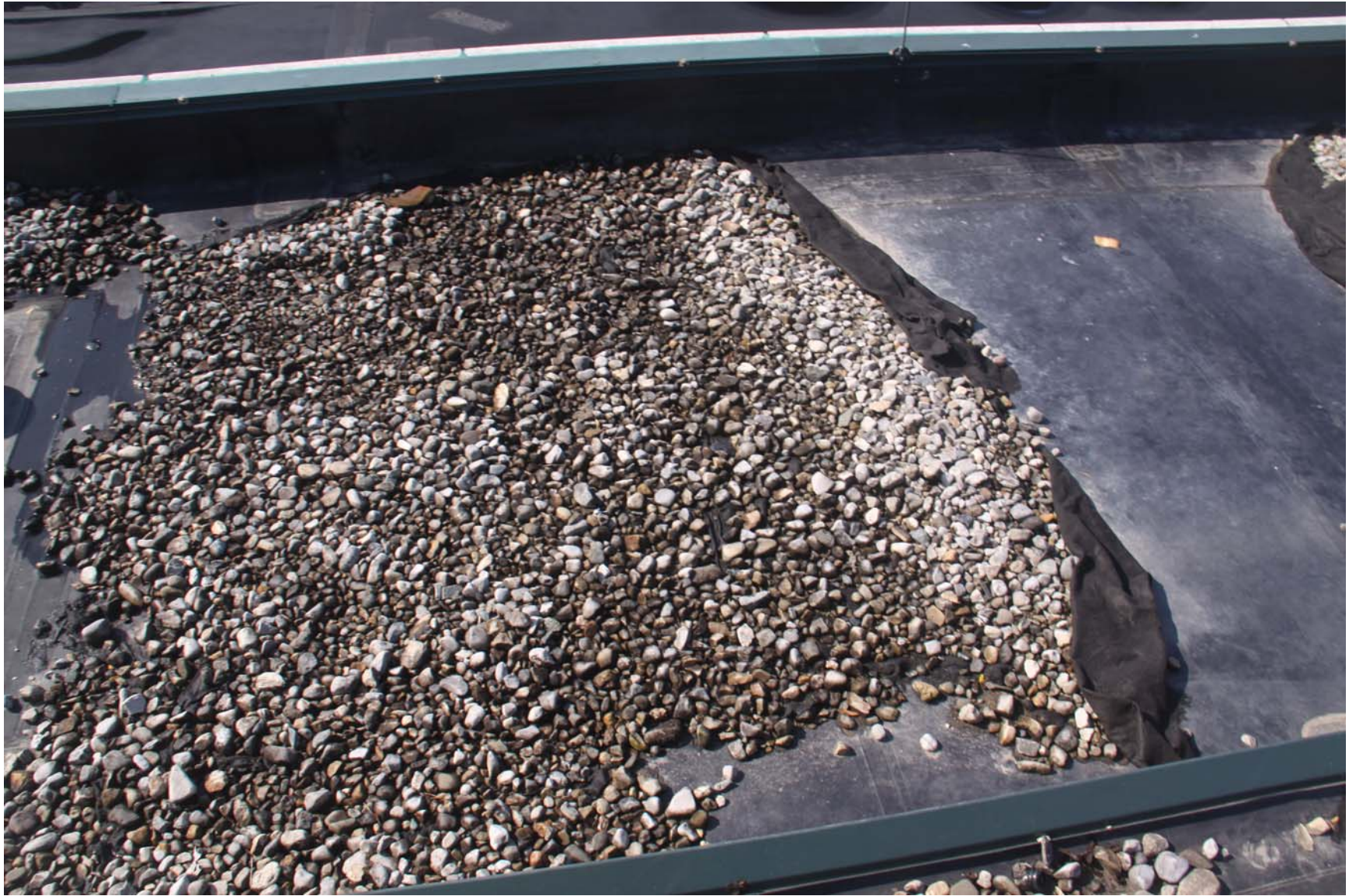
2219-00_19_0801 - ECs Roof [MP] (1044).JPG
