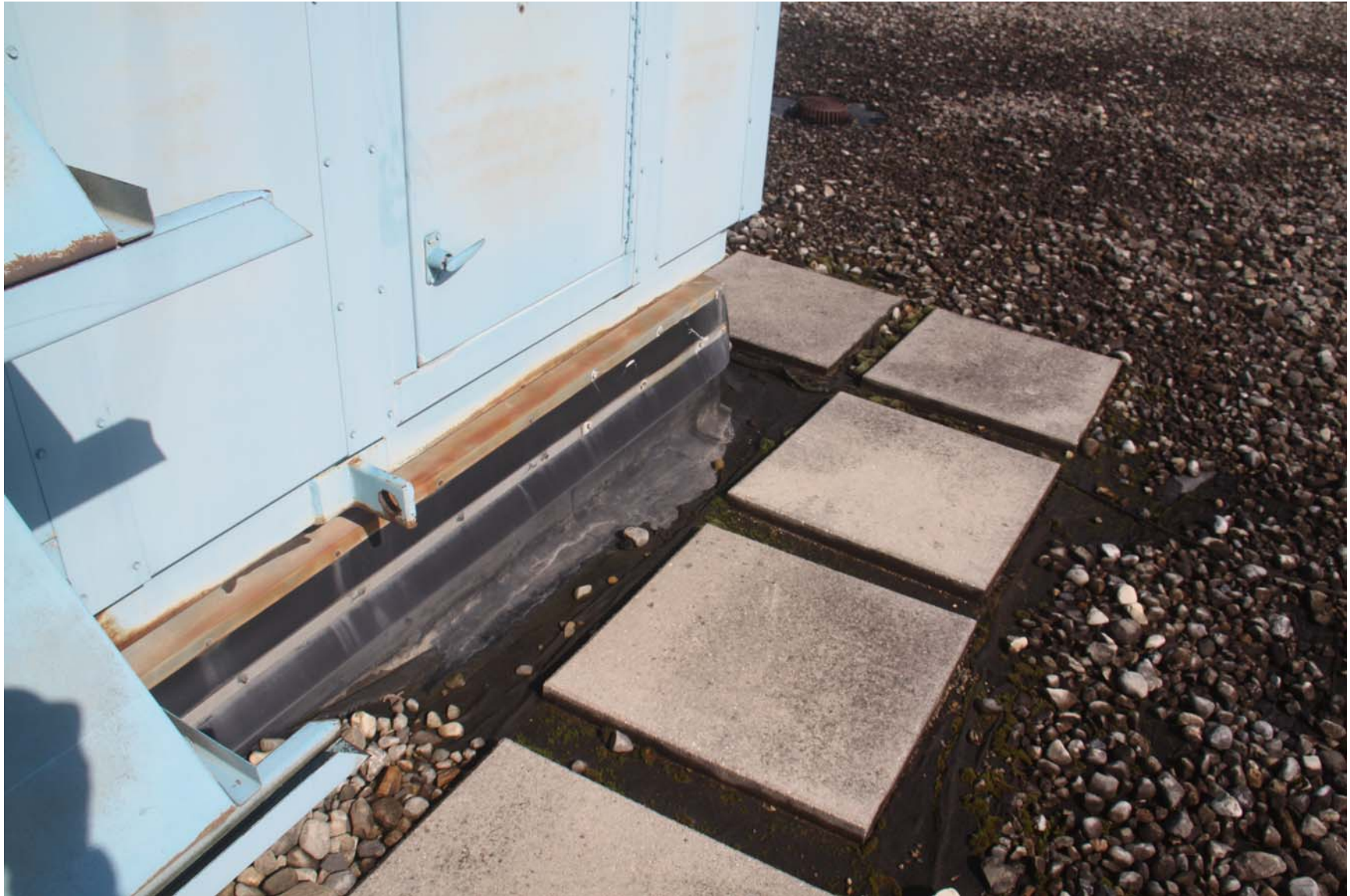
2219-00_19_0801 - ECs Roof [MP] (1017).JPG
