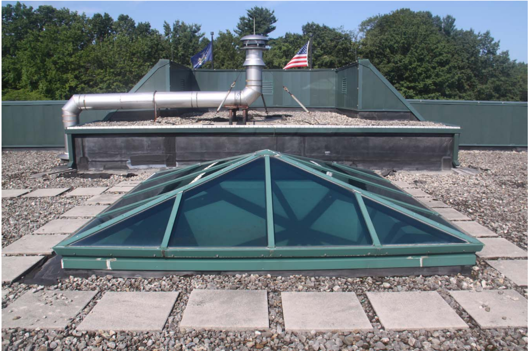
2219-00_19_0801 - ECs Roof [MP] (1113).JPG
