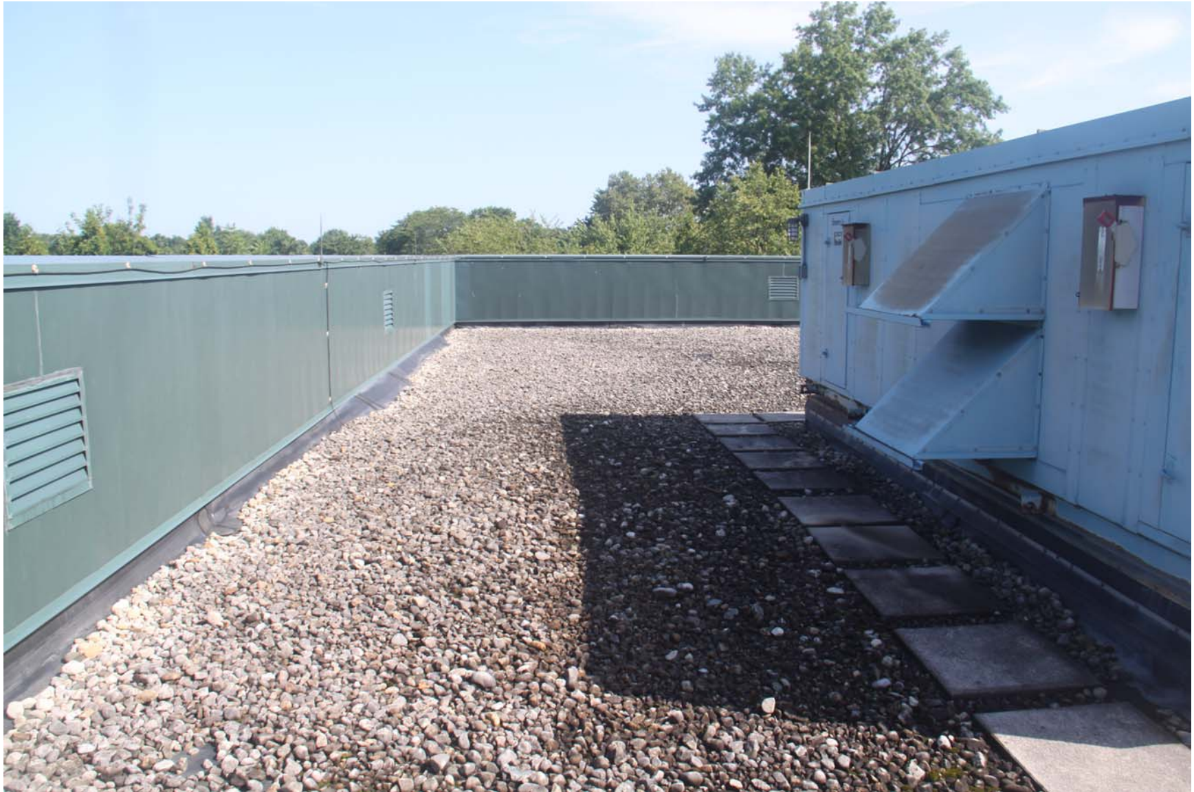
2219-00_19_0801 - ECs Roof [MP] (1119).JPG
