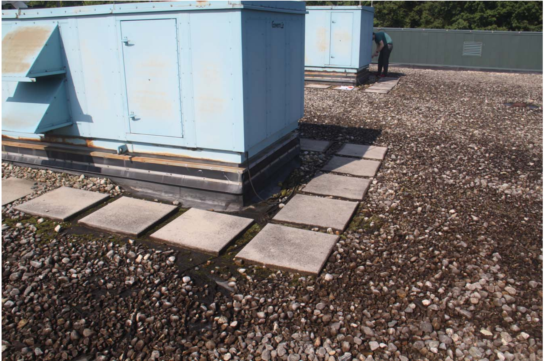
2219-00_19_0801 - ECs Roof [MP] (1014).JPG
