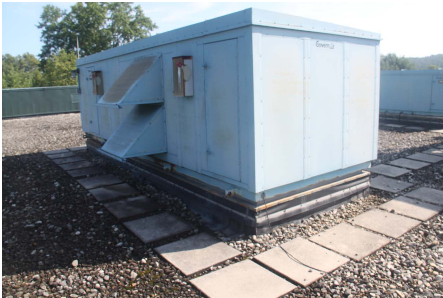
2219-00_19_0801 - ECs Roof [MP] (1118).JPG
