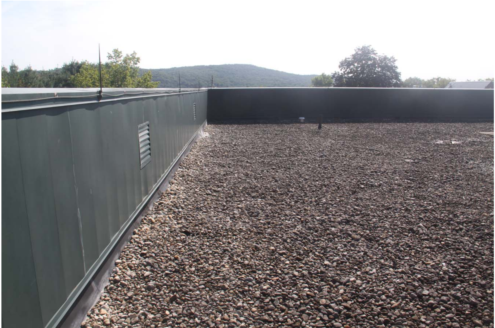
2219-00_19_0801 - ECs Roof [MP] (1123).JPG
