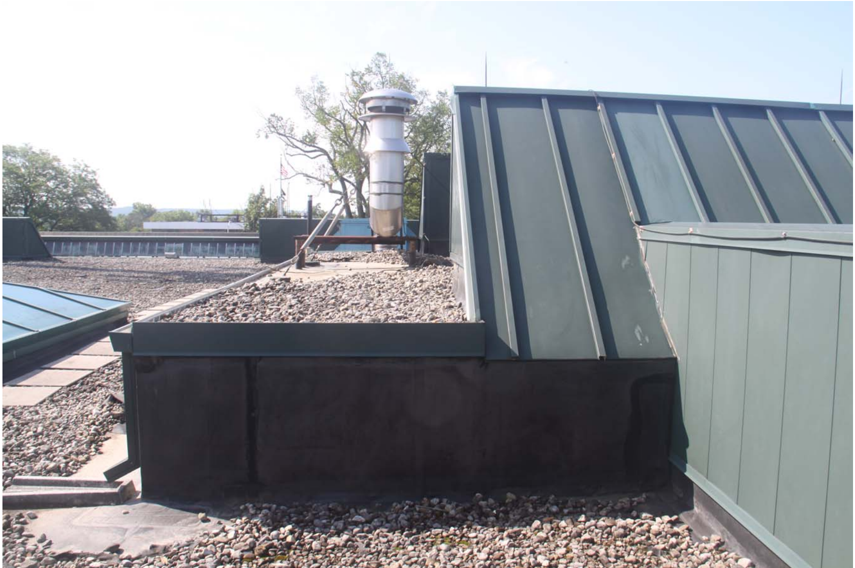
2219-00_19_0801 - ECs Roof [MP] (1120).JPG
