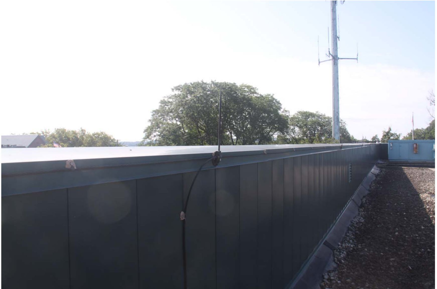
2219-00_19_0801 - ECs Roof [MP] (1013).JPG
