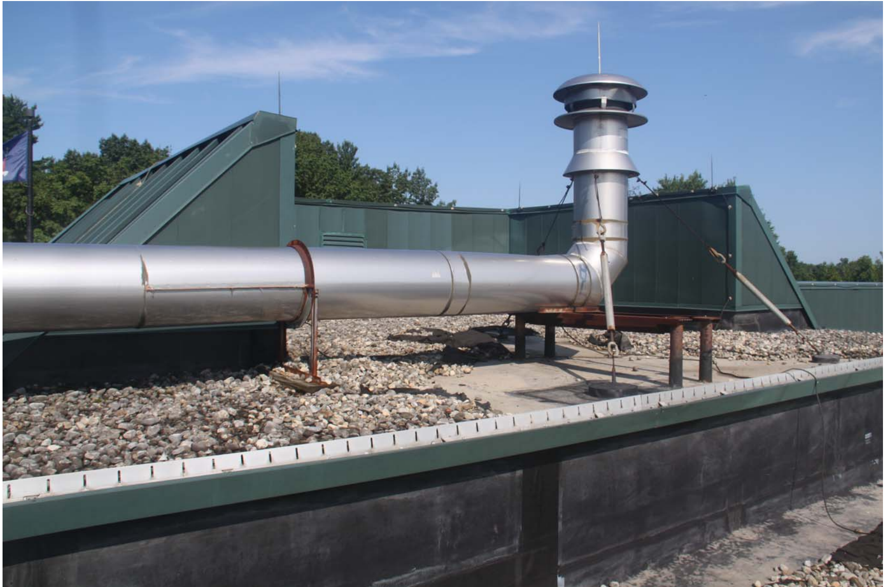
2219-00_19_0801 - ECs Roof [MP] (1100).JPG
