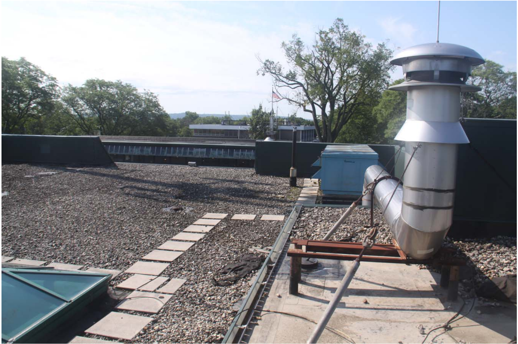
2219-00_19_0801 - ECs Roof [MP] (1147).JPG
