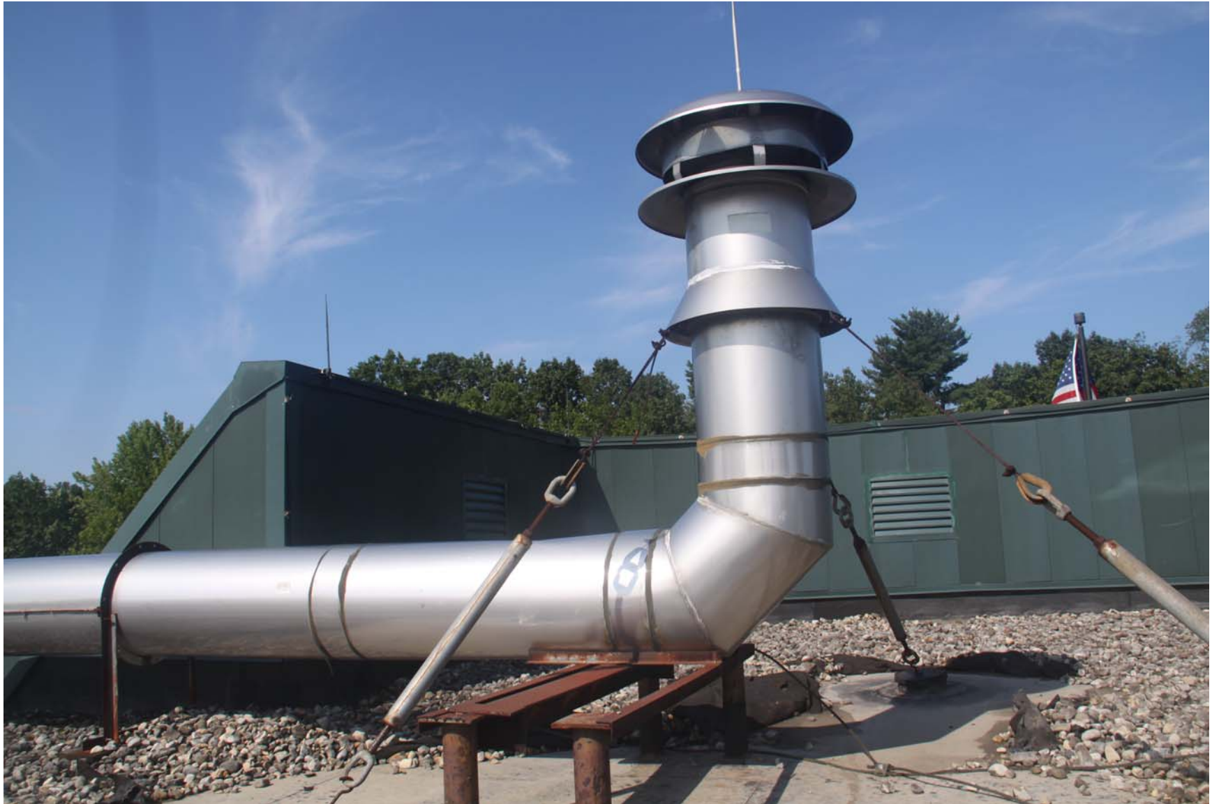
2219-00_19_0801 - ECs Roof [MP] (1105).JPG
