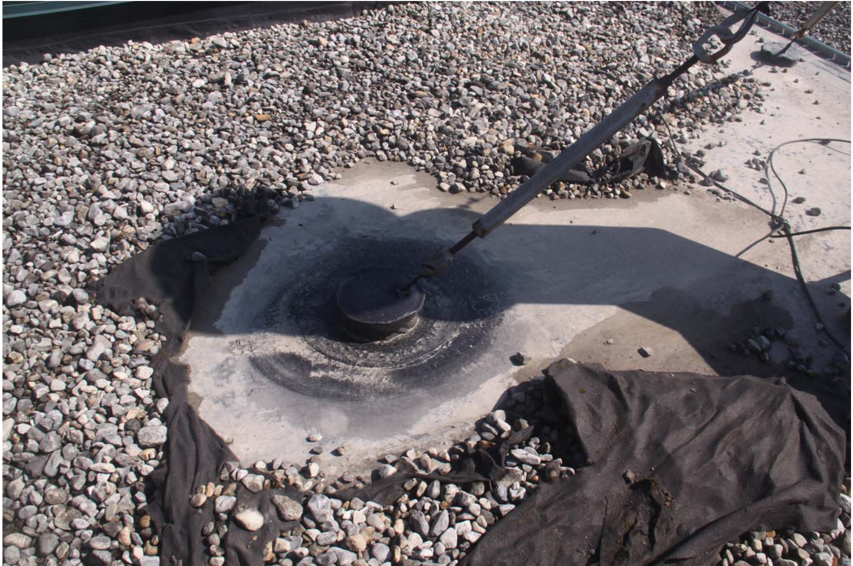
2219-00_19_0801 - ECs Roof [MP] (1136).JPG
