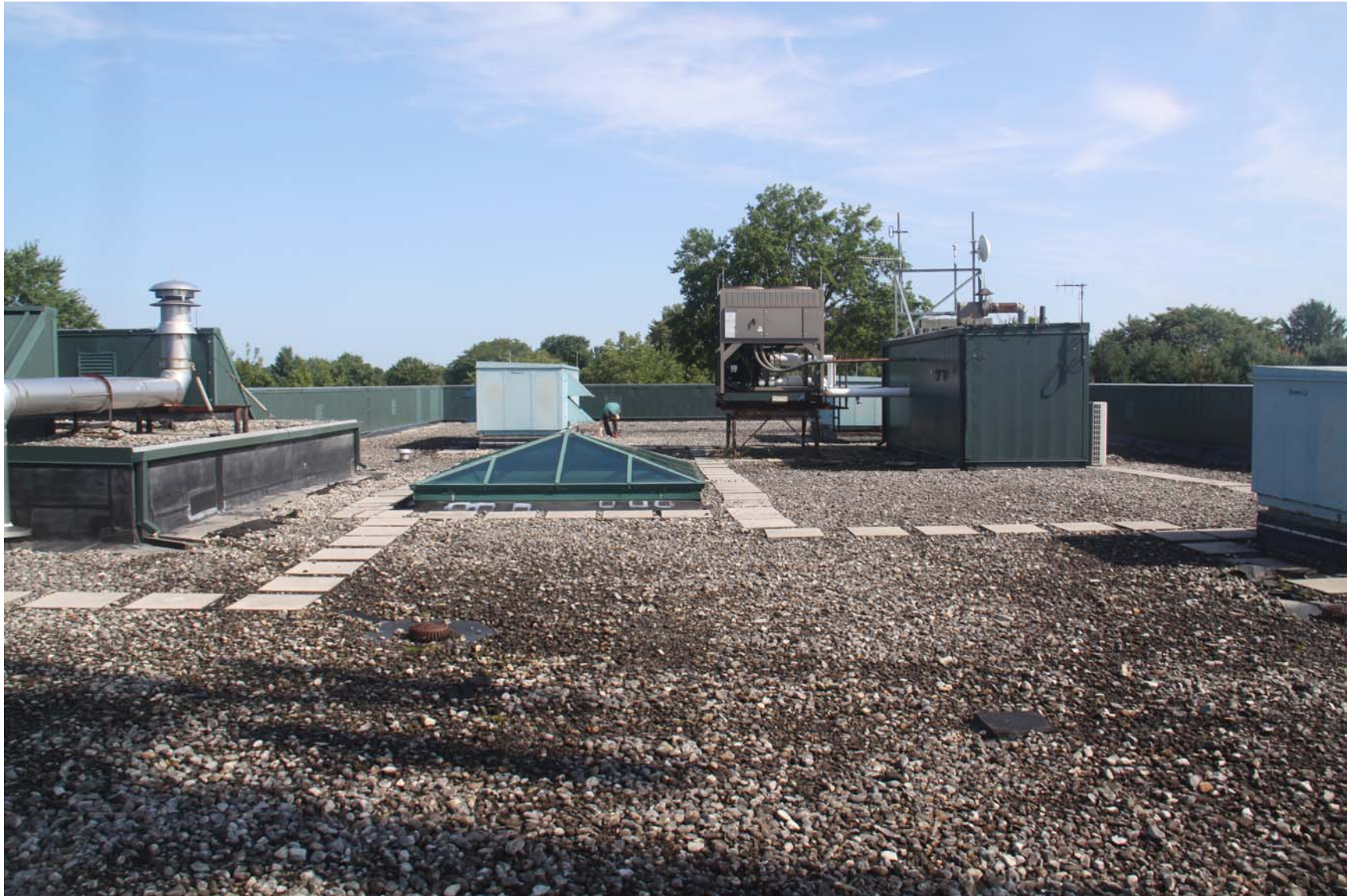
2219-00_19_0801 - ECs Roof [MP] (1049).JPG
