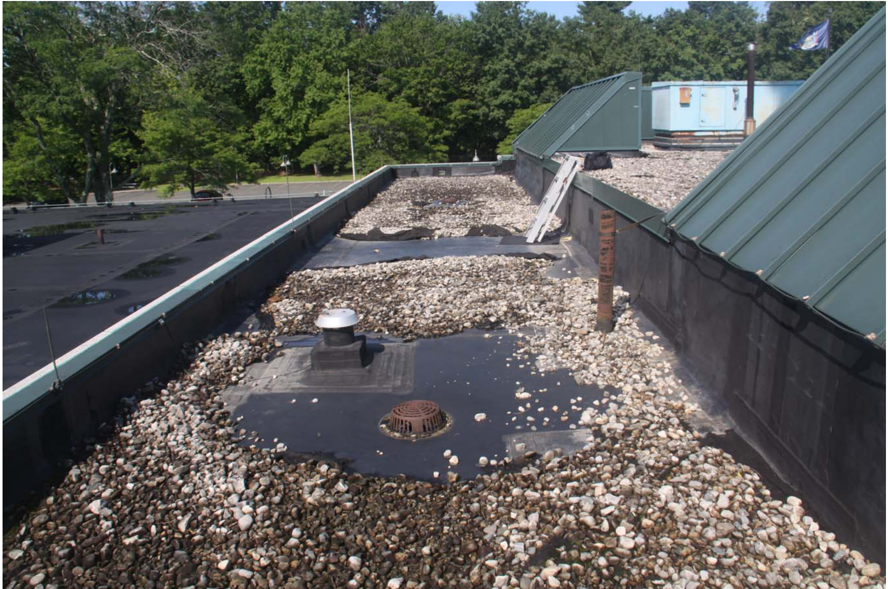
2219-00_19_0801 - ECs Roof [MP] (1081).JPG
