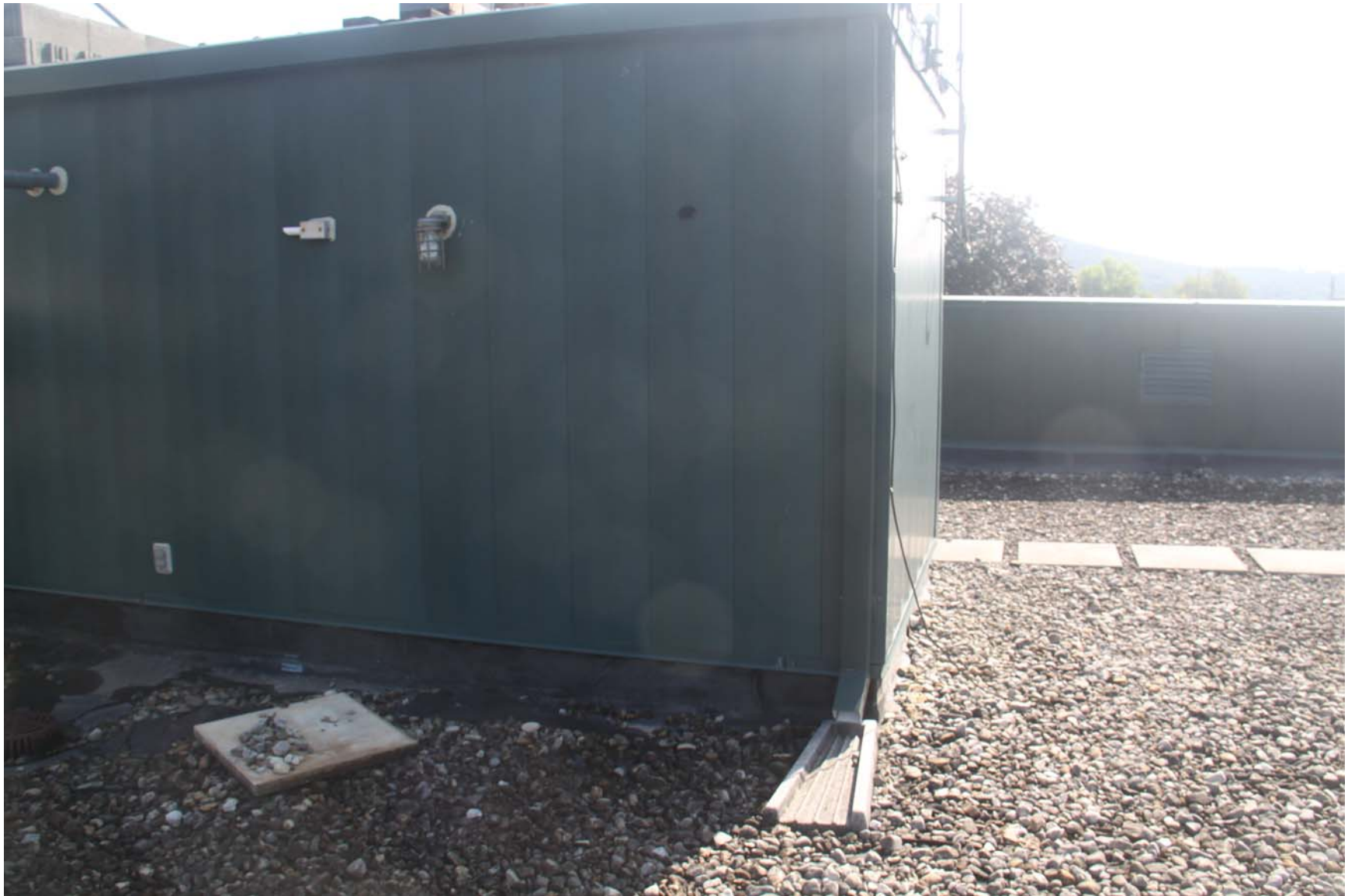
2219-00_19_0801 - ECs Roof [MP] (1112).JPG
