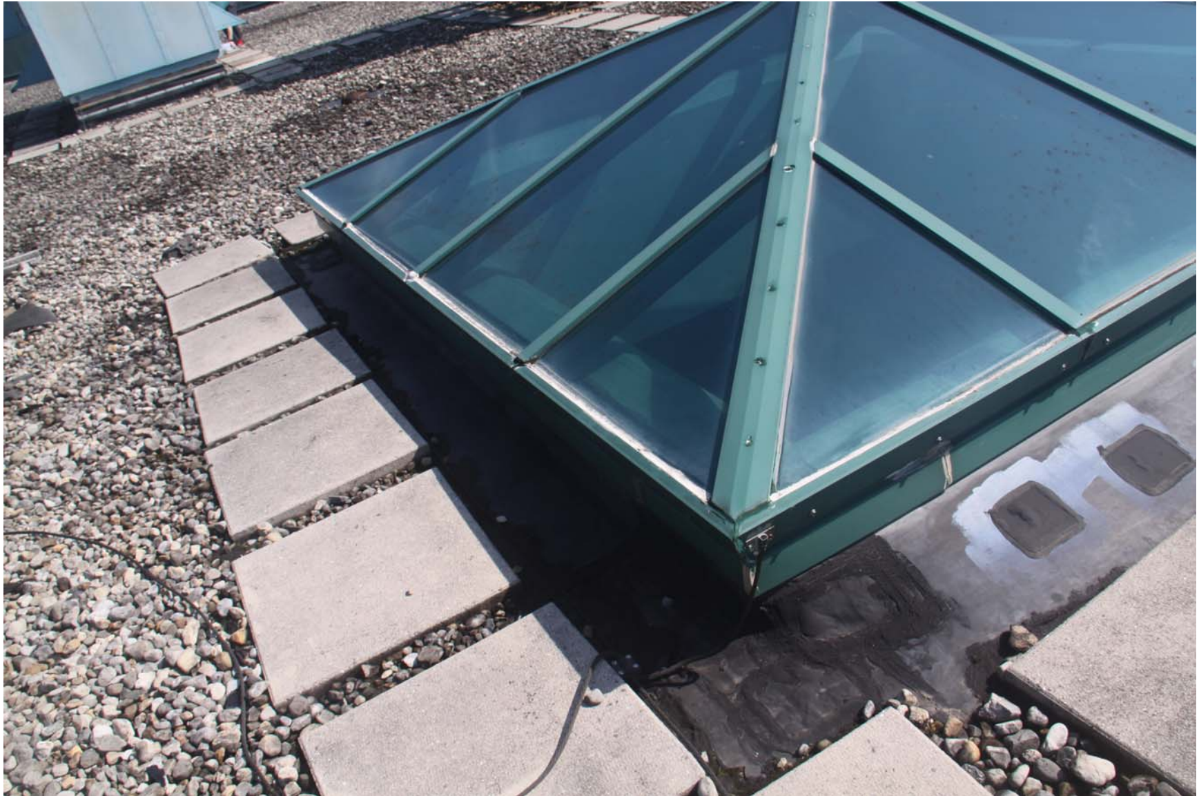
2219-00_19_0801 - ECs Roof [MP] (1103).JPG
