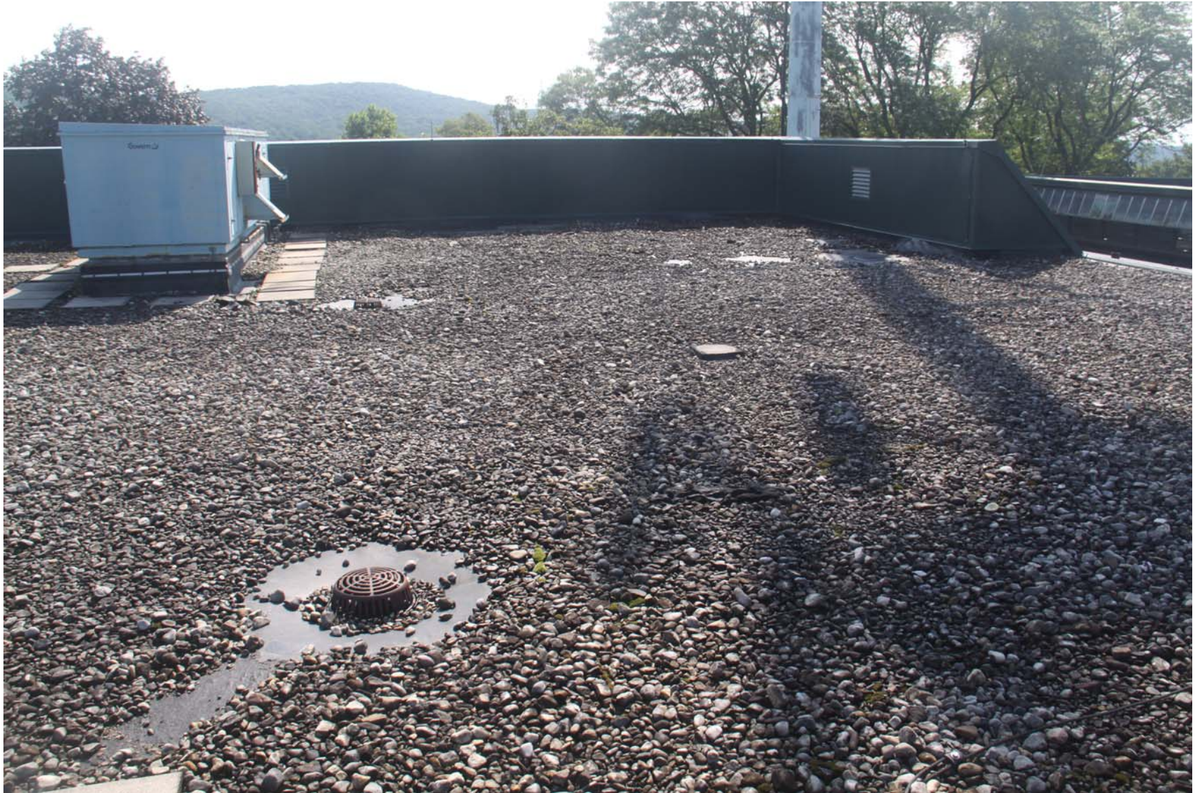
2219-00_19_0801 - ECs Roof [MP] (1095).JPG
