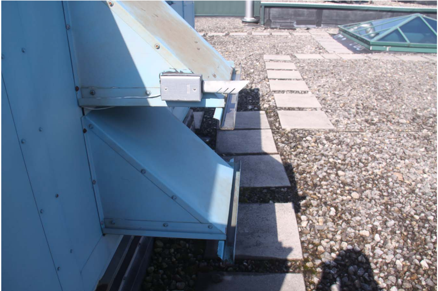
2219-00_19_0801 - ECs Roof [MP] (1034).JPG
