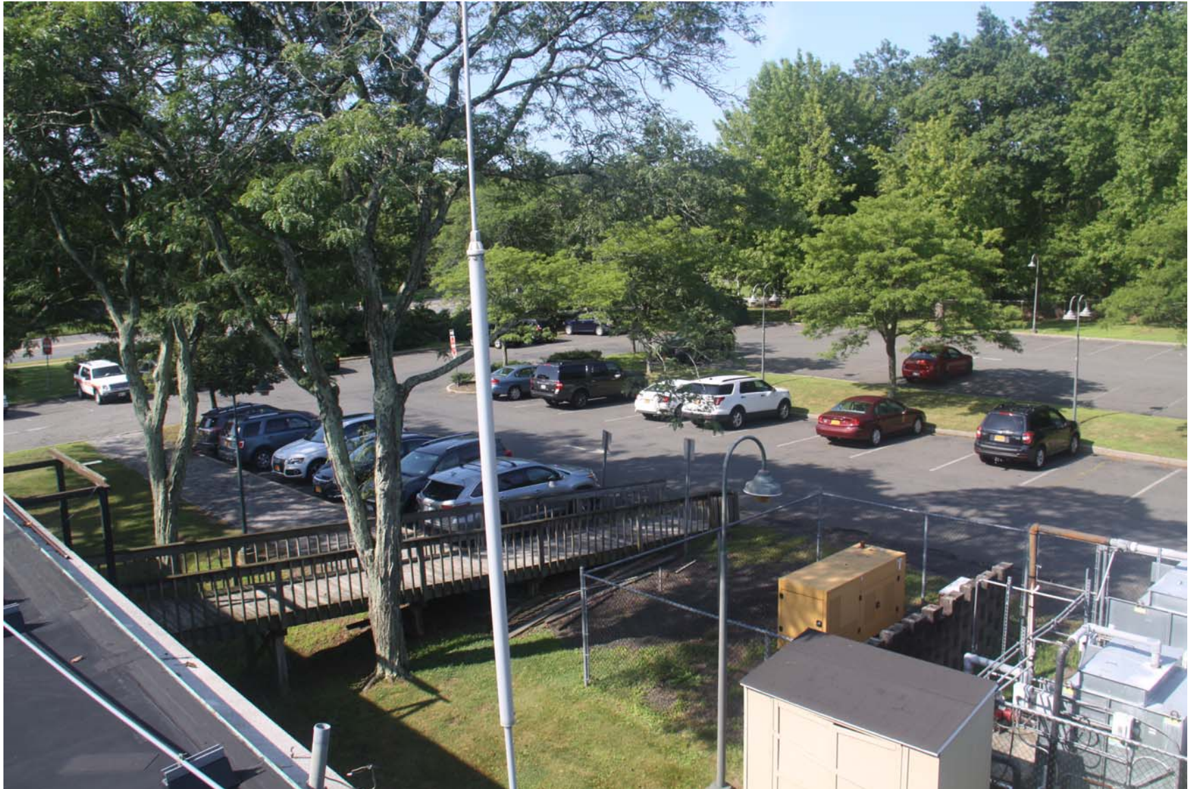
2219-00_19_0801 - ECs Roof [MP] (1056).JPG
