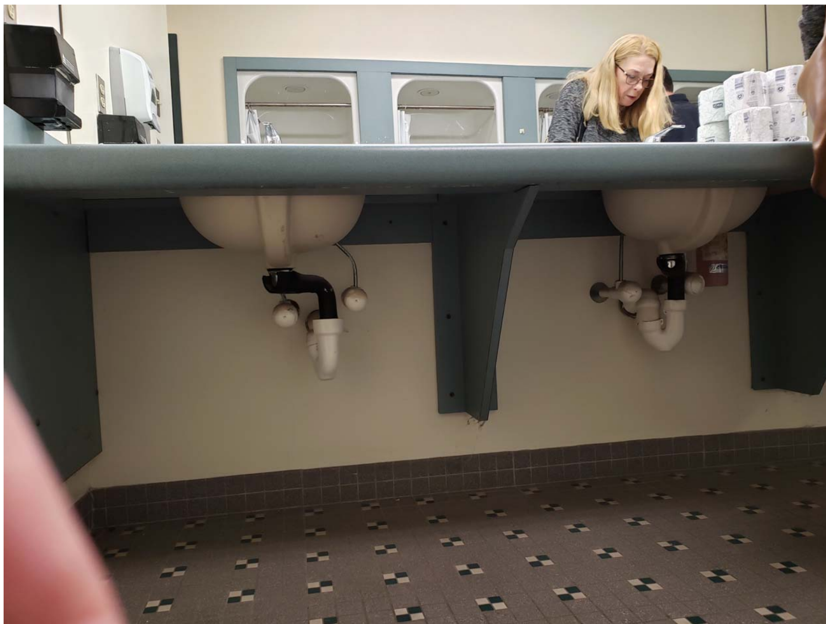
2219-00_19_1025 - ECs Mens Locker RR UL [BG] (9423).jpg
