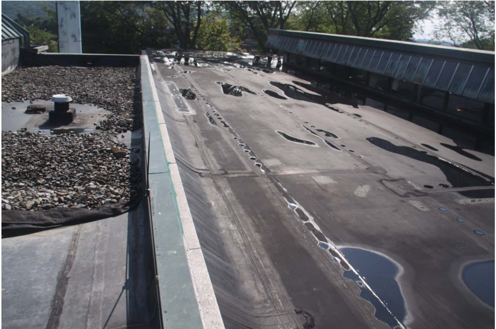
2219-00_19_0801 - ECs Roof [MP] (1069).JPG
