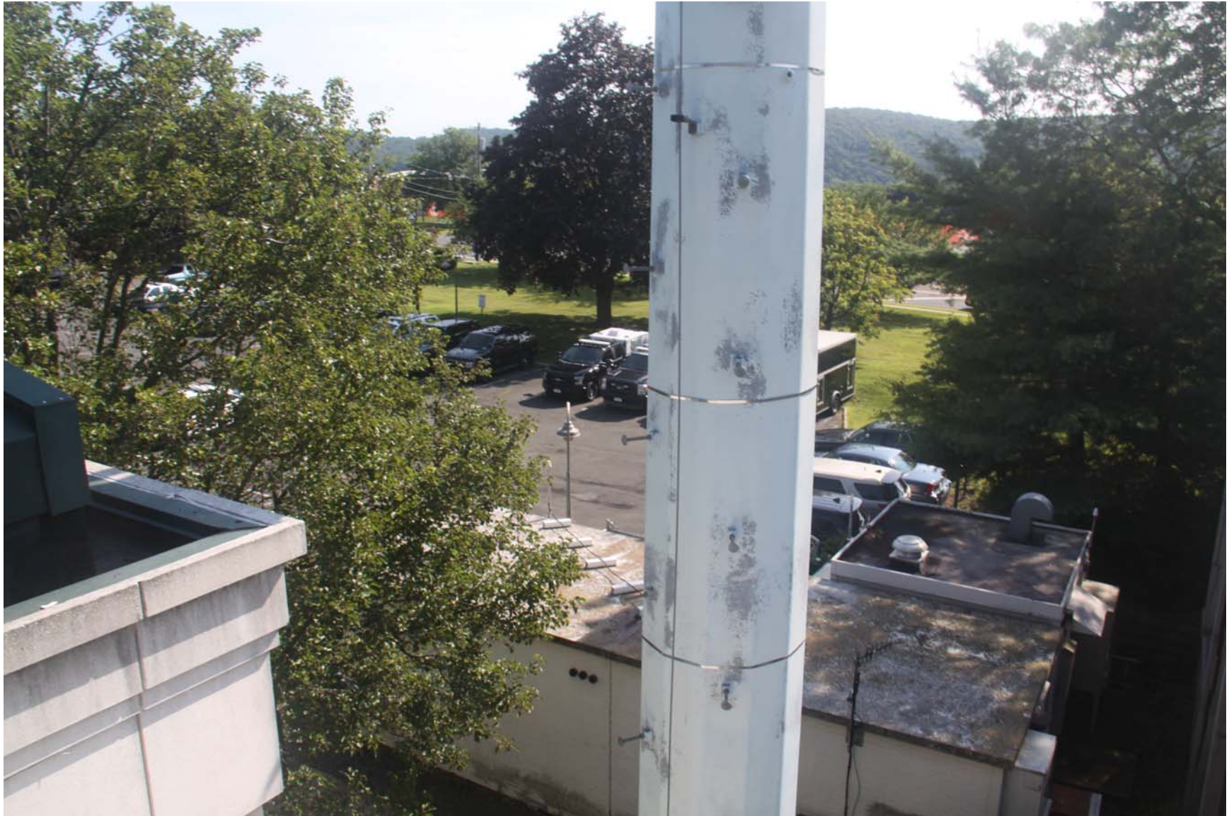
2219-00_19_0801 - ECs Roof [MP] (1076).JPG
