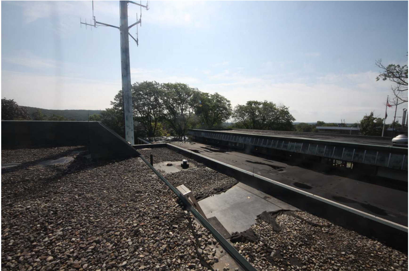
2219-00_19_0801 - ECs Roof [MP] (1180).JPG
