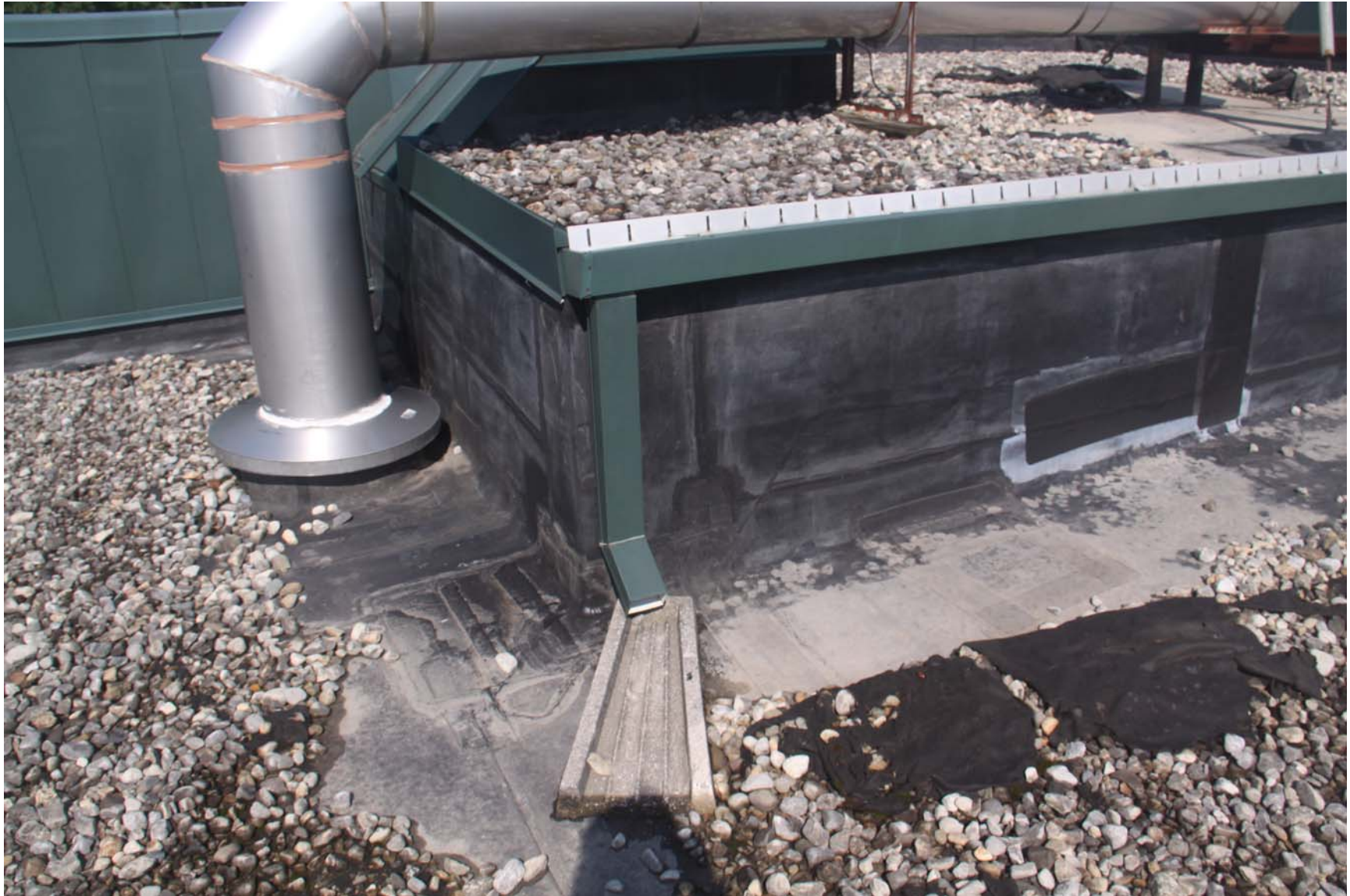
2219-00_19_0801 - ECs Roof [MP] (1098).JPG
