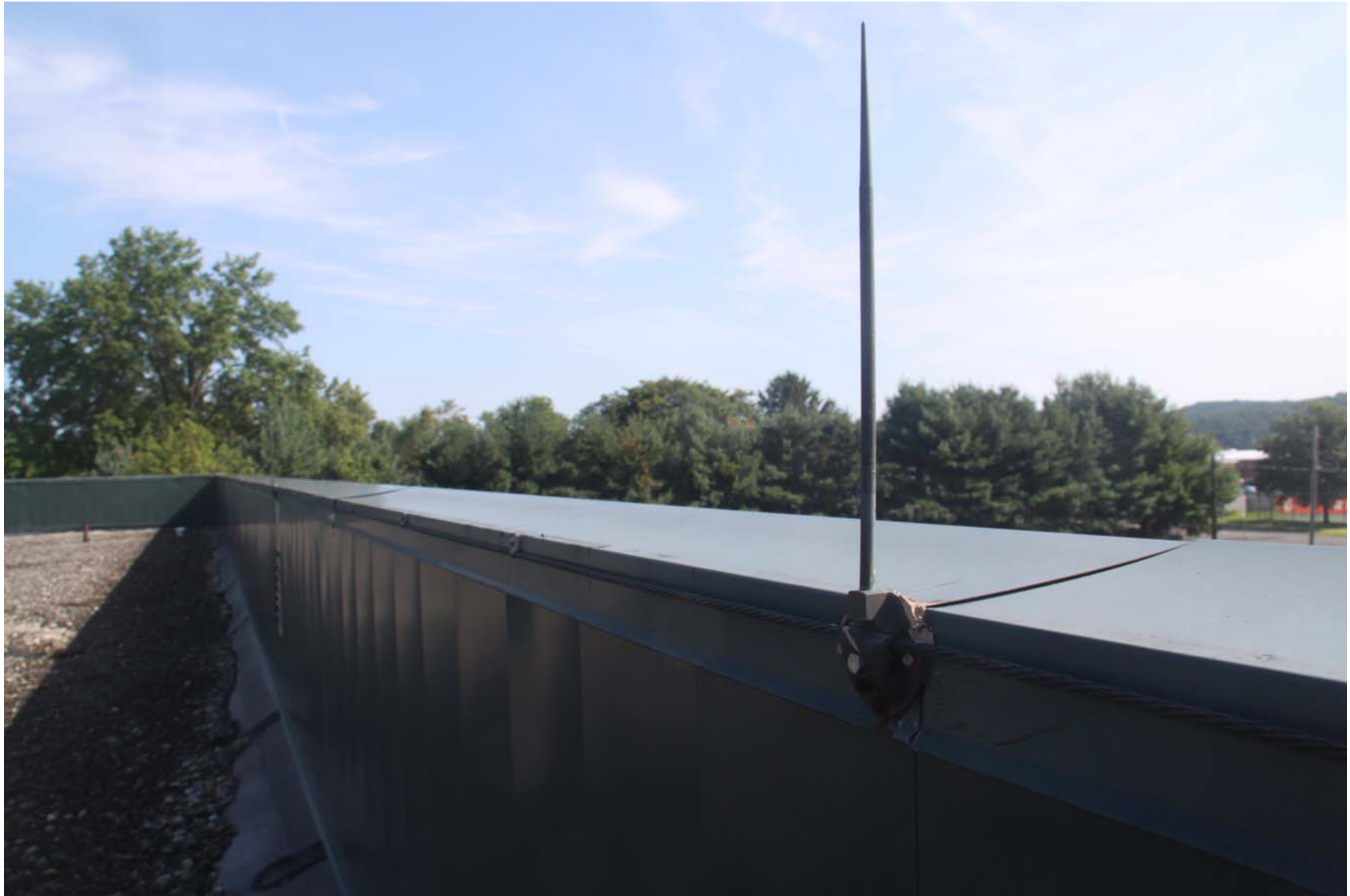
2219-00_19_0801 - ECs Roof [MP] (1032).JPG
