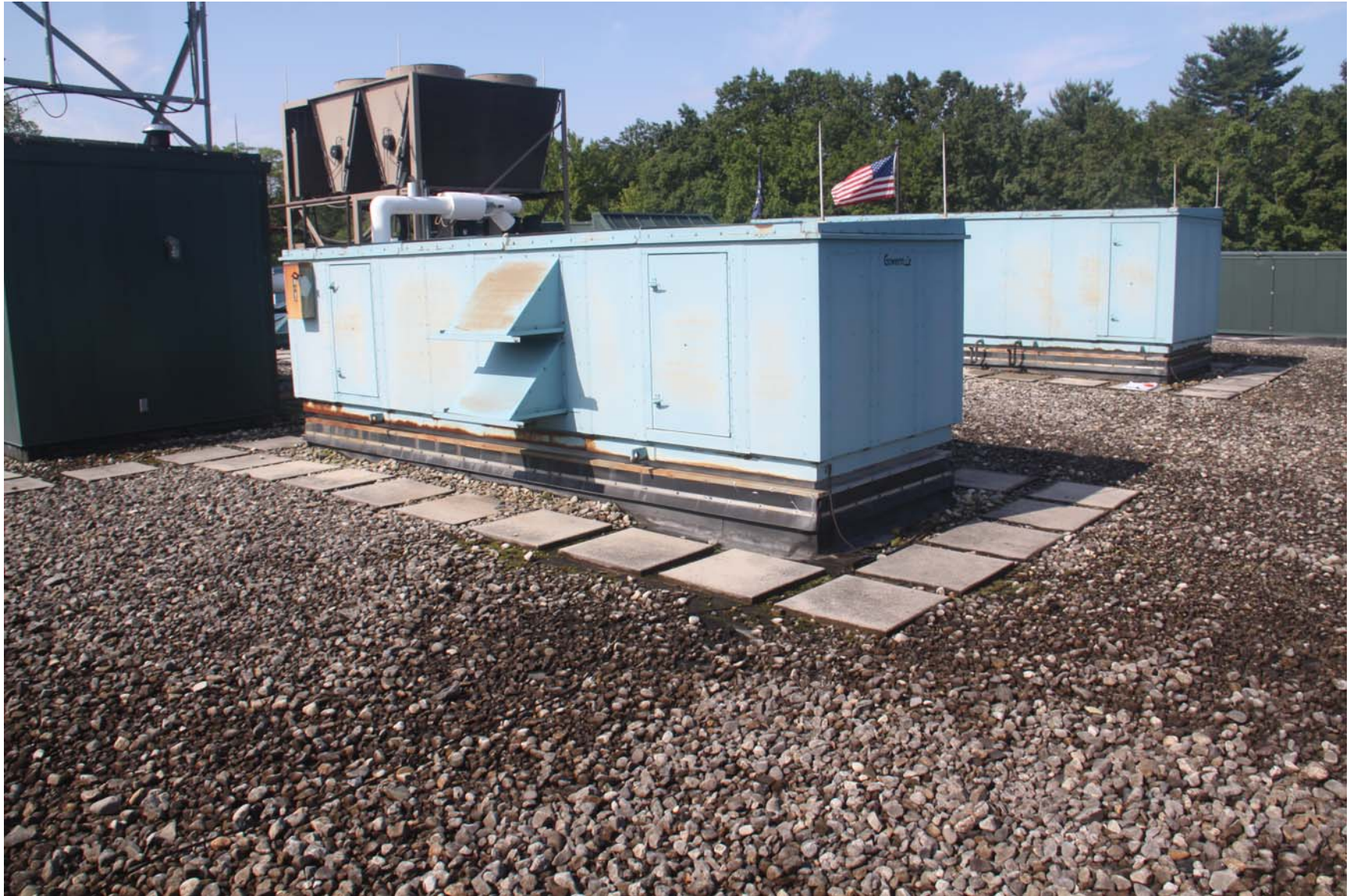
2219-00_19_0801 - ECs Roof [MP] (1010).JPG
