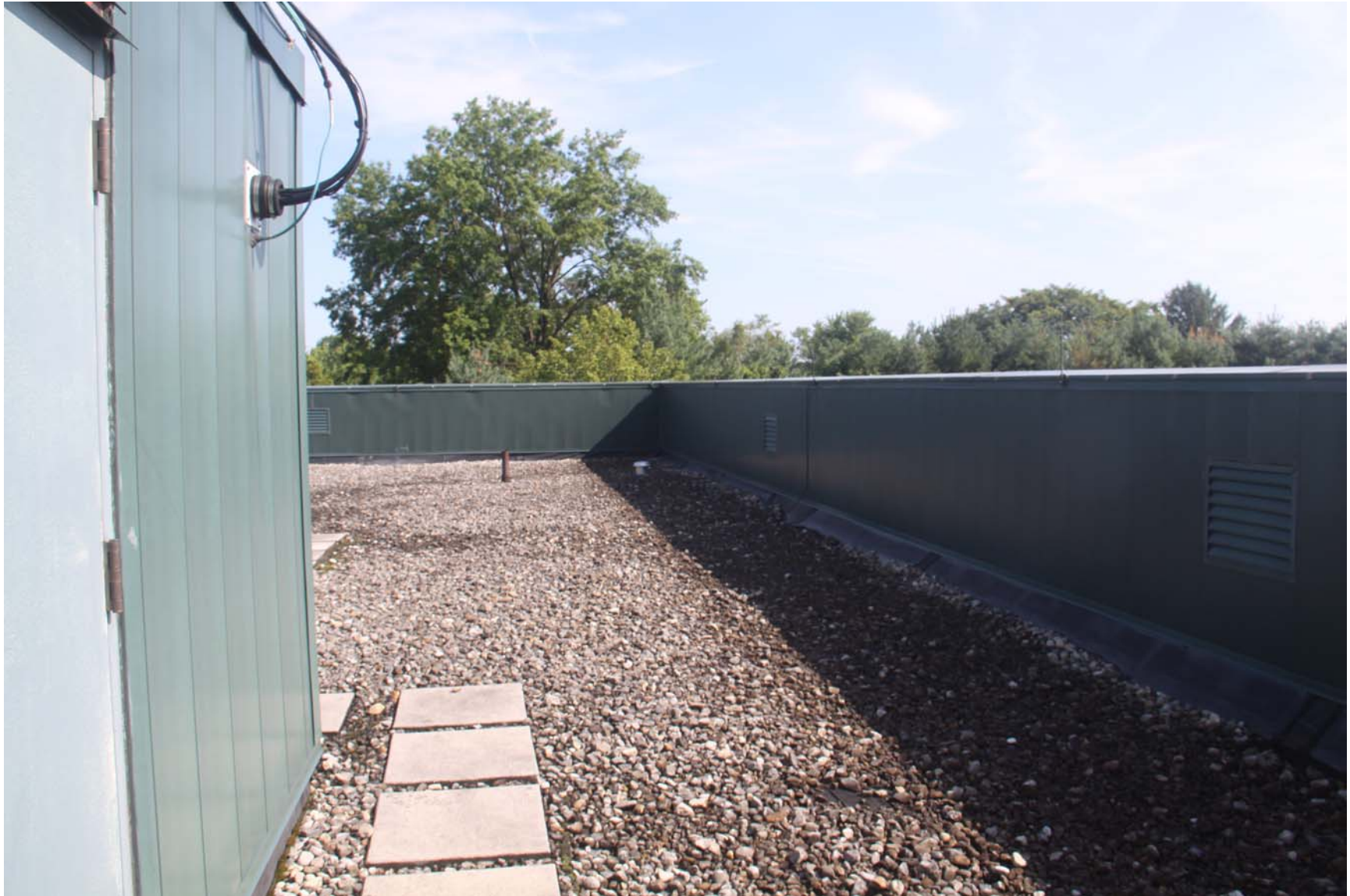
2219-00_19_0801 - ECs Roof [MP] (1021).JPG
