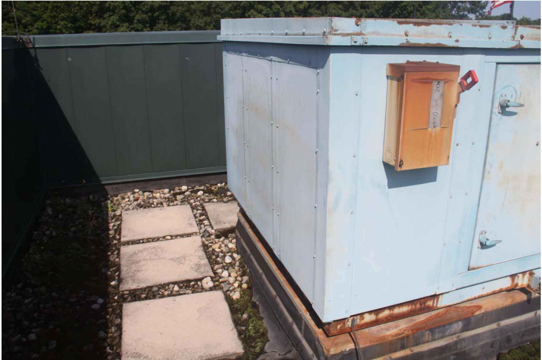
2219-00_19_0801 - ECs Roof [MP] (1088).JPG
