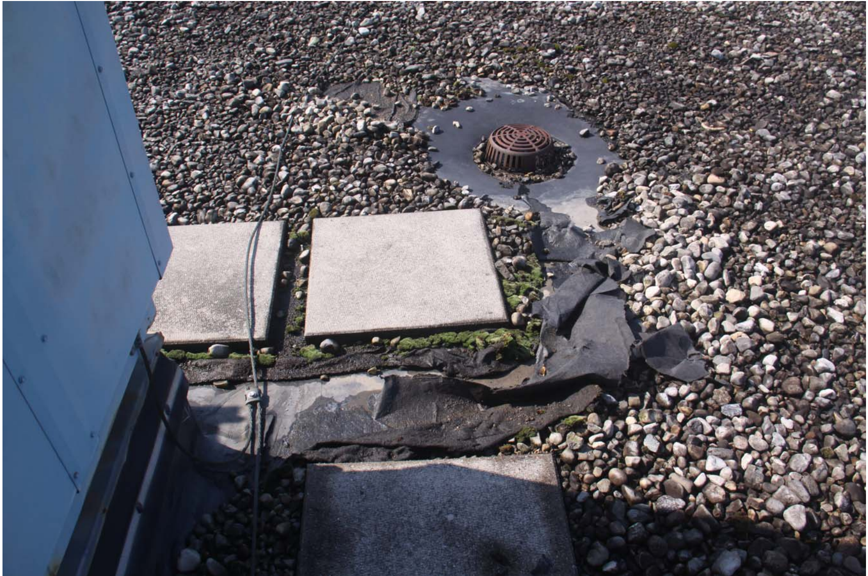
2219-00_19_0801 - ECs Roof [MP] (1035).JPG
