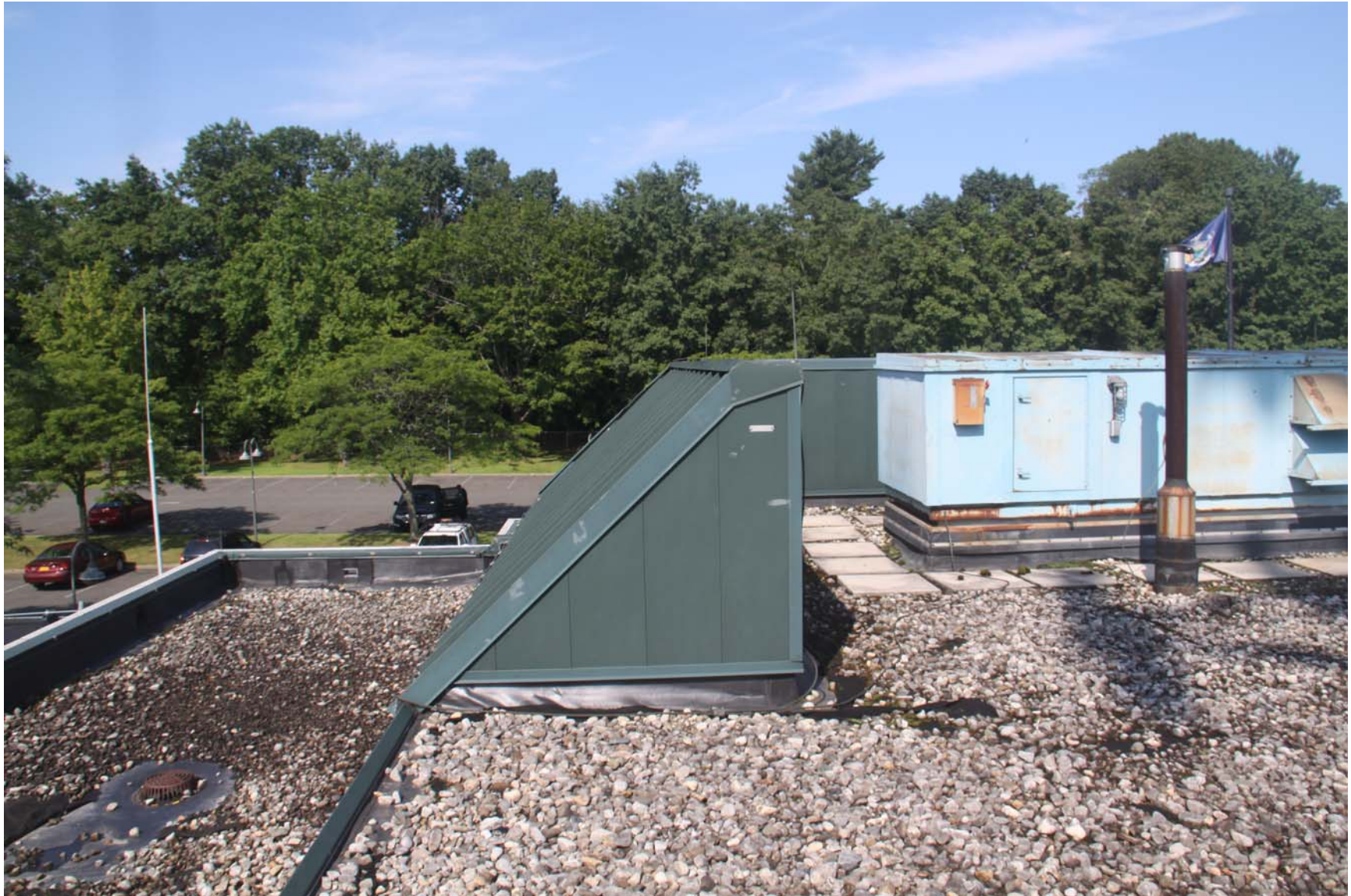
2219-00_19_0801 - ECs Roof [MP] (1048).JPG
