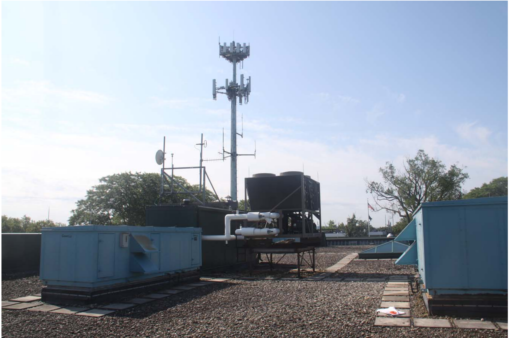
2219-00_19_0801 - ECs Roof [MP] (1130).JPG
