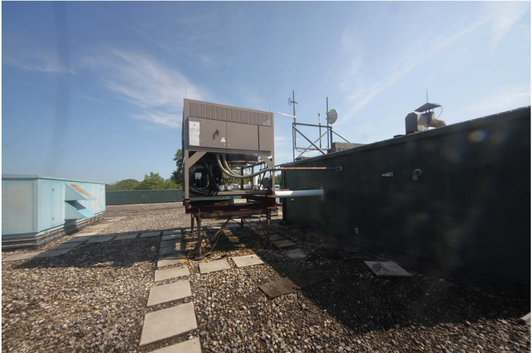
2219-00_19_0801 - ECs Roof [MP] (1166).JPG
