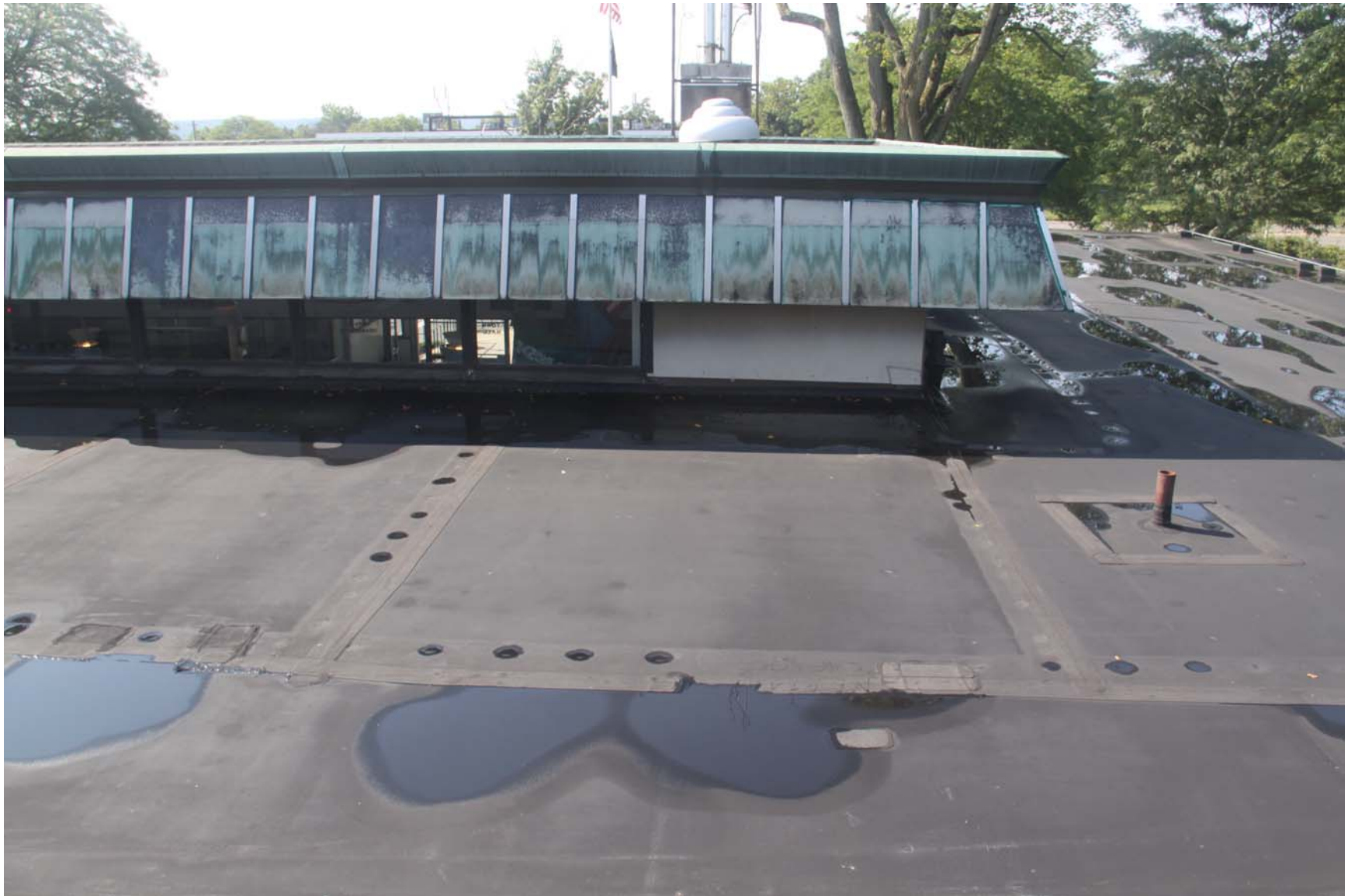
2219-00_19_0801 - ECs Roof [MP] (1071).JPG
