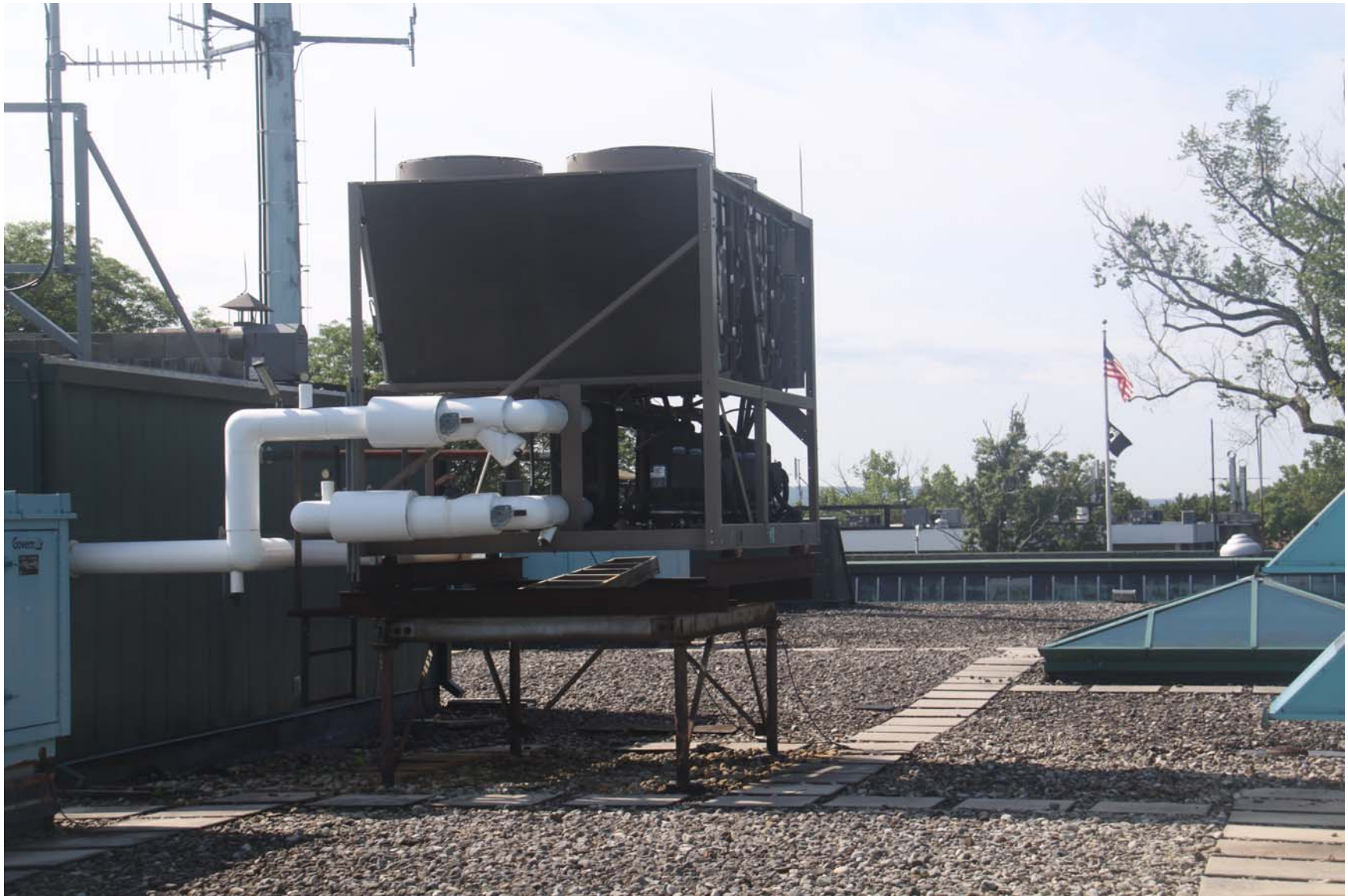
2219-00_19_0801 - ECs Roof [MP] (1129).JPG
