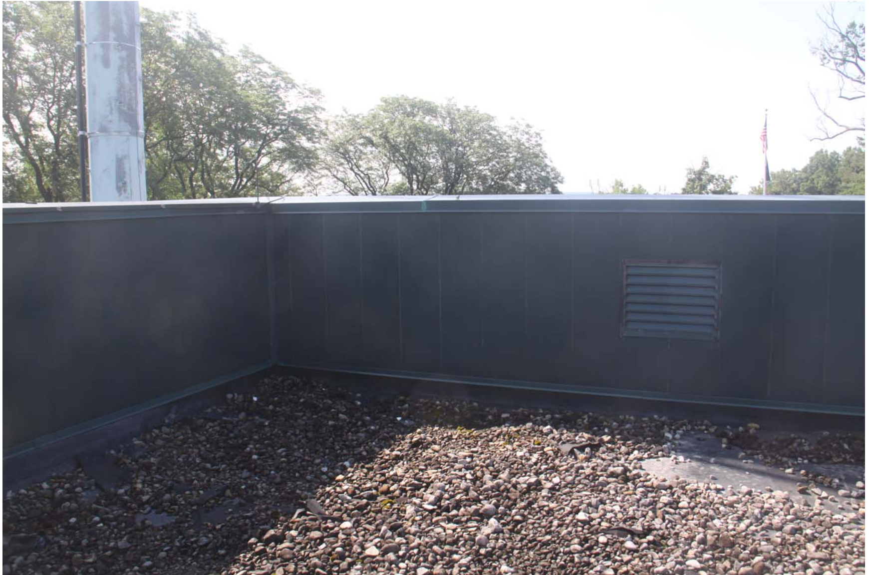
2219-00_19_0801 - ECs Roof [MP] (1039).JPG
