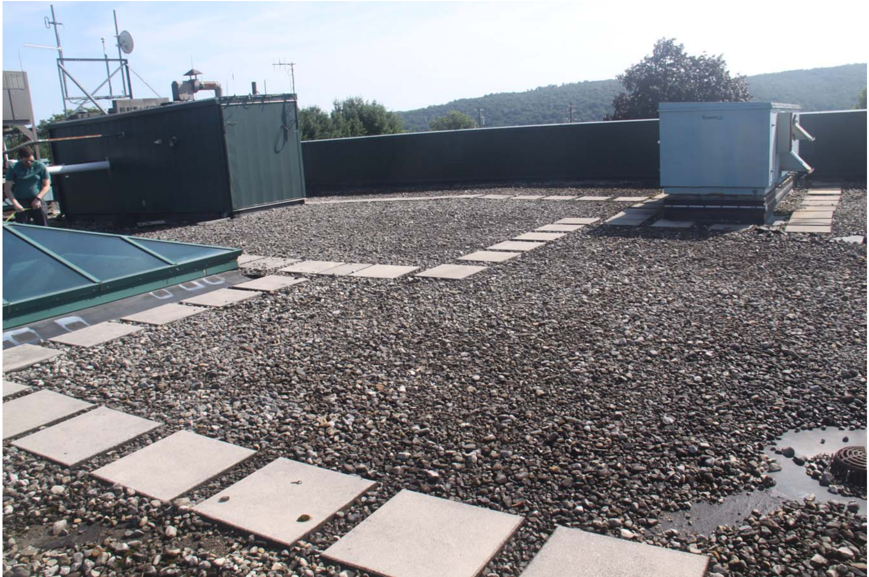
2219-00_19_0801 - ECs Roof [MP] (1096).JPG
