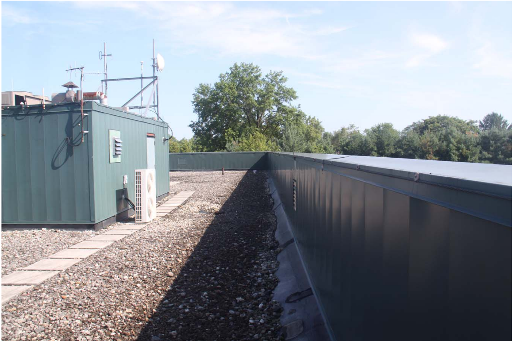
2219-00_19_0801 - ECs Roof [MP] (1031).JPG
