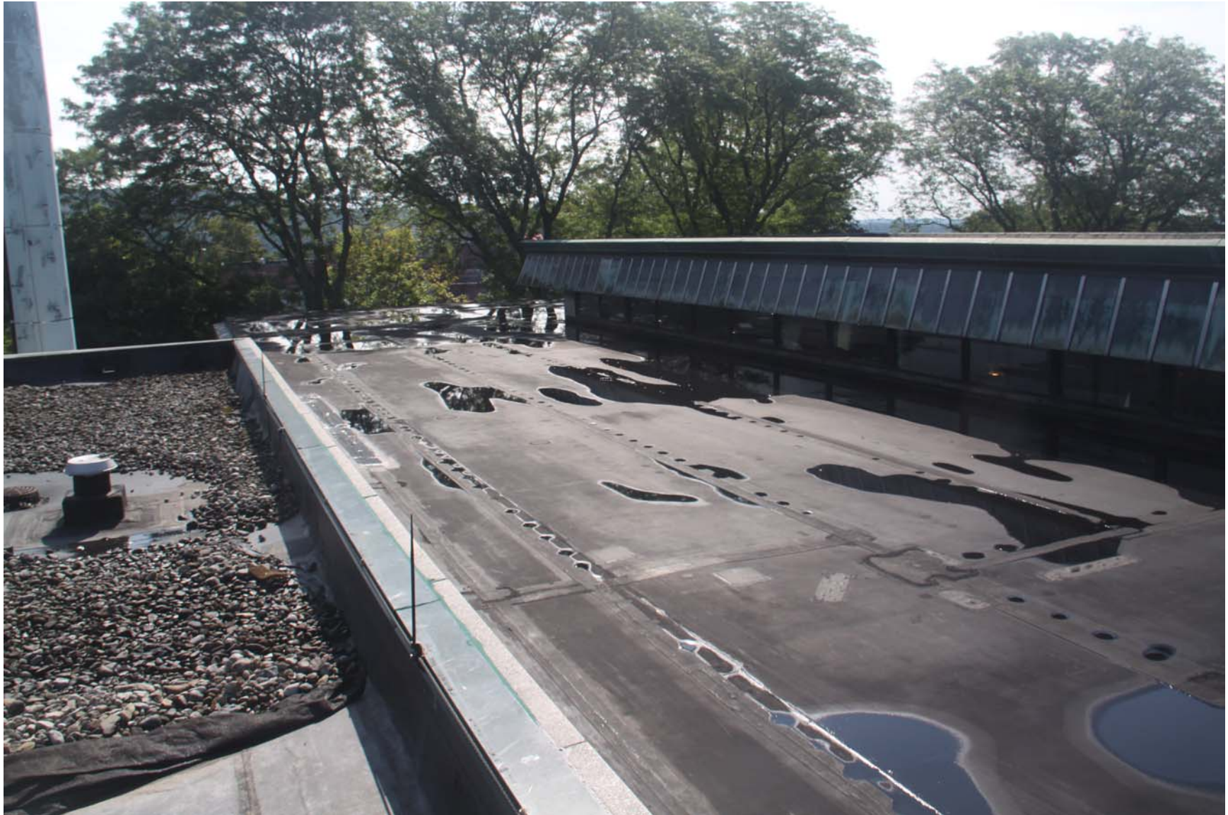
2219-00_19_0801 - ECs Roof [MP] (1070).JPG
