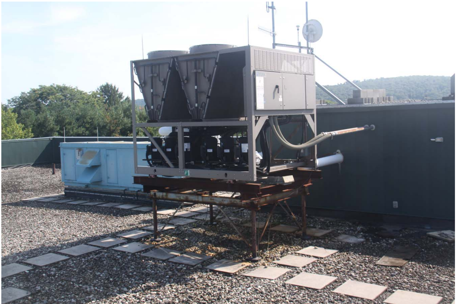
2219-00_19_0801 - ECs Roof [MP] (1152).JPG
