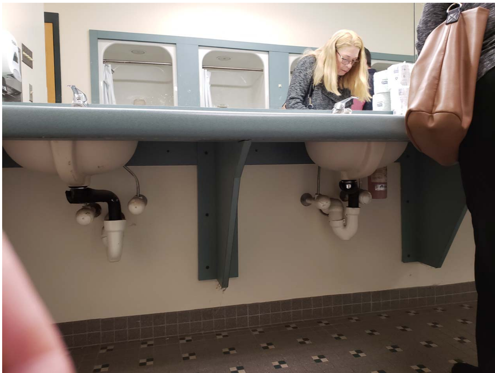
2219-00_19_1025 - ECs Mens Locker RR UL [BG] (9424).jpg
