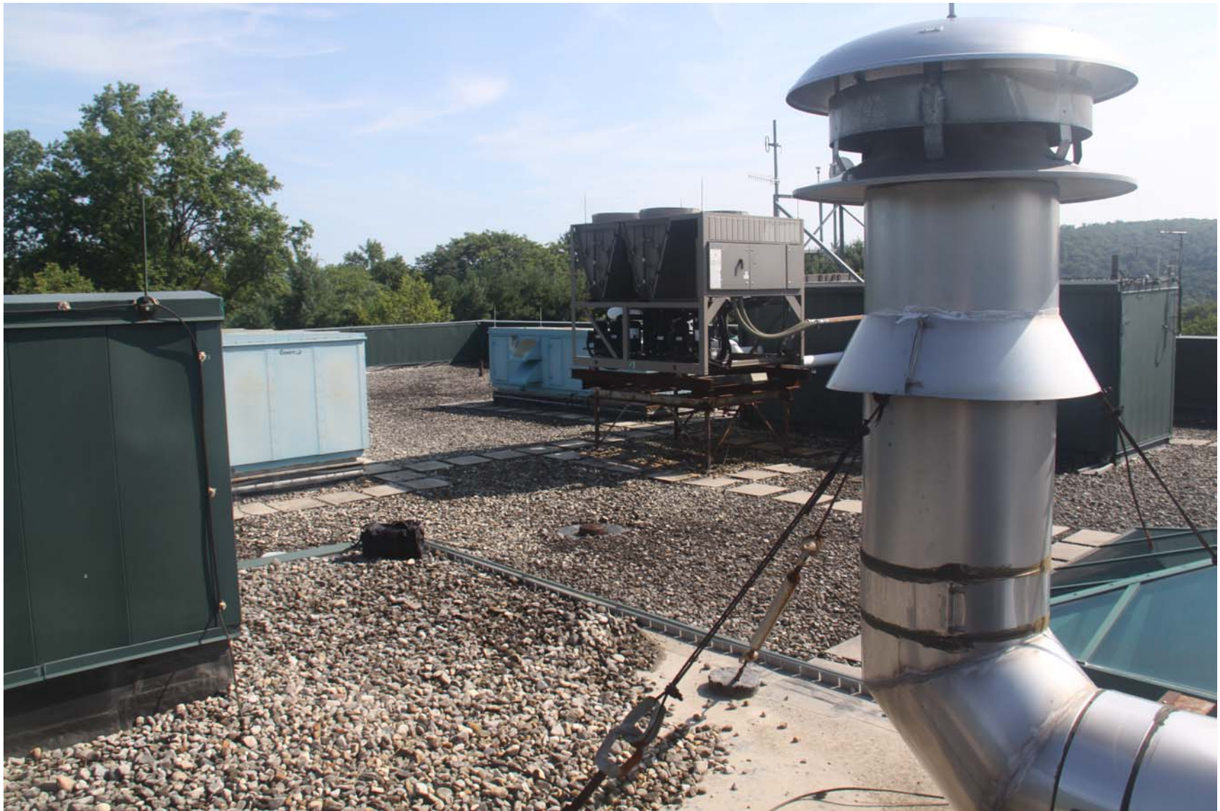
2219-00_19_0801 - ECs Roof [MP] (1137).JPG
