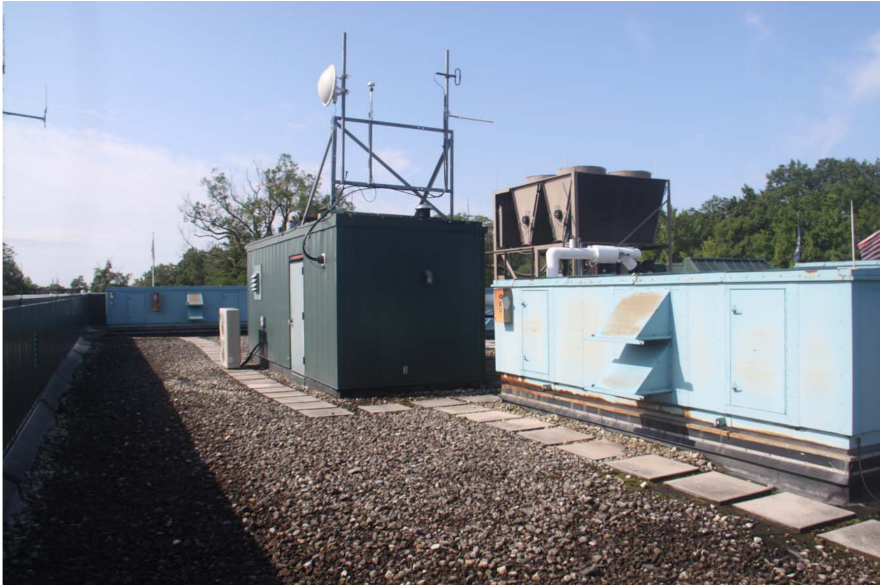
2219-00_19_0801 - ECs Roof [MP] (1011).JPG
