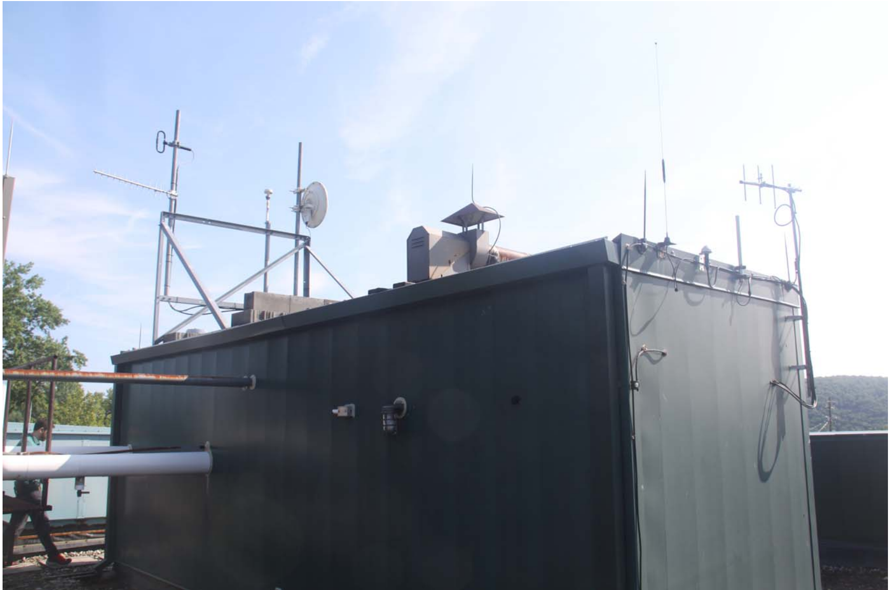
2219-00_19_0801 - ECs Roof [MP] (1115).JPG
