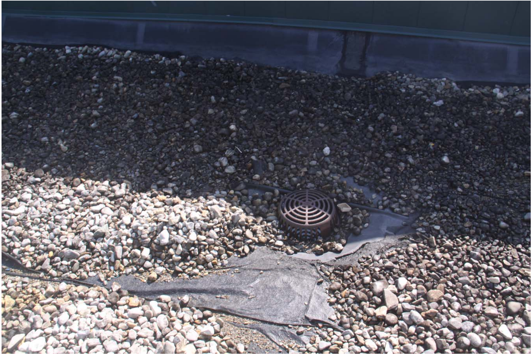
2219-00_19_0801 - ECs Roof [MP] (1022).JPG
