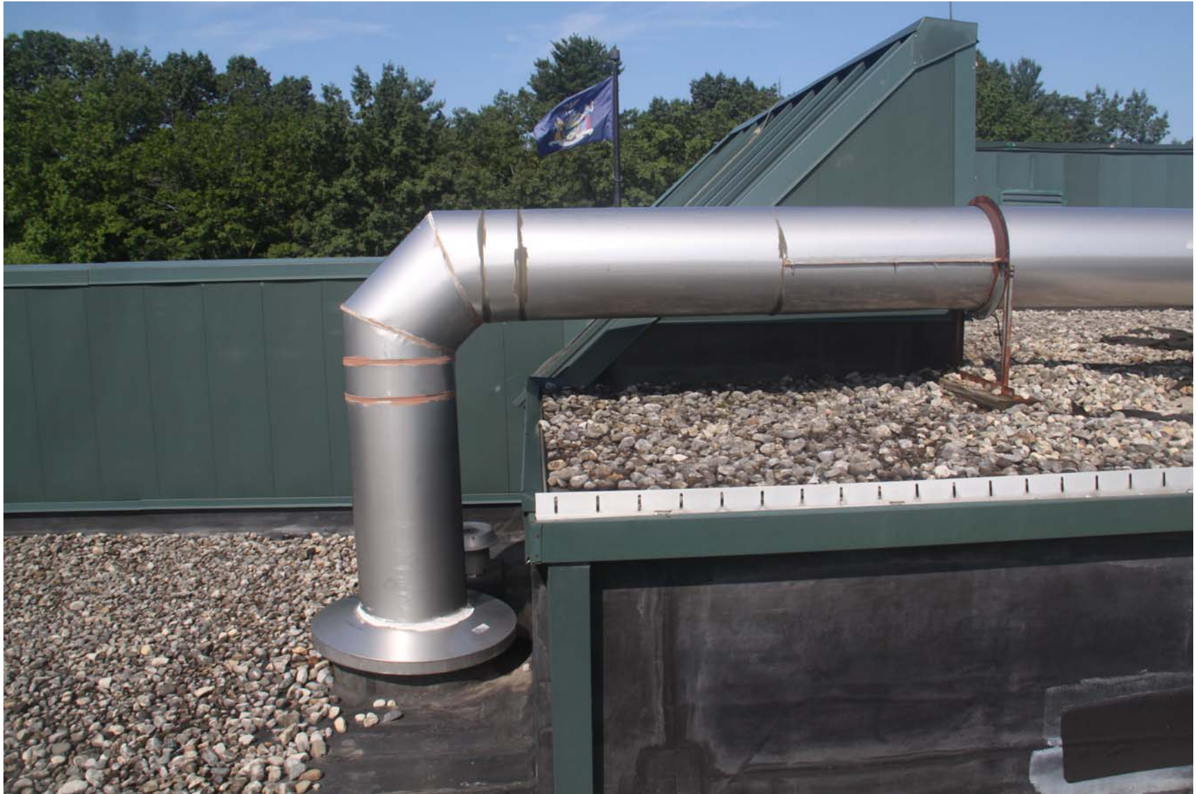
2219-00_19_0801 - ECs Roof [MP] (1099).JPG
