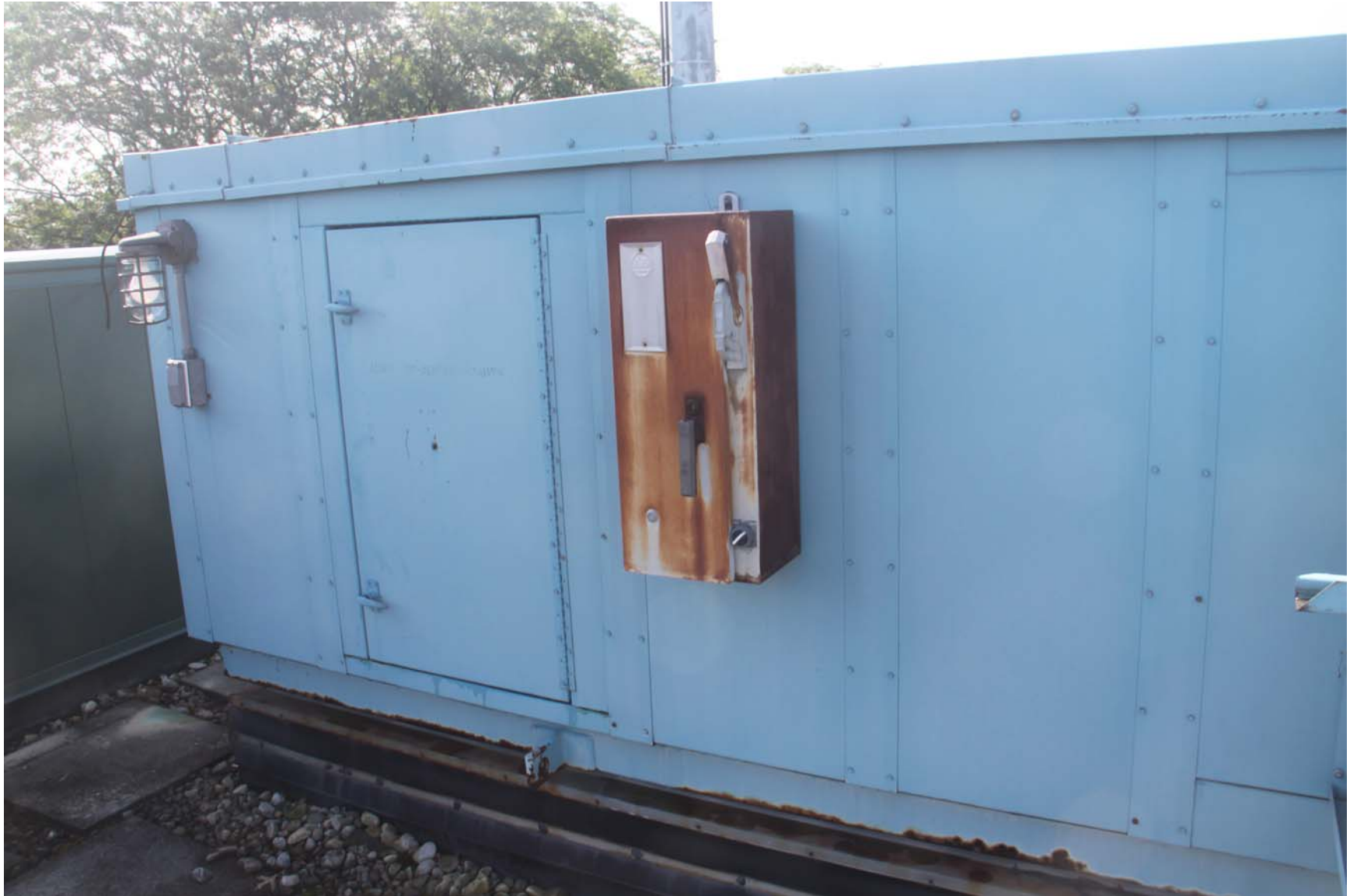
2219-00_19_0801 - ECs Roof [MP] (1030).JPG
