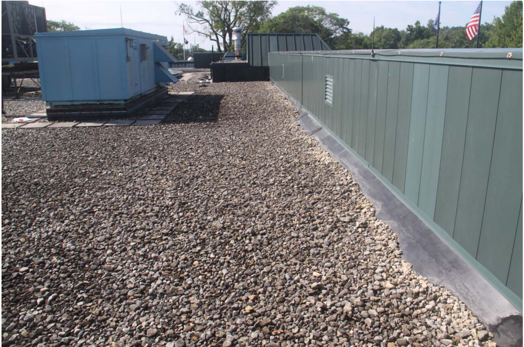
2219-00_19_0801 - ECs Roof [MP] (1124).JPG
