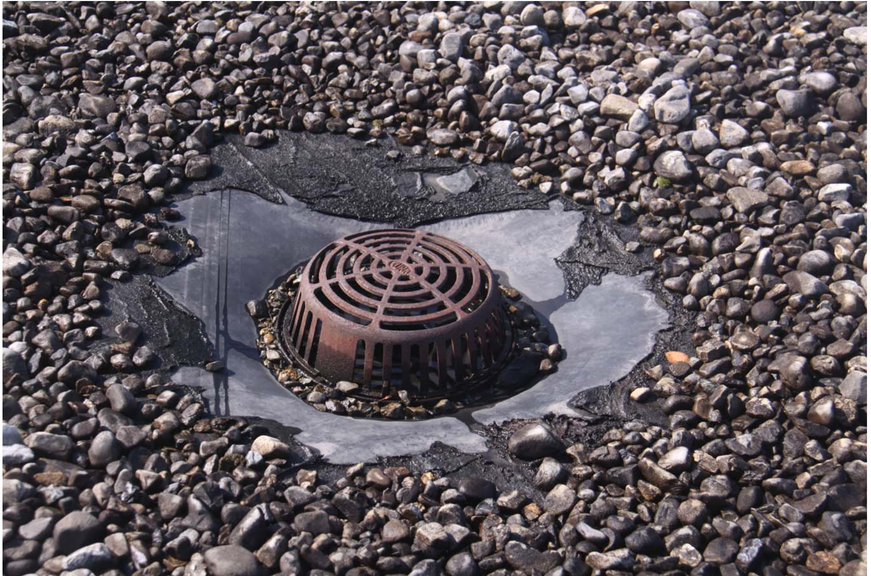
2219-00_19_0801 - ECs Roof [MP] (1009).JPG
