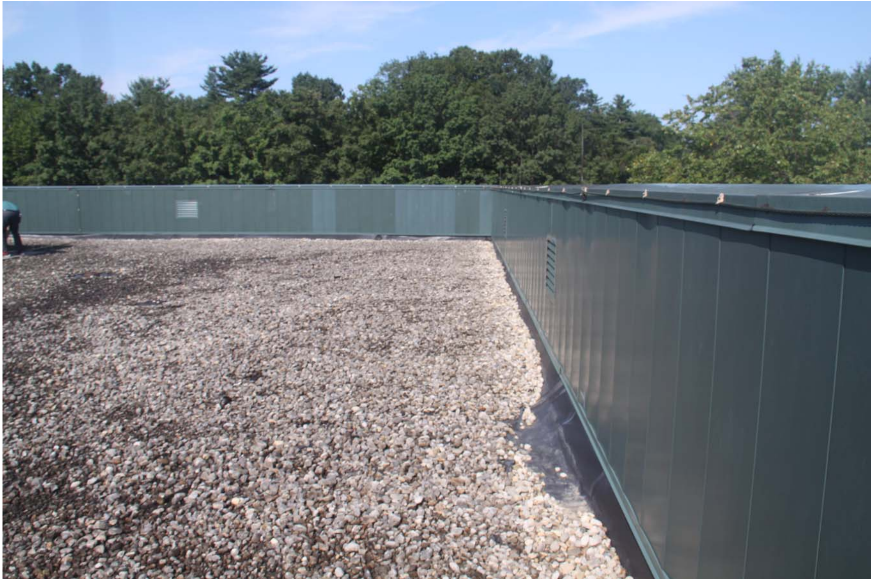
2219-00_19_0801 - ECs Roof [MP] (1006).JPG
