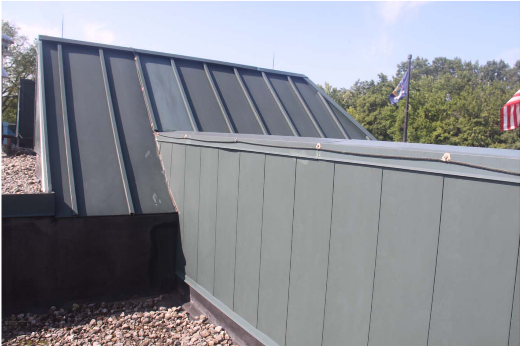
2219-00_19_0801 - ECs Roof [MP] (1121).JPG
