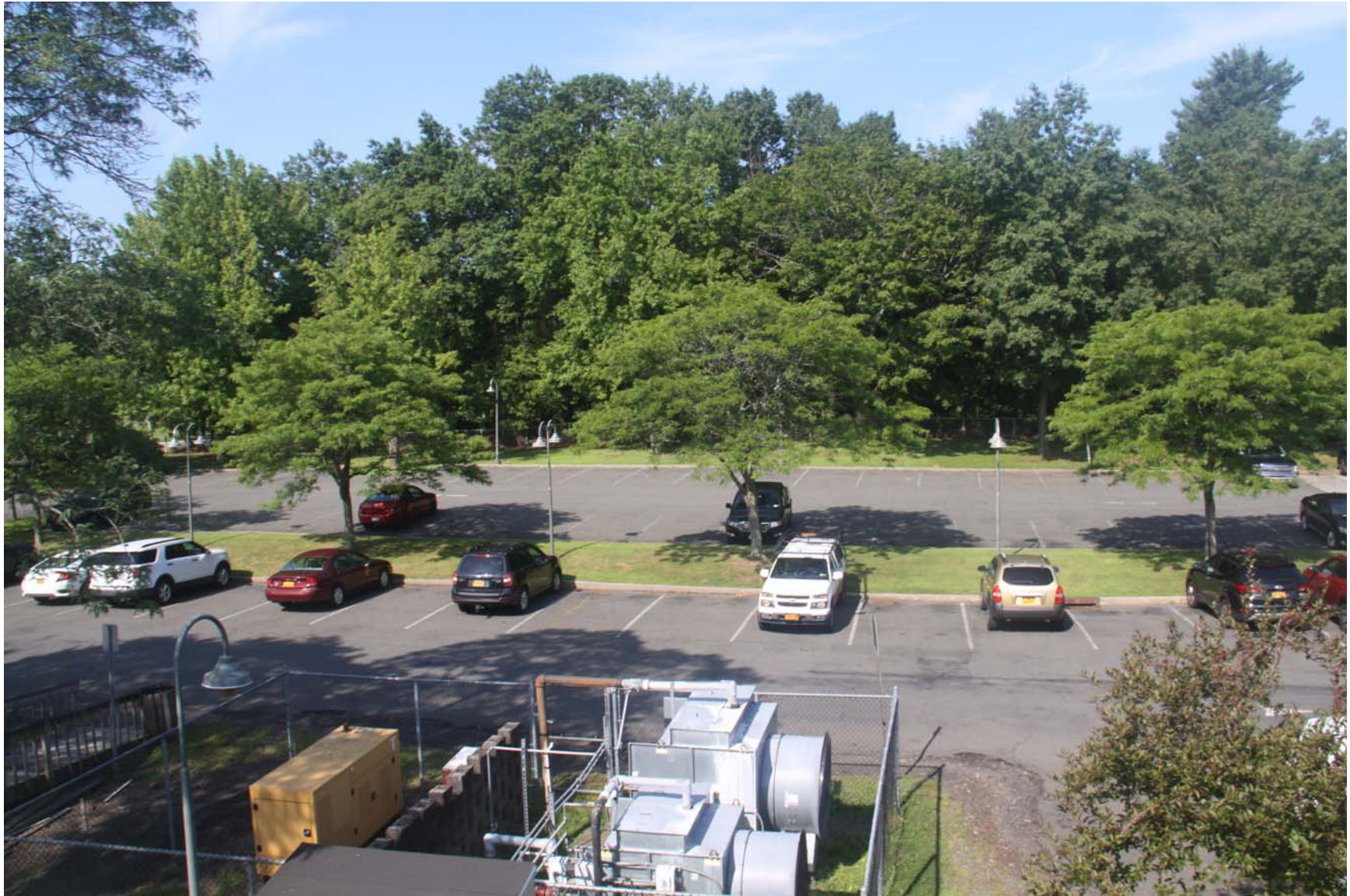
2219-00_19_0801 - ECs Roof [MP] (1063).JPG
