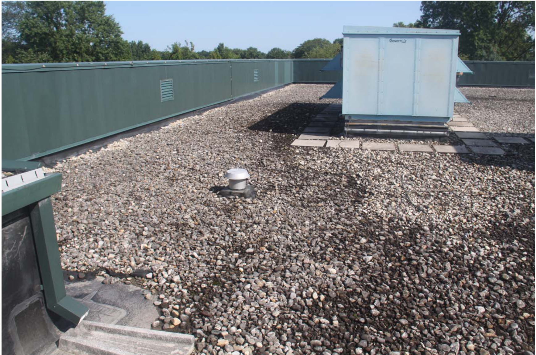
2219-00_19_0801 - ECs Roof [MP] (1107).JPG
