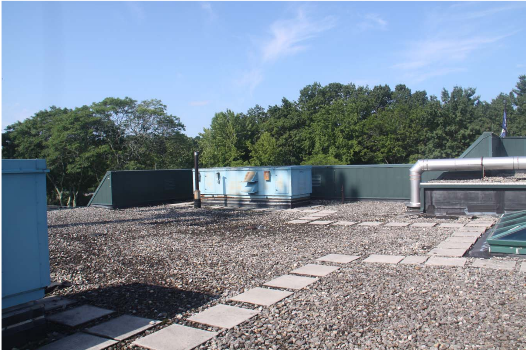
2219-00_19_0801 - ECs Roof [MP] (1027).JPG
