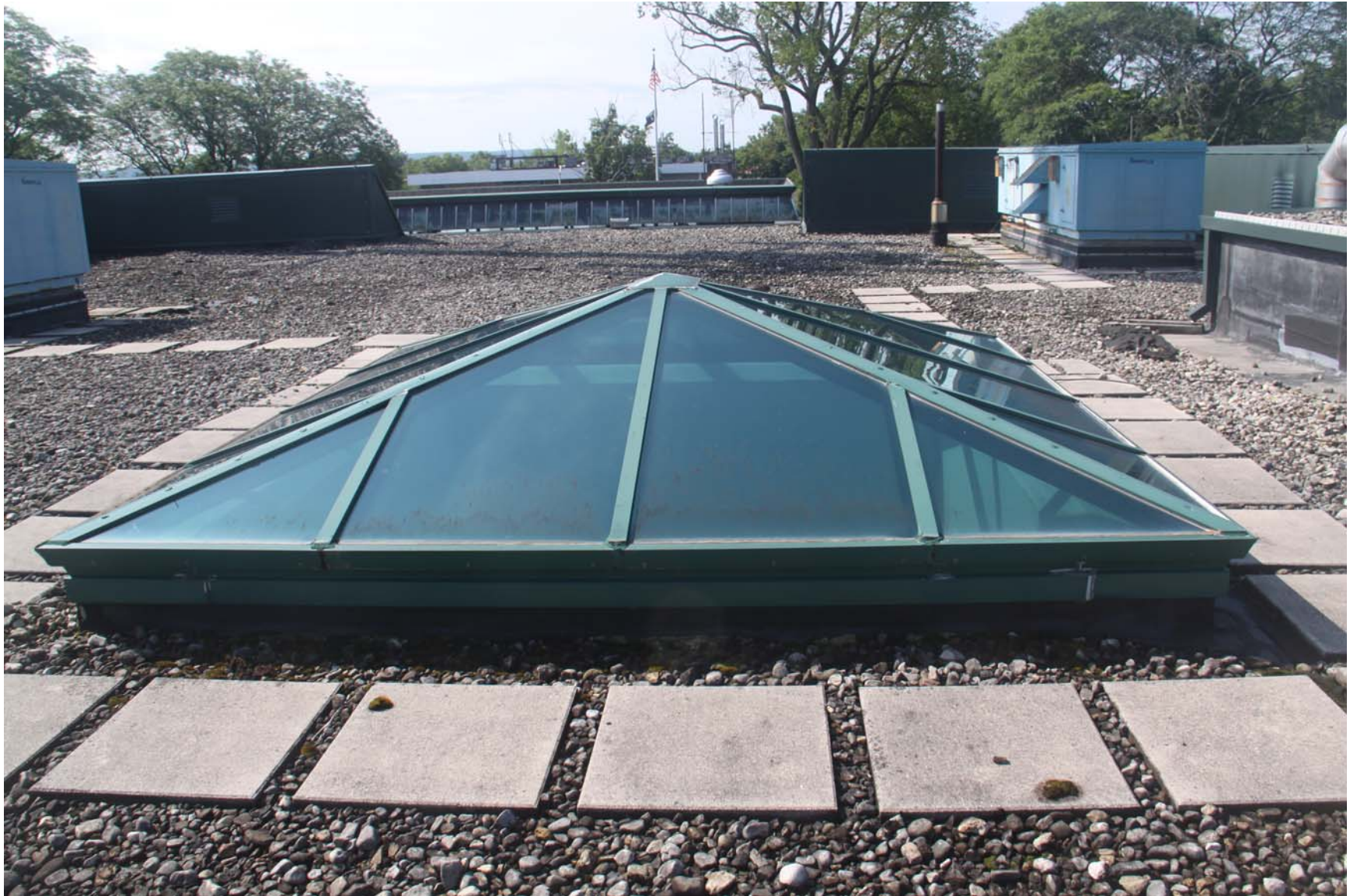
2219-00_19_0801 - ECs Roof [MP] (1109).JPG
