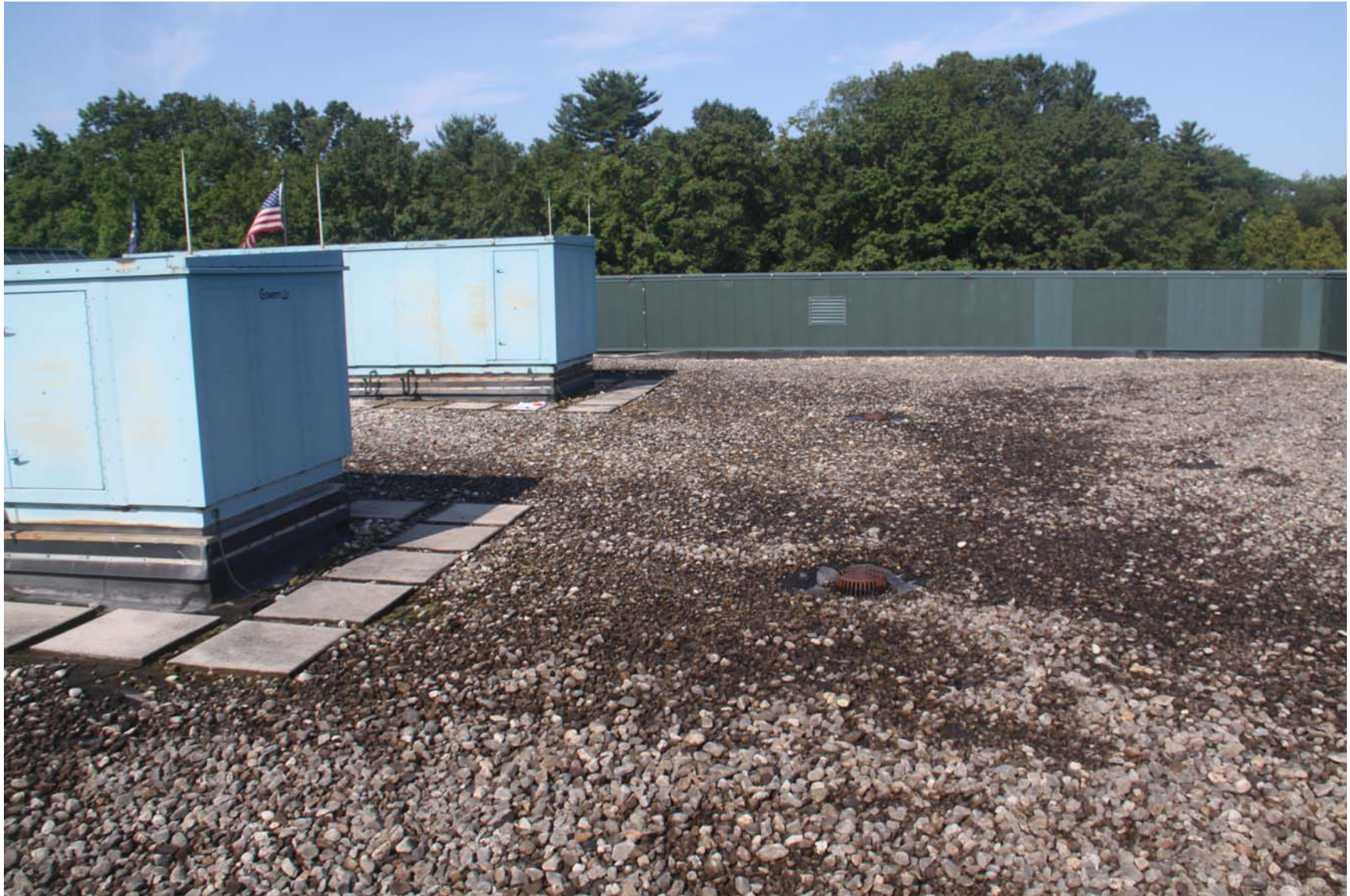
2219-00_19_0801 - ECs Roof [MP] (1012).JPG
