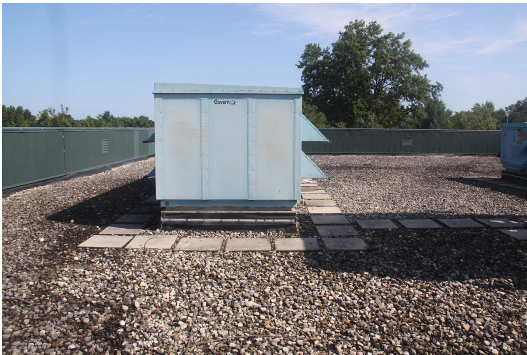
2219-00_19_0801 - ECs Roof [MP] (1116).JPG
