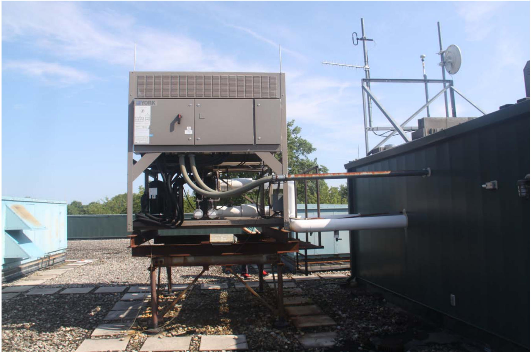
2219-00_19_0801 - ECs Roof [MP] (1114).JPG
