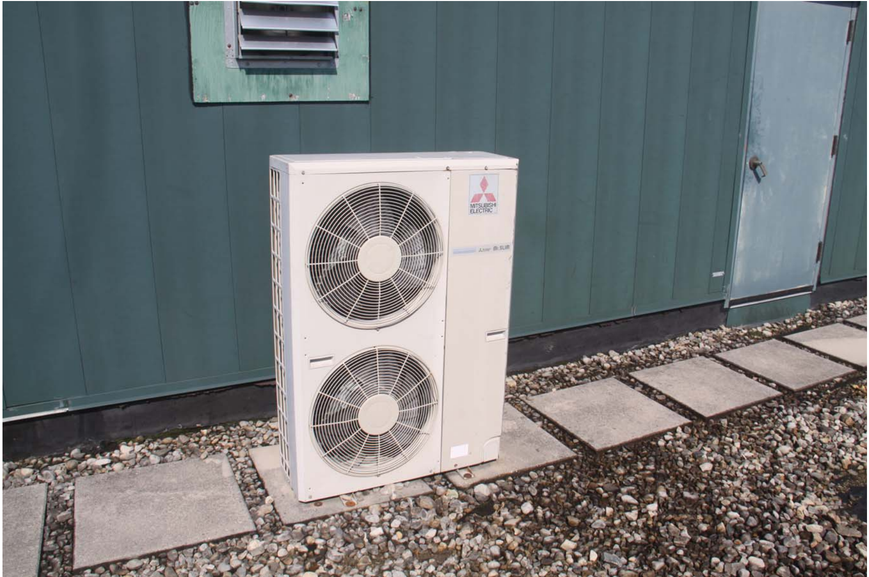
2219-00_19_0801 - ECs Roof [MP] (1023).JPG
