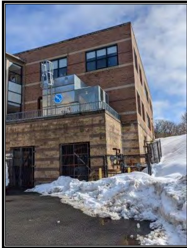
Photo 3: Non-ACM Mortar to Exterior CMU Wall (Gray)
