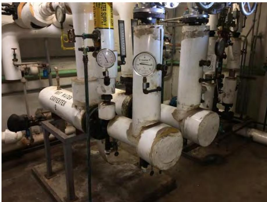
Photo 20 – View of the hot water converters in basement Mechanical Room MER 2 B-19. No asbestos was detected in gaskets at flanges the hot water converters. Photo taken May 13, 2021.
