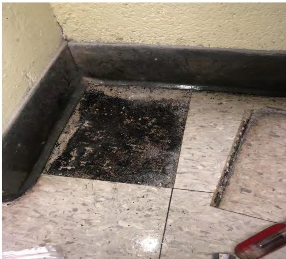
Photo 3 – View of 12"x12" floor tiles/mastic and cove base/mastic in basement room B-7. No asbestos was detected in these materials. Photo taken December 23, 2020.
