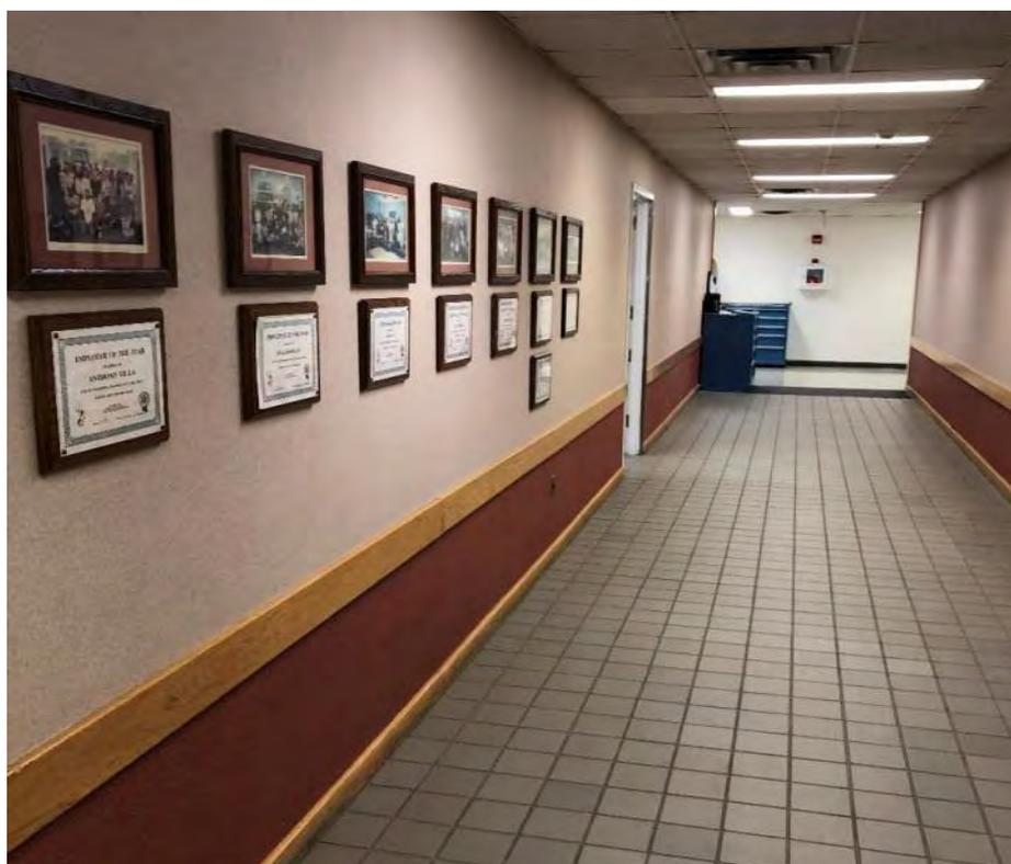
Photo 14 – View of quarry floor tiles, grout, mud-set & blue barrier on the first floor. No asbestos was detected in these materials. Photo taken December 23, 2020.
