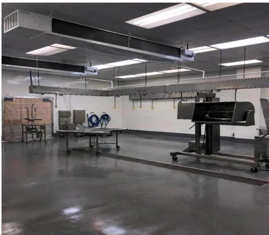
Photo 16 – View of epoxy floor at first floor salad room. No asbestos was detected in the epoxy floor materials. Photo taken December 23, 2020.
