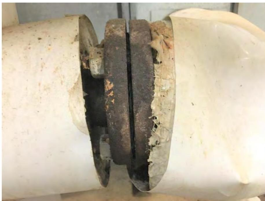
Photo 18 – View of a flange and gasket at a low pressure steam line at AC-4 in basement Mechanical Room MER B14. No asbestos was detected in accessible gaskets collected by Watts’ personnel in 2021. Photo taken May 13, 2021.
