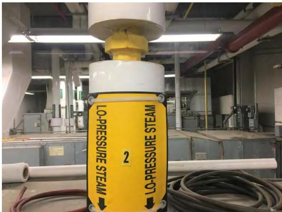
Photo 19 – View of piping in basement Mechanical Room MER 2 B-19. The majority of piping was threaded. No asbestos was detected in gasket samples collected by Watts' personnel in 2021. Photo taken May 13, 2021.
