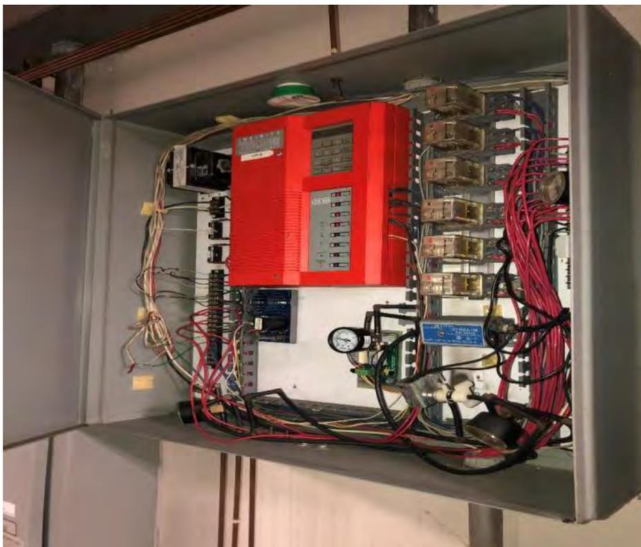
Photo 8 – View of non-suspect wire insulation and metal backer board in basement room B-19.
