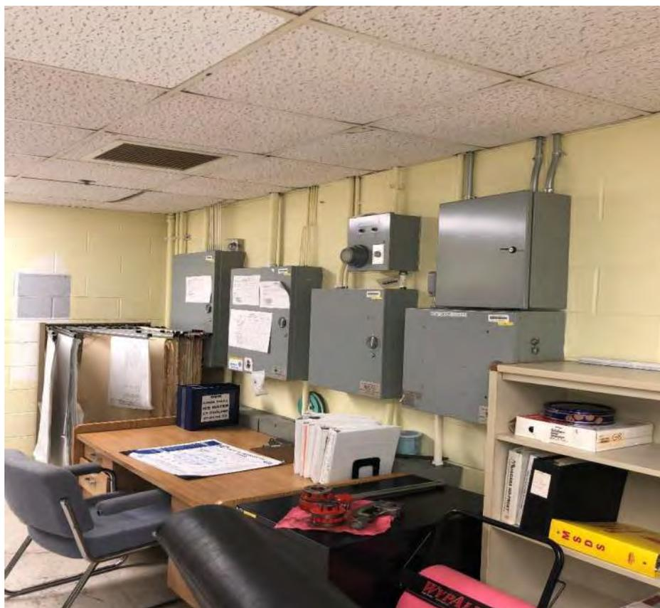
Photo 1 – View of the non-asbestos mortar for cinder block wall, 2'x 2' suspended pinhole ceiling tile and panel boards in basement room B-7. Photo taken December 23, 2020.
