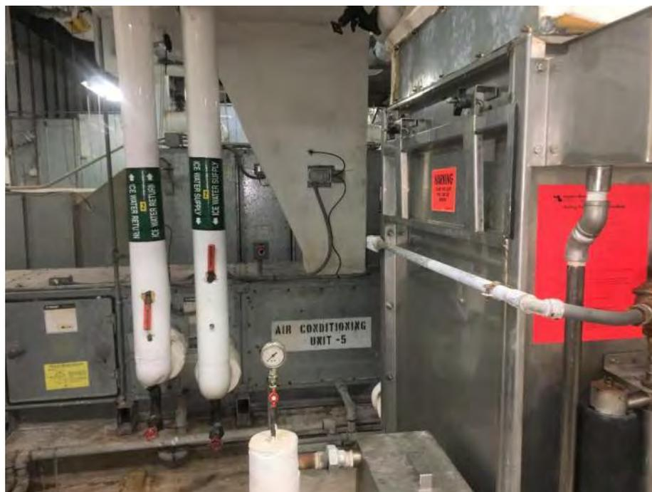
Photo 17 – View of an air conditioning unit in basement Mechanical Room MER B14. No asbestos was detected in gasket samples collected by Watts’ personnel in 2021. Photo taken May 13, 2021.
