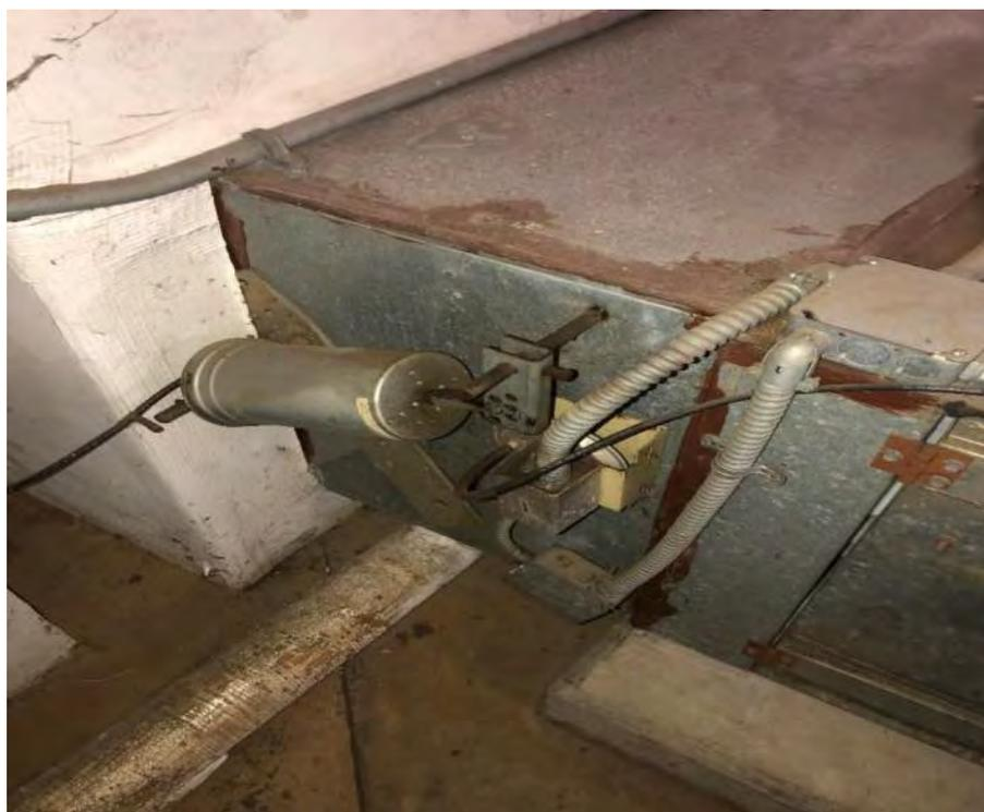
Photo 10 – View of non-suspect louver actuator in basement room B-19 and sealant on metal duct joints. No asbestos was detected in the sealant. Photo taken December 23, 2020.
