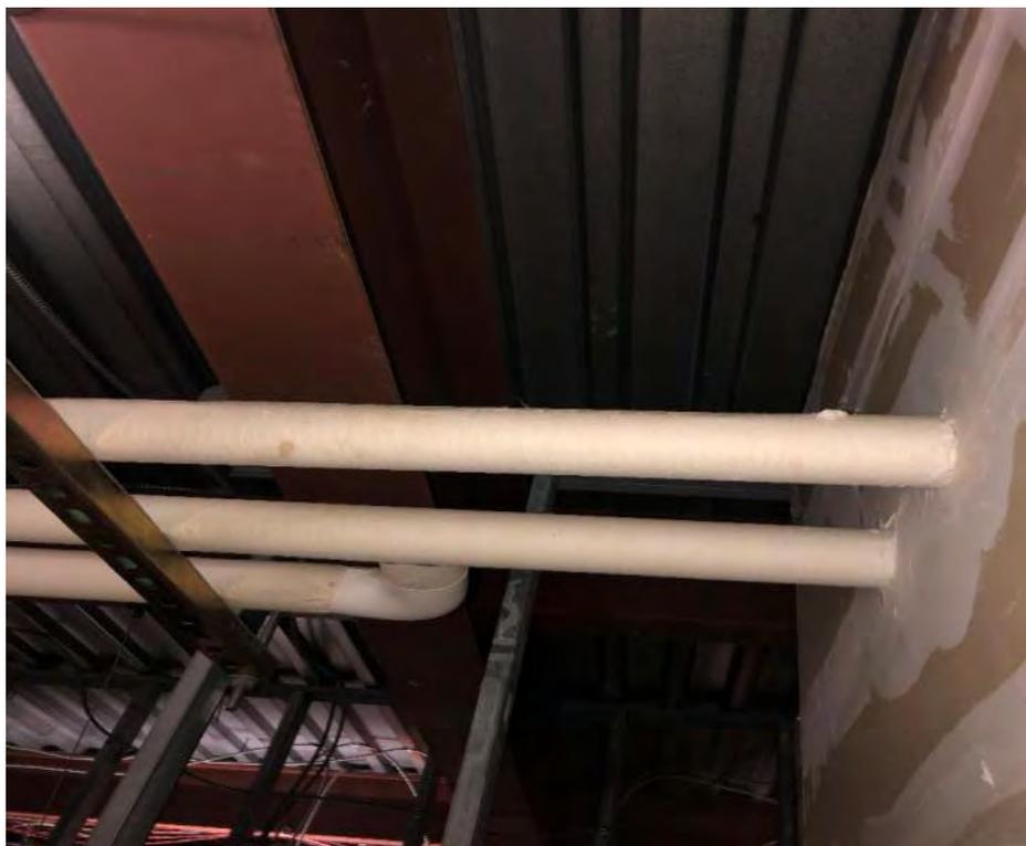
Photo 12 – View of paper tape, joint compound, wall sheetrock and paper wrap on fiberglass pipe insulation on the first floor. No asbestos was detected in these materials. Photo taken December 23, 2020.
