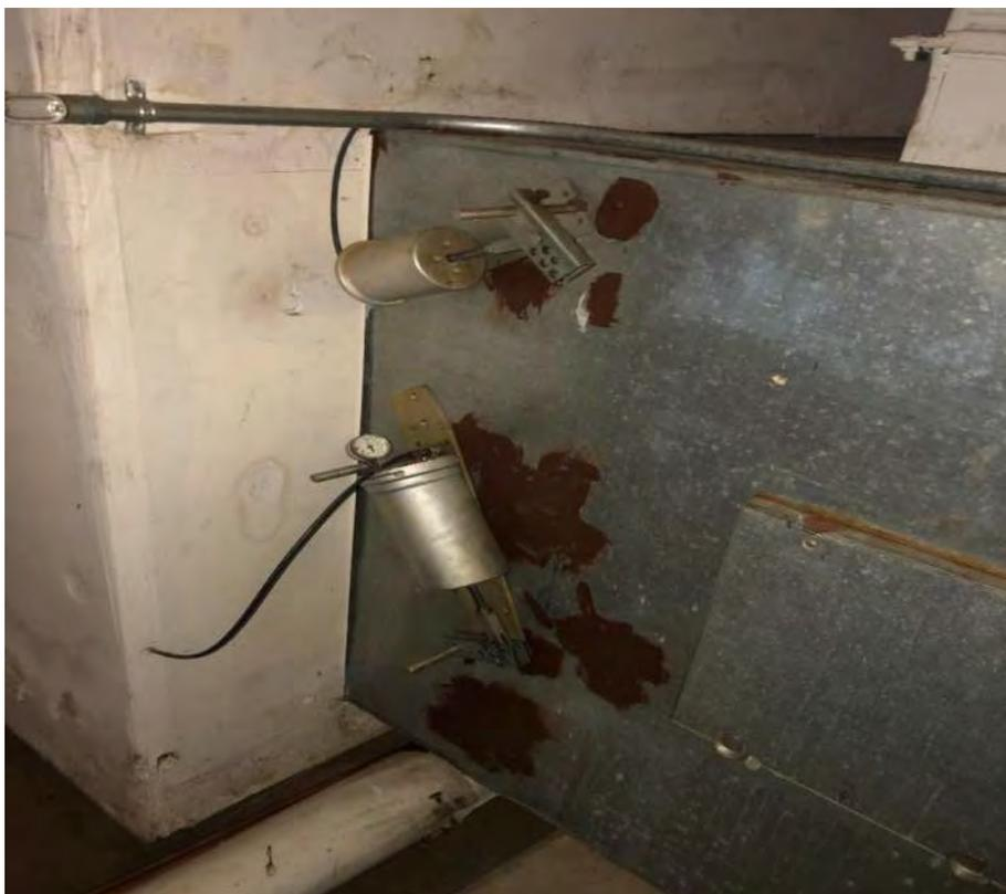
Photo 11 – View of non-suspect louver actuator in basement room B-19 and sealant on metal duct joints. No asbestos was detected in the sealant. Photo taken December 23, 2020.
