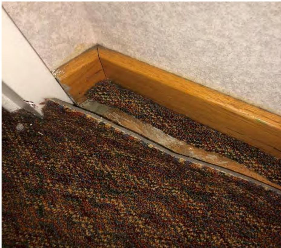
Photo 13 – View of carpet mastic and self-sticking wall paper on the first floor. No asbestos was detected in these materials. Photo taken December 23, 2020.
