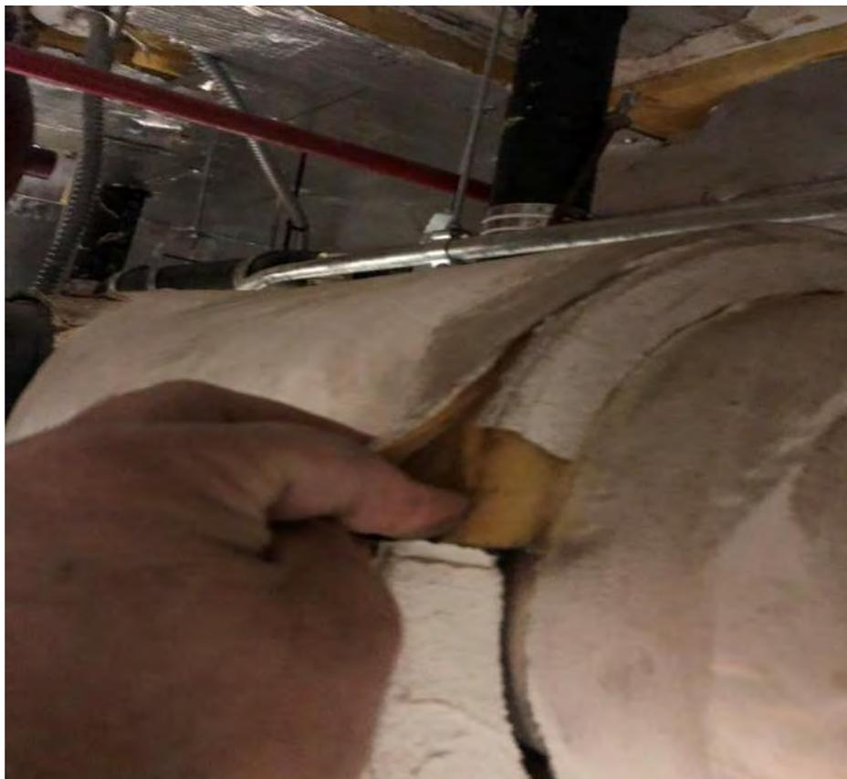
Photo 5 – View of paper wrap and sealant on end of fiberglass pipes in basement room B-5. No asbestos was detected in sealant. Photo taken December 23, 2020.
