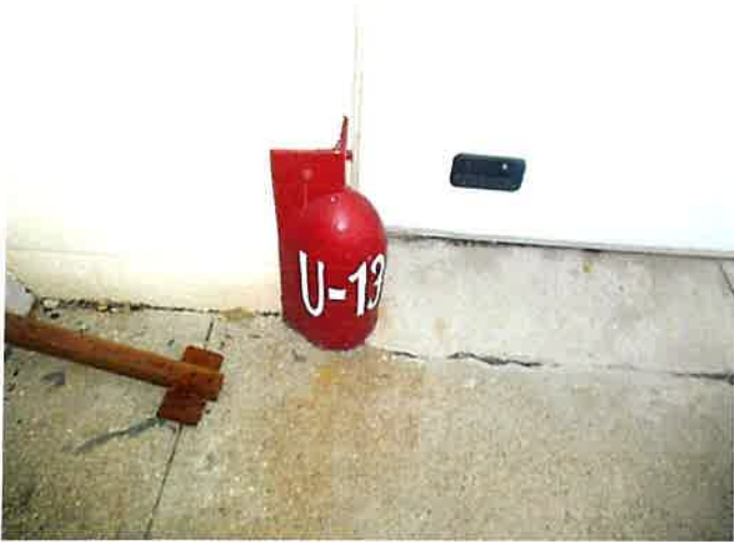
Exterior – Red Metal Corner Bumper-Lead Based Paint
