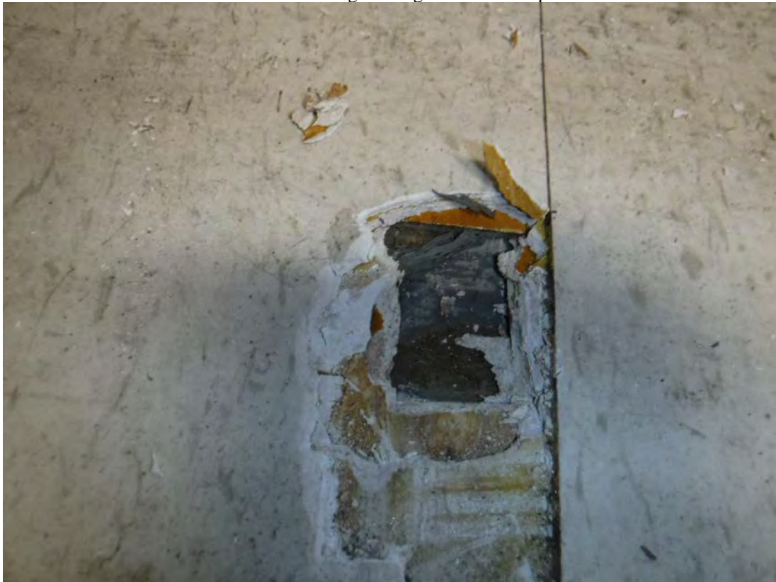
Asbestos containing flooring on 1 st floor- captains box
