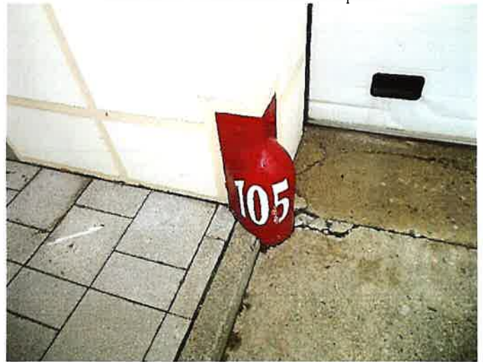
Exterior – Red Metal Corner Bumper-Lead Based Paint
