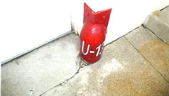
Exterior – Red Metal Corner Bumper-Lead Based Paint
