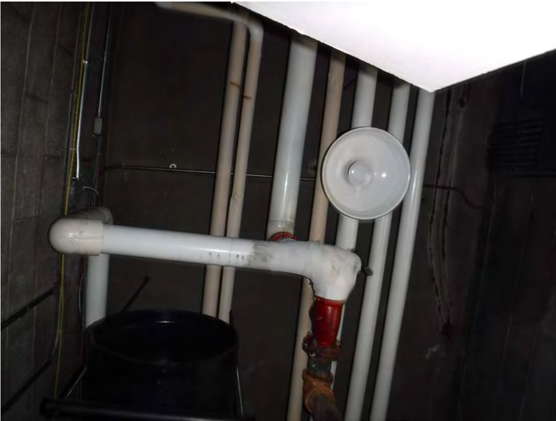
Asbestos containing pipe insulation on 1 st floor (encased with white plastic)
