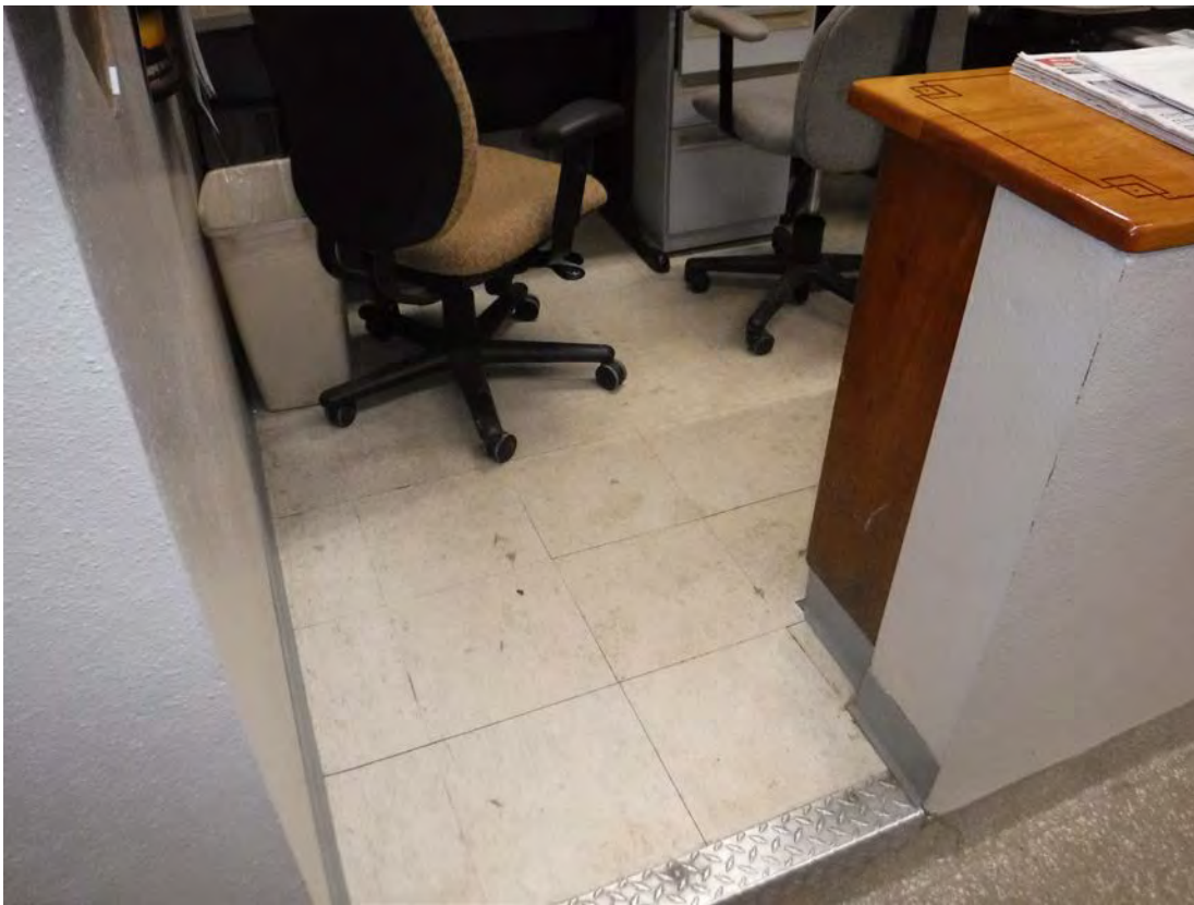
Asbestos containing flooring on 1 st floor- captains box
