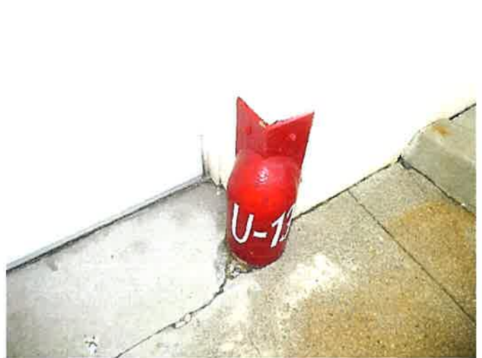
Exterior – Red Metal Corner Bumper-Lead Based Paint
