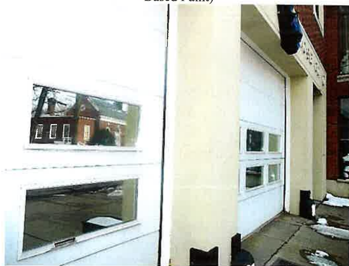
Exterior – assay # 162 - White Metal Bay Door Frame (Lead Based Paint)
