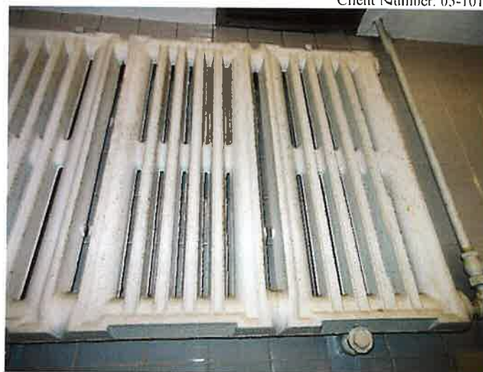
Space Identification #1005 – assay # 52 - Grey Metal Radiator (Lead Based Paint)
