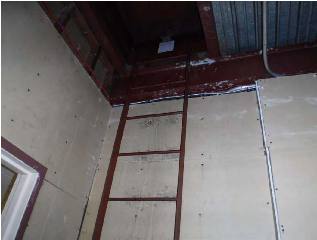
Interior, 2 nd floor- non-asbestos containing wallboard, tape, and joint compound
