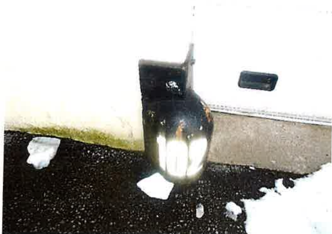
Exterior – Black Metal Corner Bumper (Lead Based Paint)
