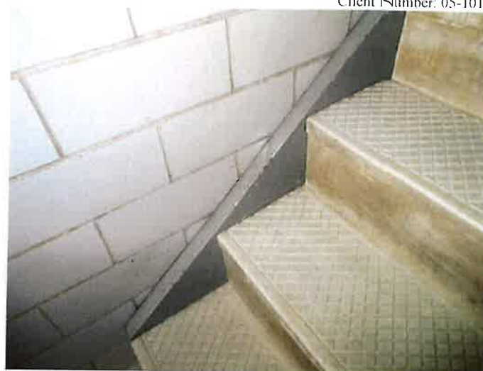
Space Identification # 1001 – assay # 7 - Staircase Stringer (Lead Based Paint)
