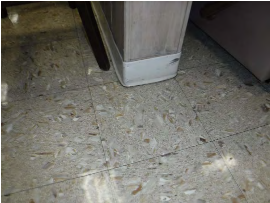
Interior, 2 nd floor- non-asbestos containing cove base and associated mastic
