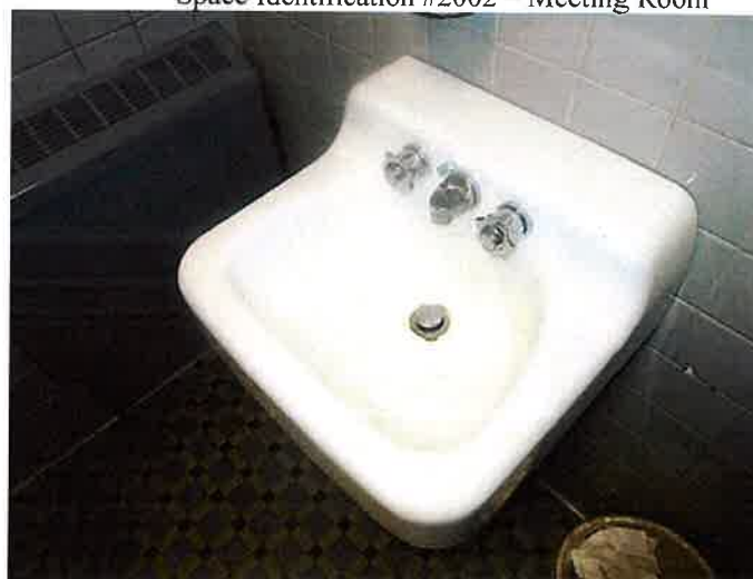
Space Identification #2003 – assay # 85 - White Sink (Lead Based Glazing)
