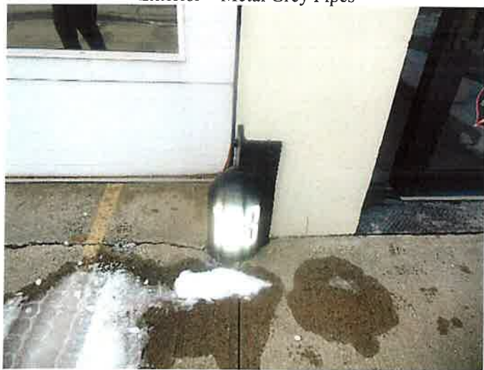
Exterior – Black Metal Corner Bumper (Lead Based Paint)
