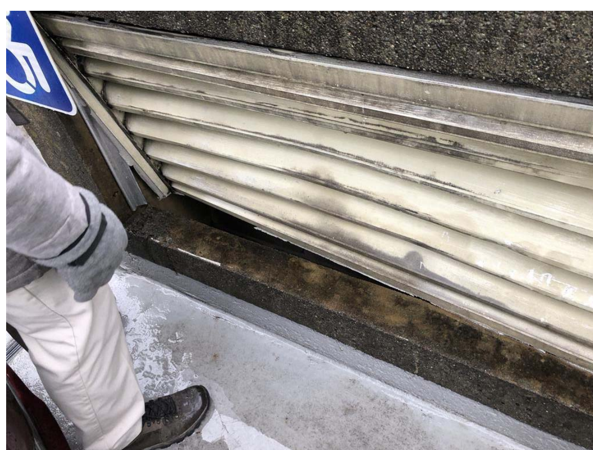
6 DAMAGE LOUVER D0.6 Not To Scale
