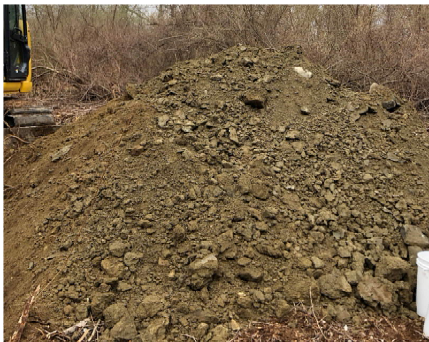
Photo 2: Excavated material from test pit LTP-5
