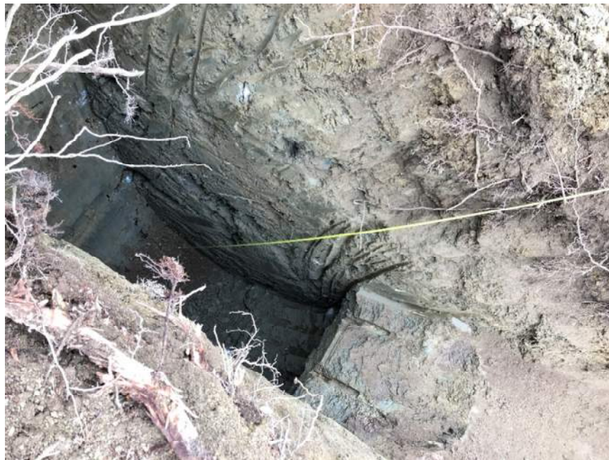
Photo 1: Profile view of test pit LTP-5
