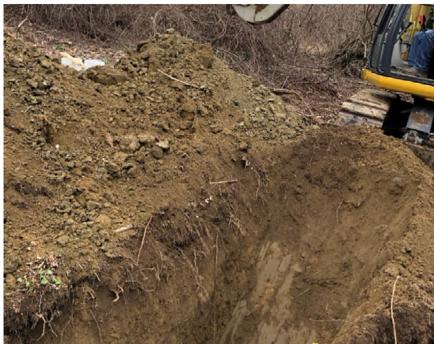
Photo 2: Excavated material from test pit LTP-2
