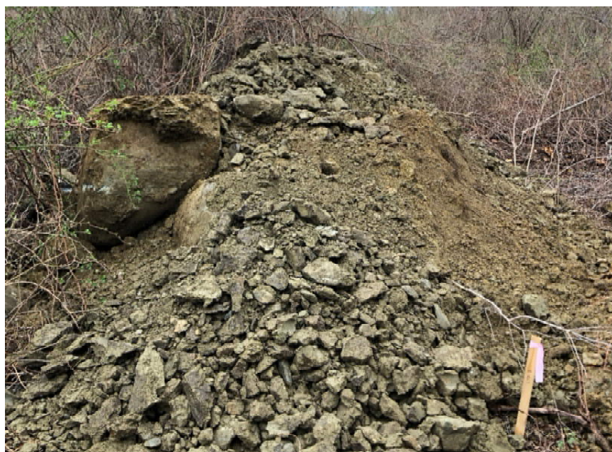
Photo 2: Excavated material from test pit LTP-6
