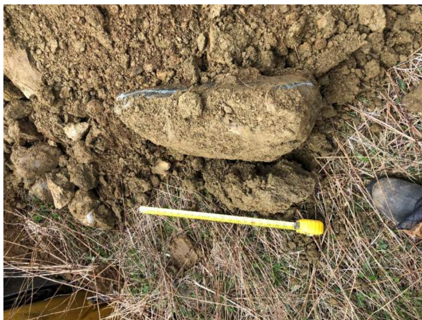
Photo 2: Excavated material from LTP-15
