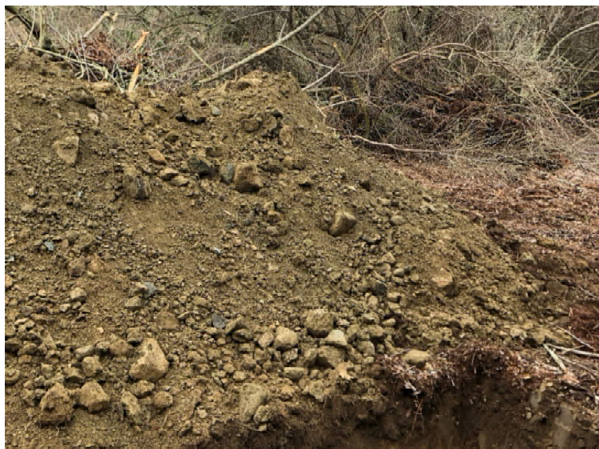
Photo 2: Excavated material from test pit LTP-7
